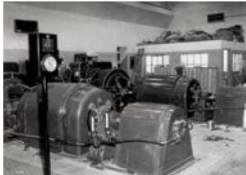
“Two 750 kw Westinghouse Turbine-Generator Sets/Ready for Trial Run.” August 30, 1942. National Park Service.
