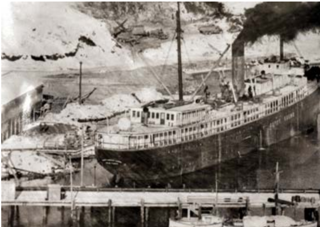
Siems Drake workers accessing beached Northwestern via gangplank. In background, center, earth-movers excavate the footprint of the Naval Air Station Powerhouse. Museum of the Aleutians.
