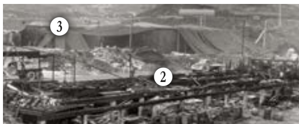
Warehouse remains #2, and intact wooden fuel storage tanks #3. Museum of the Aleutians.
