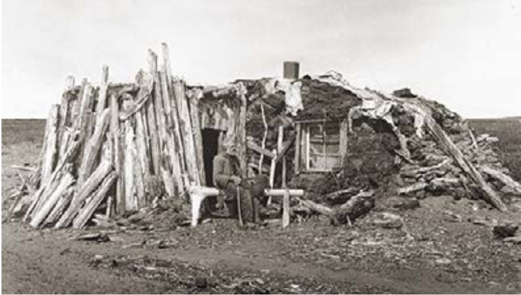
Miner's cabin built of logs and sod, Nome Beach. Alfred G. Simmer Collection, Alaska State Library, ASL-P137-038.
