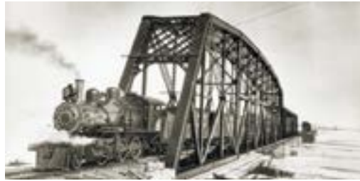
Of the hundred and twenty-nine bridges built on the CRNW line, the "Million Dollar Bridge," (or Miles Glacier Bridge [above]) was the most costly, with a price tag of 1.4 million. (Damaged by the 1964 earthquake and repaired in 2004-5 at a cost of 19 million, the bridge could arguably be called the "20 Million Plus Dollar Bridge.") The CRNW Railroad was listed on the National Register of Historic Places in 1973; the Million Dollar Bridge was added to the register in 2000. National Park Service.
