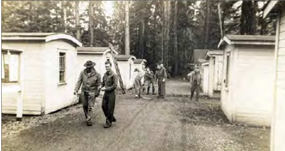
Figure 210. Soldiers with the U.S. Army Air Corps Marine Rescue Squadron clown behind their officer's back upon completion of semaphore training at the Ward Lake CCC camp in June, 1942. The gable-roofed recreation hall can be seen at the end of the right row in this view north.
