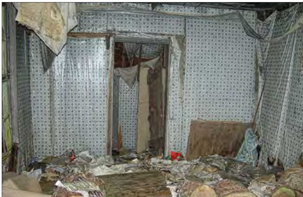
Figure 89. The interior of Building B is littered with documents predating World War II.
