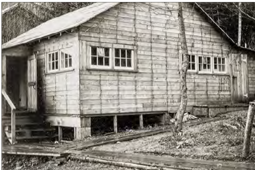
Figure 62. Building T south of the mill was mapped as a laundry, toilet, and shower facility in 1942, and was later incorporated into the home of Sam Pekovich. Both plank doors visible here remained in place in 2008.
