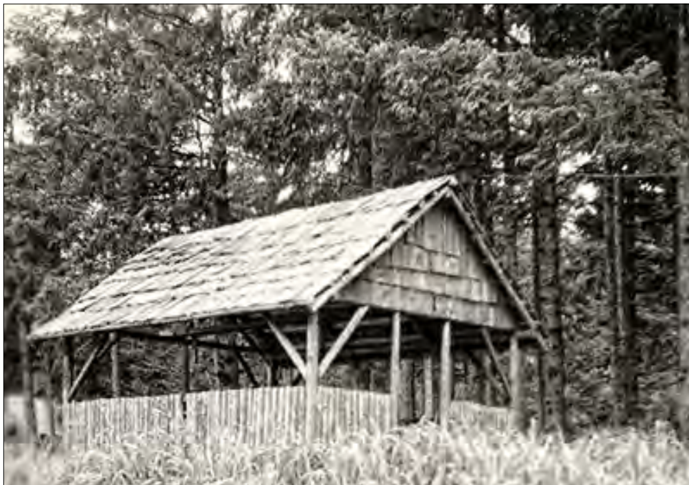
Figure 161. A fish-cleaning station of spruce poles and cedar shakes in the Adirondack style was built near the beach.
