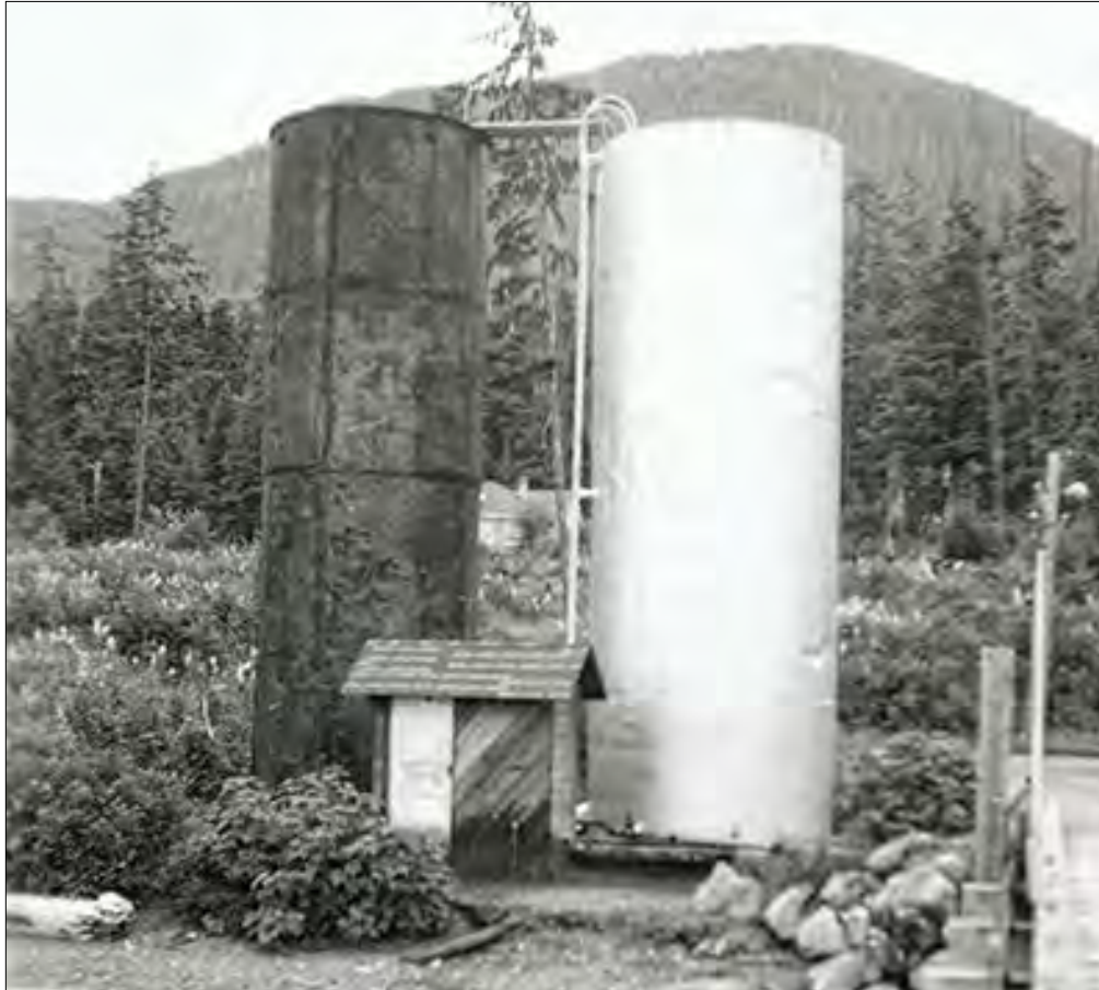
Figure 160. Two 20,000 gallon steel tanks (viewed here in 1944) behind the clinic held the campus's heating oil.
