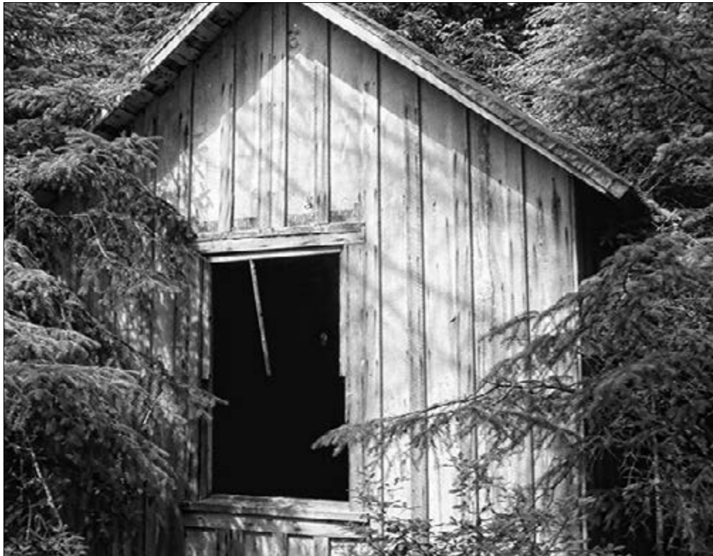
Figure 36. Centrally located on the cannery site is a small frame board-and-batten cabin from the cannery era.
