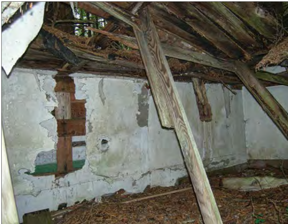
Figure 41. The interior walls of the most intact Aleut cabin are covered with beaverboard painted white.
