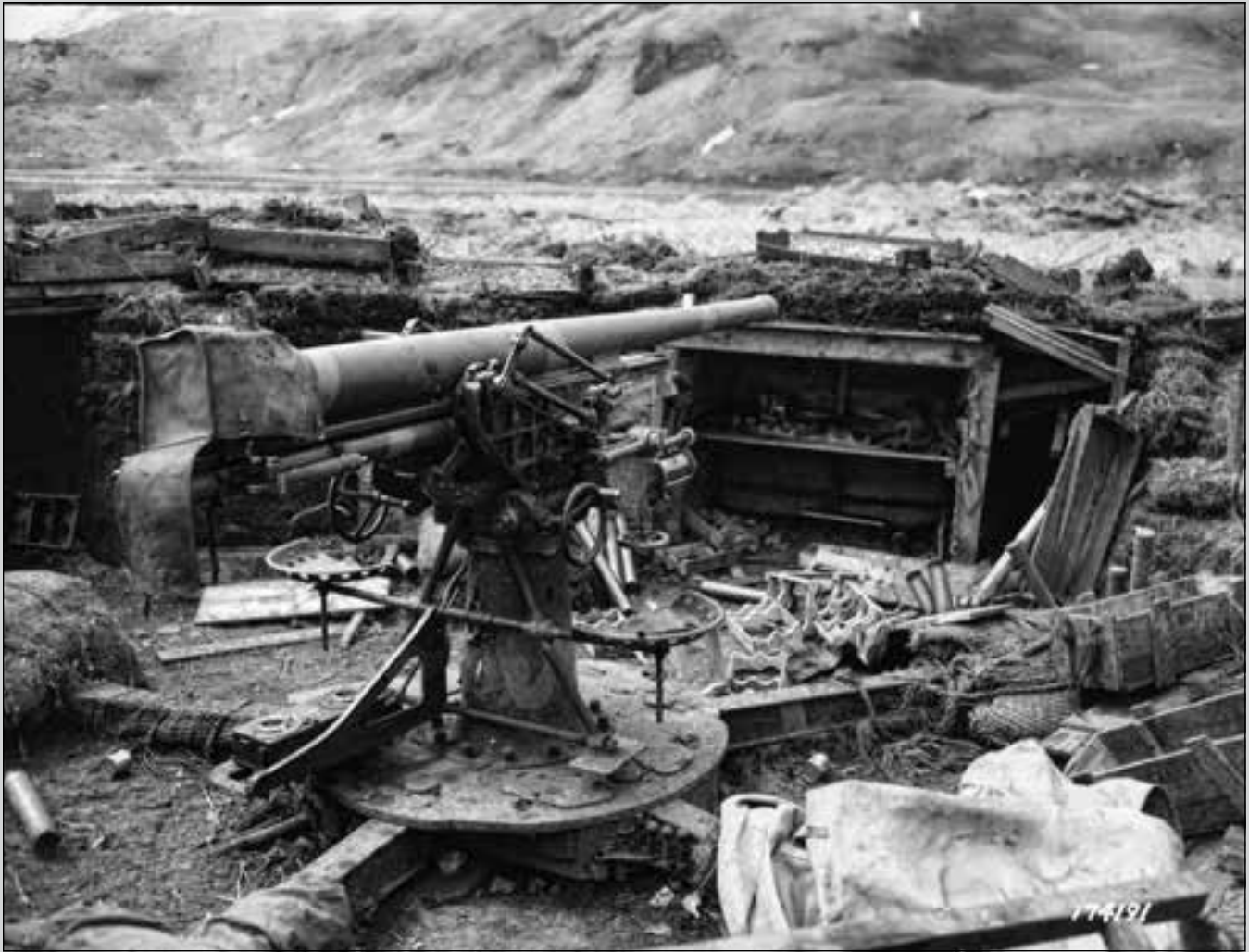
Above: Photo IV-14: The Japanese employed the Type 88 75-millimeter dual-purpose gun extensively as an anti-aircraft and direct fire gun. The Type 88 provided the Japanese with their main artillery defense capability on Attu. This one was captured in the West Arm of Holtz Bay. It was dug in and protected by a berm to withstand anything but a direct hit. Unlike Kiska, where whole batteries of the 75-millimeter guns remain, only one gun can be found today in the East Arm. (U.S. Army Signal Corps, NARA 2, RG111-156-174190)
