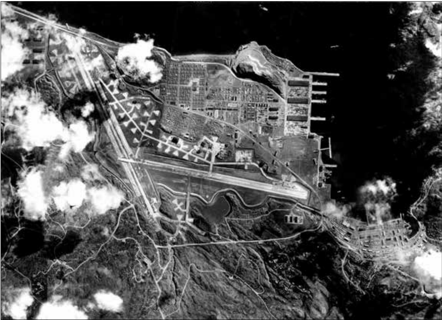
Photo III-11: Following the end of the war, the Army transferred Adak to the Navy who turned it into an anti-submarine warfare base. With the end of the Cold War, the Navy closed Adak Air Facility in 1997. (Rhodes Arnold Collection, UAF 1994-0197-00117)
