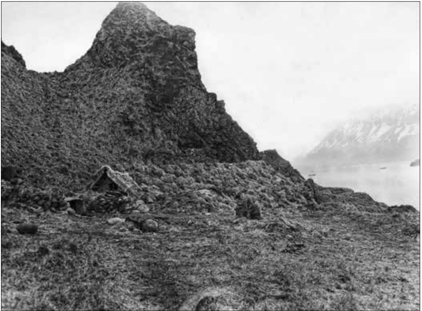
Photo IV-12: The Japanese took great pains to camouflage their positions including their barracks and supply buildings. This building was found on the side of a hill on the West Arm of Holtz Bay. (U.S. Army Signal Corps, NARA 2, RG111-169-177679)
