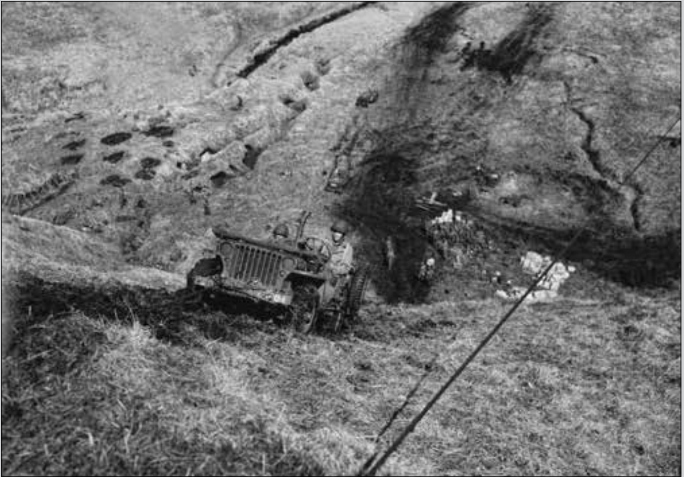
Photo V-15: Engineers overcame the steep escarpment by establishing a cableway. The tableland between the escarpment and Hill X permitted the use of jeeps to move men, equipment and supplies. (U.S. Army Signal Corps, NARA 2, RG111-156-174155)
