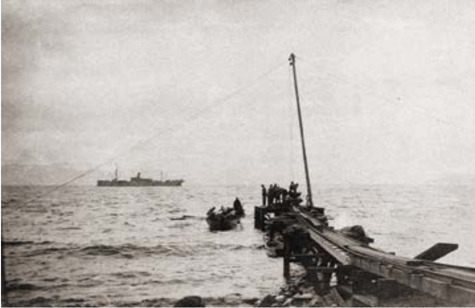
The wharf on Unalga, with the USS Nero, 1912. This wharf replaced the first that was destroyed in a storm. U.S. Naval Historical Center. Photo #: NH 105434.
