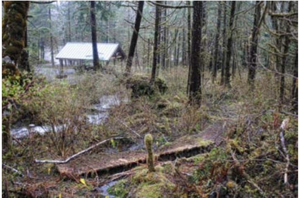
Boardwalk at Ward Lake, May 4, 2011. Photograph by Charles Mobley.
