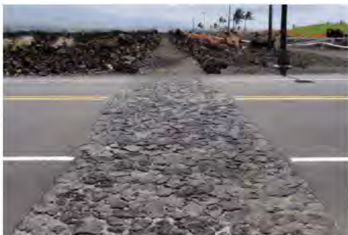
This is the preferred surface treatment. It mimics the authentic, historic surface while enabling road use.
