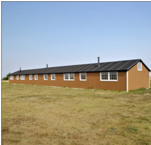
The reconstructed barrack at Amache. NPS photo.
