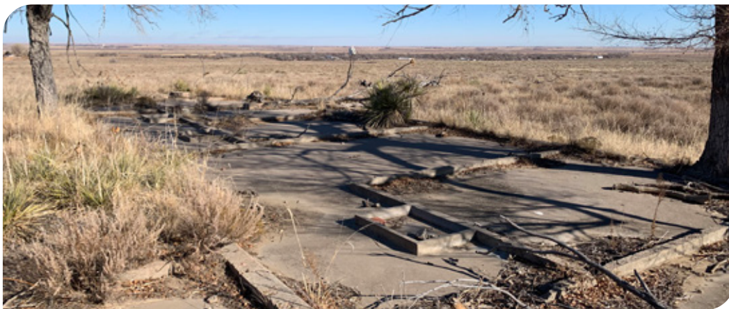
Visible foundations of the bathroom in Block L-9. The historic integrity of the site was commonly referenced by commenters. NPS photo.
