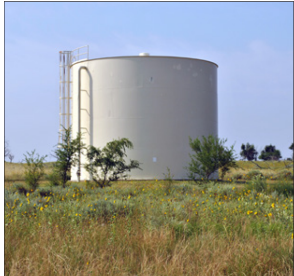
A 219,000-gallon water storage tank, part of the Town of Granada's water infrastructure, is located at the Amache site. NPS photo.
