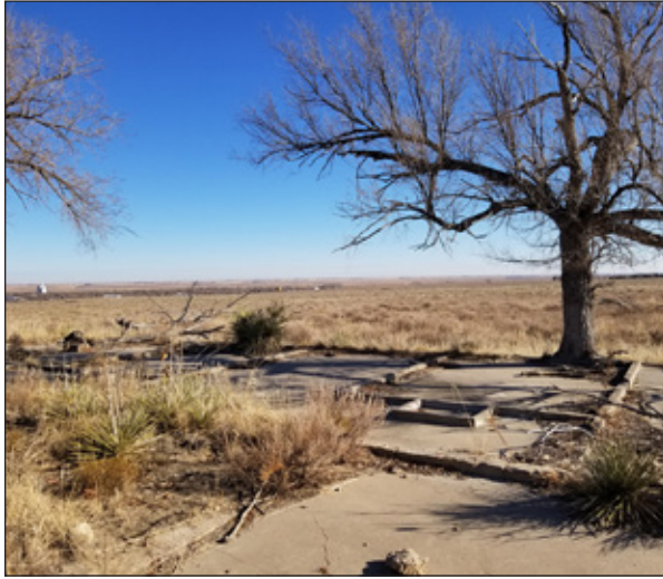
Intact building foundations can be found throughout the Amache site's cultural landscape. NPS photo.
