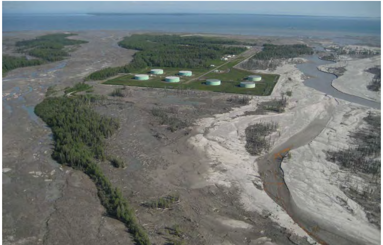
Figure 7. Aerial view of the lower Drift River and the Drift River Oil Terminal after 2009 eruptive activity on Redoubt Volcano. April 4th lahar deposits (lighter color on right) overlie older darker lahar deposits from earlier event(s) in March. Image taken by Max Kaufman on June 8, 2009 and courtesy of the AVO/UAF-GI, AVO image ID 19402
