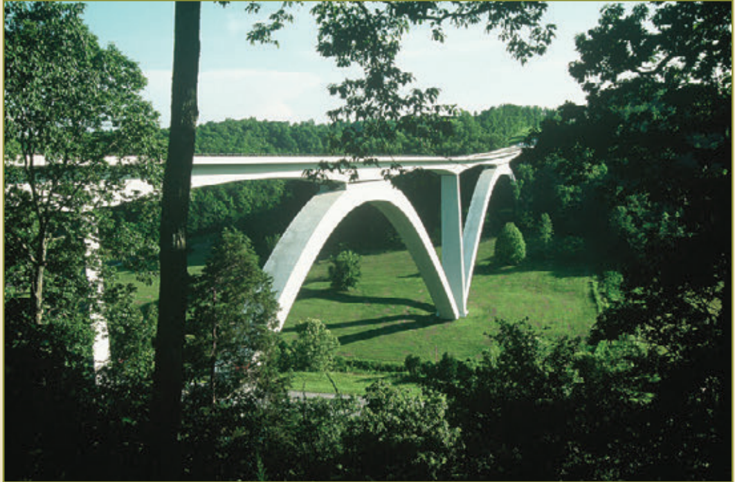
The Denver Service Center completed a project in 1994 to construct the first precast segmental double arch bridge in the United States located over Route 96 in Tennessee as part of Natchez Trace National Parkway.
