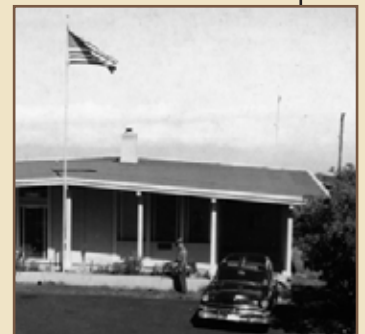
The visitor center at Haleakalā National Park is a great example of Mission 66 design and construction.
