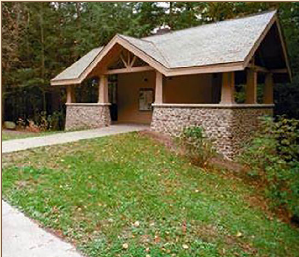
The cost of constructing a restroom near Raymondskill Falls in Delaware Water Gap National Recreation Area received widespread national media attention.
