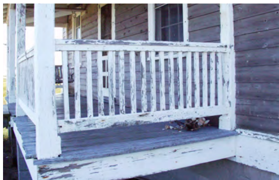
Figure 15 View of southwest end of front porch. (NPS-SERO-CR, 2002)
