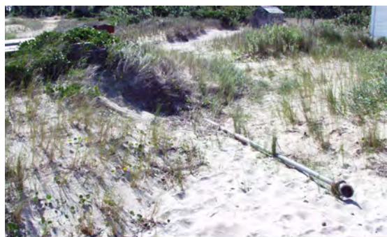
Figure 38 Waste line from kitchen at original site. (NPS-SERO-CR, 2002)
