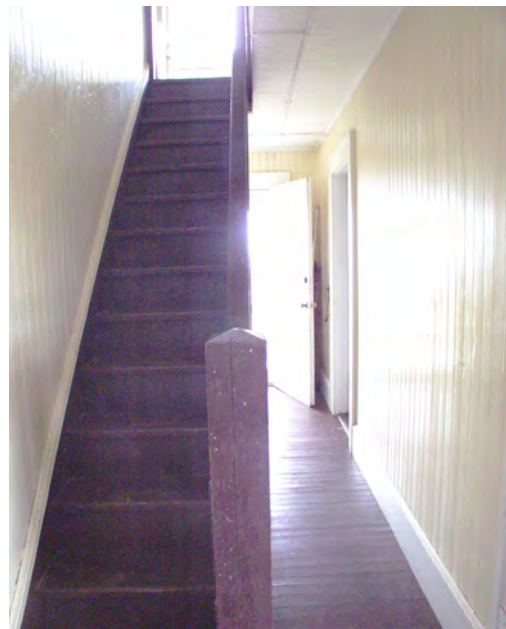
Figure 18 View to northwest in hall. (NPS-SERO-CR, 2002)
