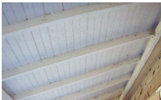
Figure 16 View east of front porch ceiling. (NPS-SERO-CR, 2002)
