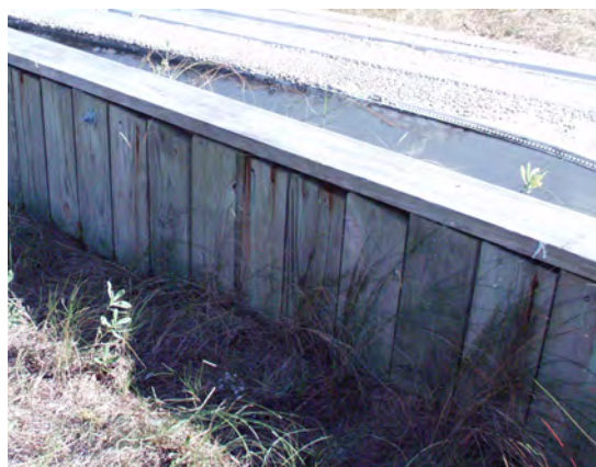
Figure 2 View of flood wall surrounding house. (NPS-SERO-CR, 2002)
