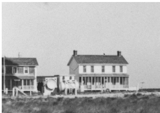
Figure 11 Partial view of Keeper's Dwelling (at left) around 1940, after being resided with cedar shingles. The structures between the two buildings have not been identified. (CALO Coll. D-01)
