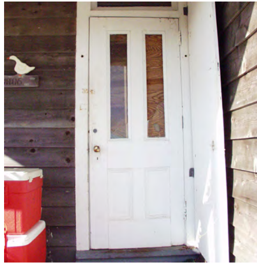
Figure 8 View of back door. Original front door was of a similar design. (NPS-SERO-CR, 2002)
