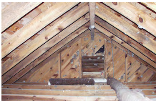
Figure 7 View southeast in attic. (NPS-SERO-CR, 2002)
