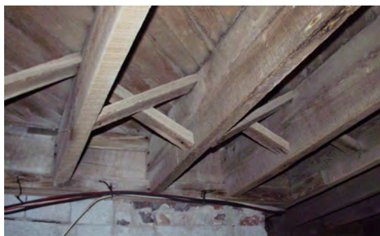
Figure 6 View of typical floor framing. (NPS-SERO-CR, 2002)
