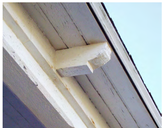
Figure 13 View of front porch eave bracket. (NPS-SERO-CR, 2002)
