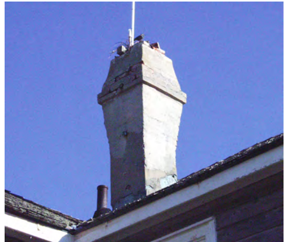
Figure 4 View of chimney. (NPS-SERO-CR, 2002)
