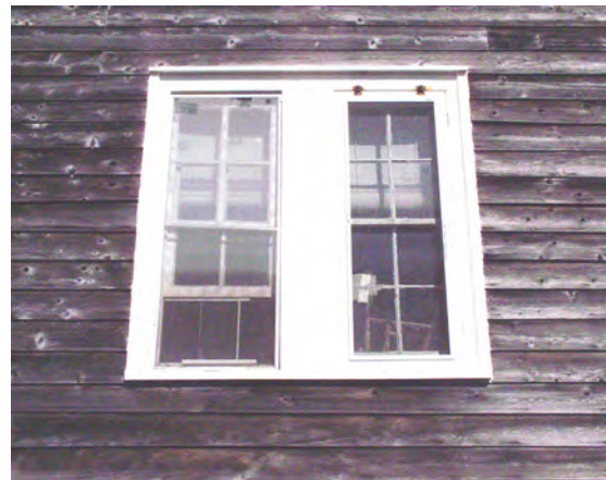
Figure 9 View of typical double windows. (NPS-SERO-CR, 2002)
