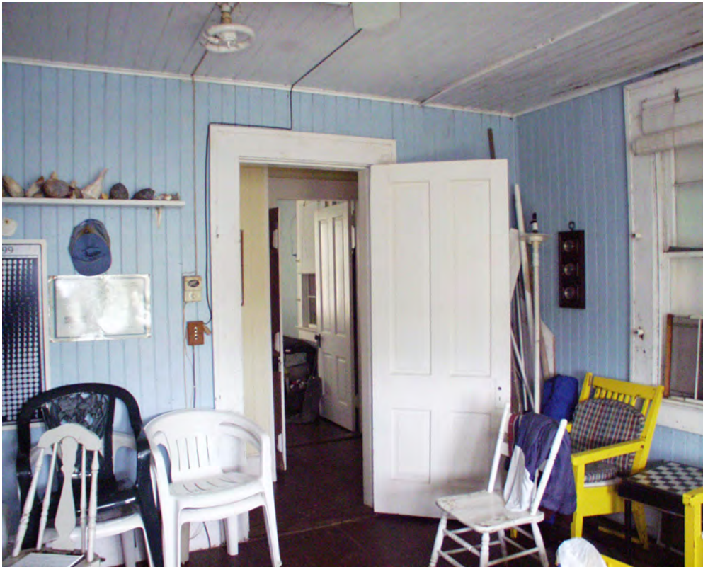
Figure 23 View to west in Room 102. (NPS-SERO-CR, 2002)
