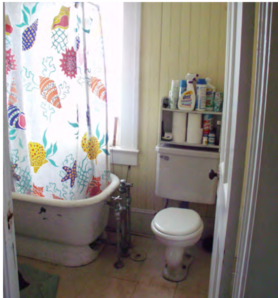
Figure 36 View to south of bathroom installed in 1930s. (NPS-SERO-CR, 2002)
