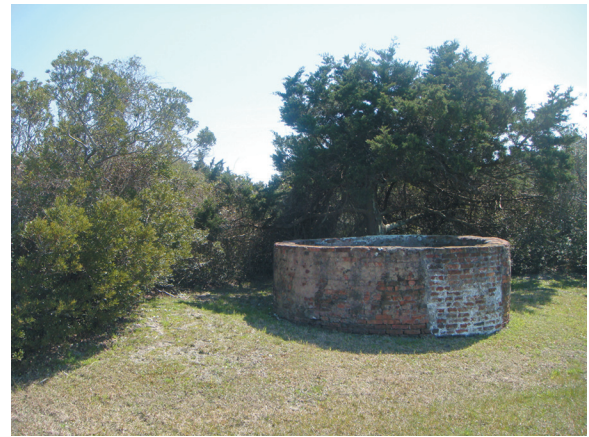
Figure 6-1. Brick cistern, Marine Hospital, Portsmouth, 2008. Photo by David E. Whisnant.
