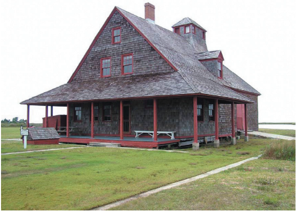
Figure 6-21. Portsmouth Life-Saving Station after renovation, 2006. Cape Lookout National Seashore archive.
