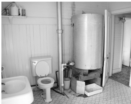
Figure 80 View to west in Room 203. (NPS-SERO-CRS, 2002)
