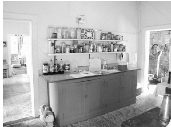
Figure 68 View of north wall of kitchen. (NPS-SERO-CR, 2002)
