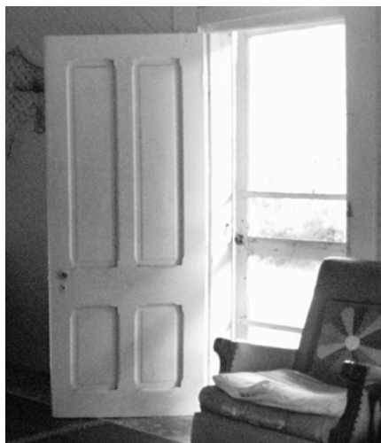
Figure 51 Four-panel door at northern end of building, typical of original doors, c. 1887. (NPS-SERO-CRS, 2002)
