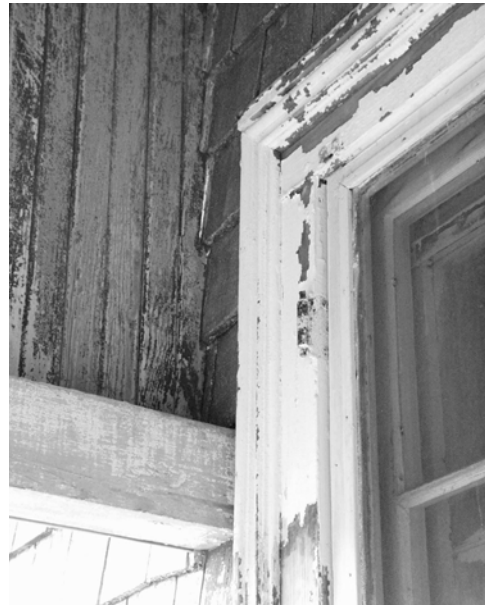
Figure 56 Typical second-floor window casing with added backband. (NPS-SERO-CRS, 2002)
