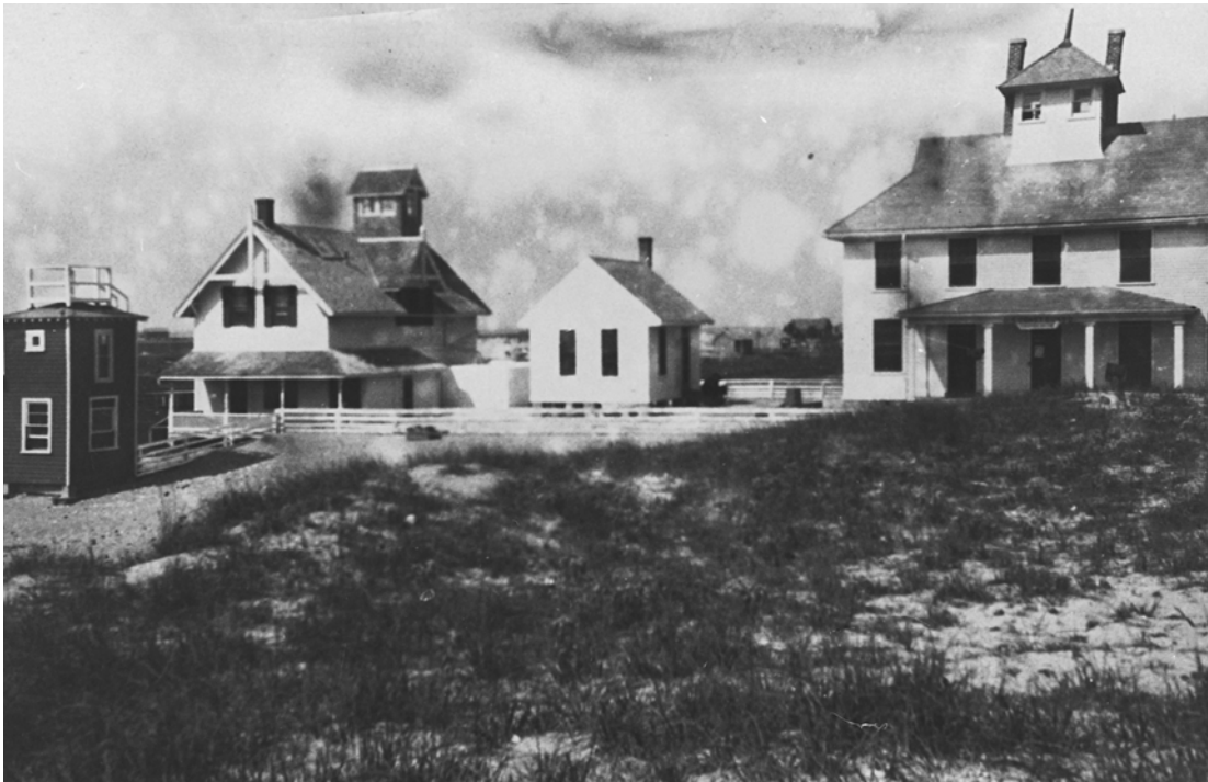
Figure 31 View north of Cape Lookout Coast Guard Station, 1920. The new compass station, or “radio shack,” is at left, and the new concrete cistern is visible between the kitchen at center and the old life-saving station. (CALO Coll. D-52)
