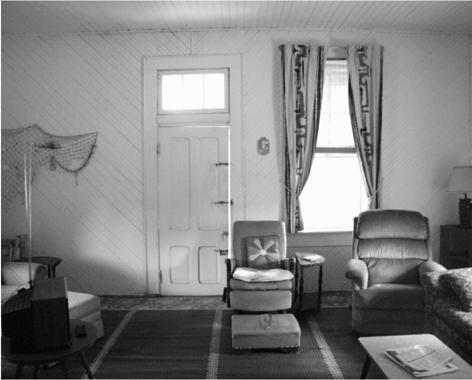
Figure 74 View north in Room 104. Two pairs of large doors originally opened into the boat room at this location. (NPS-SERO-CRS, 2002)
