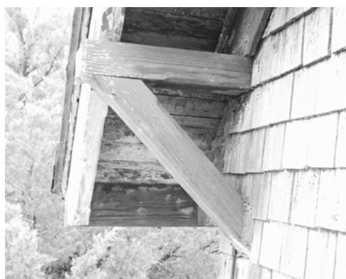
Figure 55 View of typical gable eave bracket. (NPS-SERO-CRS, 2002)
