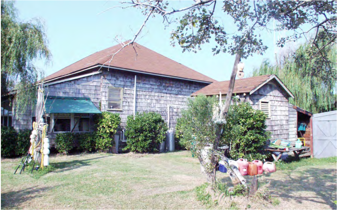
Figure 24 View west of L. S. S. Boat House. (NPS-SERO-CR, 2003)
