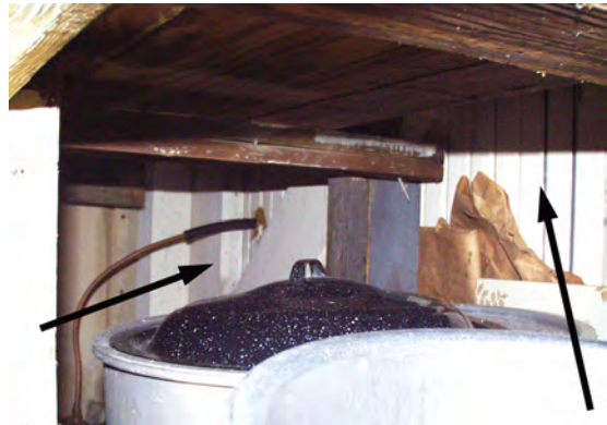
Figure 33 View of part of original boat doors under kitchen counter. Arrows indicate chamfered framing of door, left, and V-joint paneling used to finish doors, right. (NPS-SERO-CR, 2002)
