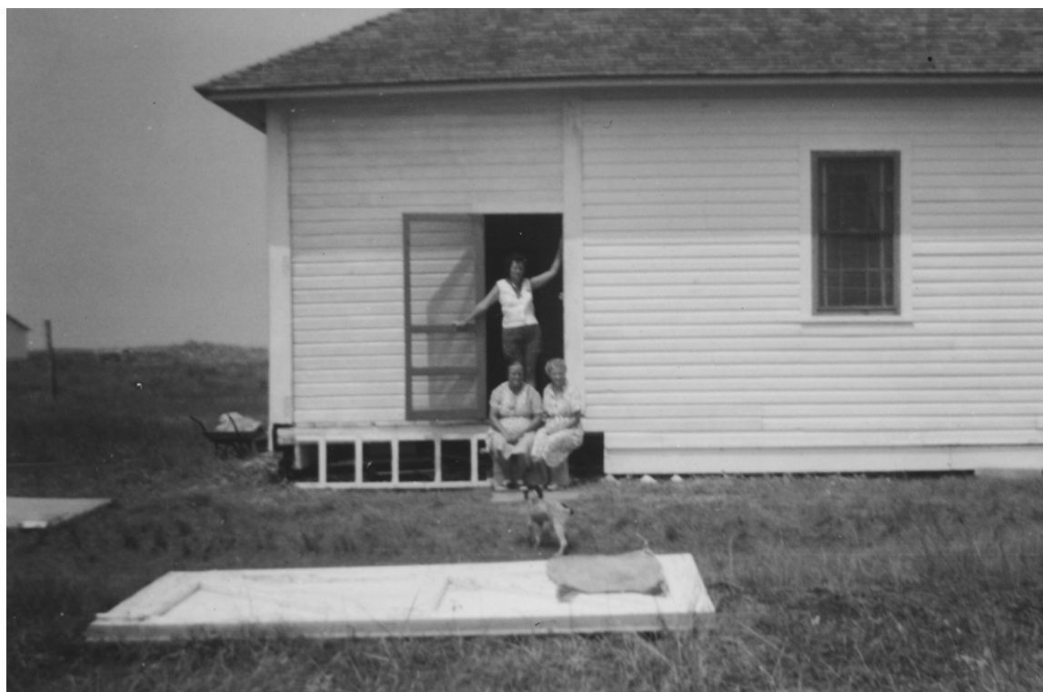
Figure 15 View of new Boat House after its relocation in 1958. (CALO Coll.)
