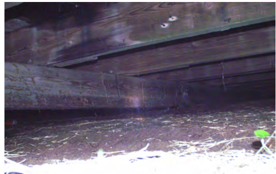
Figure 25 View of floor framing near rear of house. (NPS-SERO-CR, 2003)
