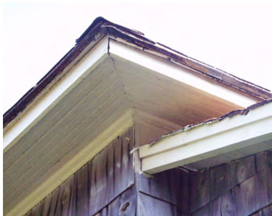
Figure 26 View of south corner and typical eave detail. (NPS-SERO-CR, 2002)
