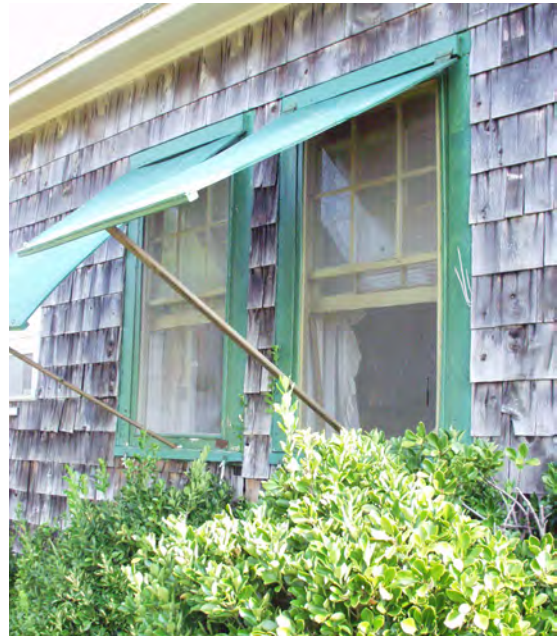
Figure 28 View of historic windows on northwest side of house with modern awning shutters. (NPS-SERO-CR, 2002)
