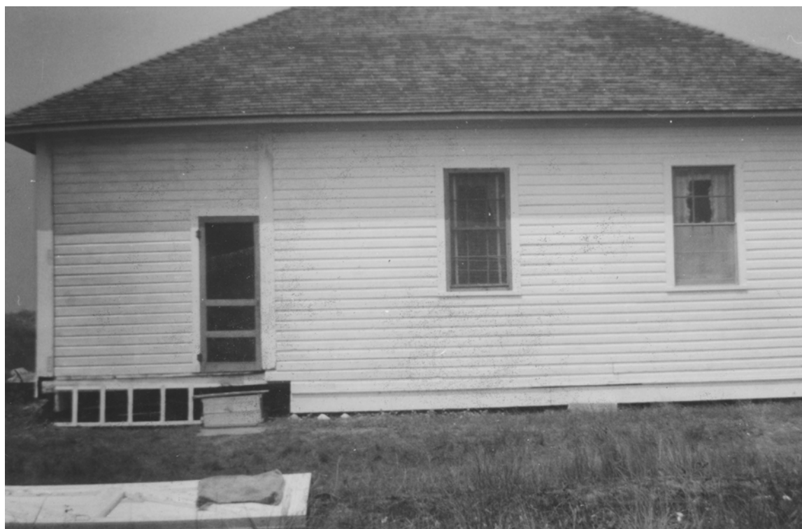
Figure 21 View of Boat House in 1961 after its conversion into a residence. One of the original doors is visible in the foreground.
