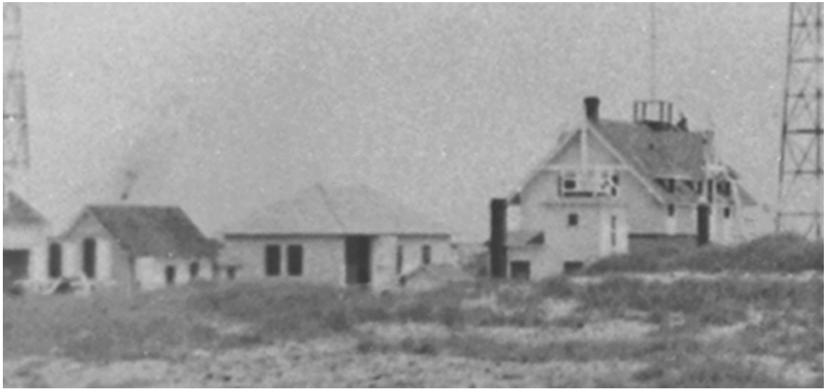
Figure 20 View north of Coast Guard Station, c. 1941, with Boat House at center. (CALO Coll.)
