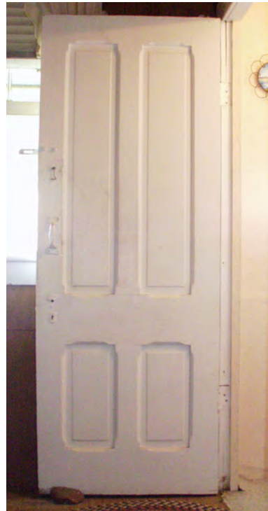
Figure 36 View of door to Room 102, believed salvaged from Life- Saving Station when it was remodeled in 1924. (NPS-SERO-CR, 2002)
