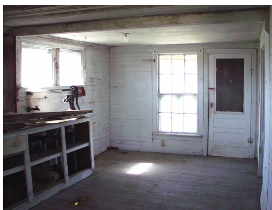
Figure 21 View west showing what was Room 103, now combined with Room 104. (NPS-SERO-CRS, 2002)
