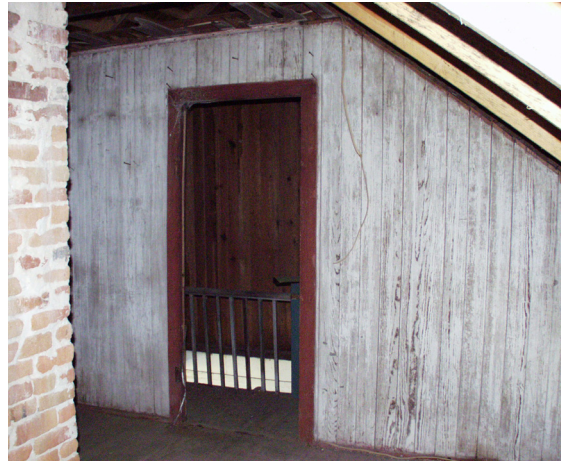
Figure 27 View south in Room 202. (NPS-SERO-CRS, 2002)
