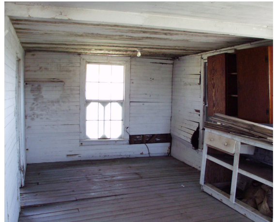
Figure 22 View east showing Room 104, now combined with Room 103. (NPS-SERO-CRS, 2002)
