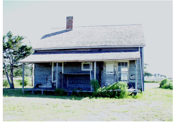
Figure 10 View of rear or southwest side of Dixon House. (NPS-SERO-CRS, 2002)
