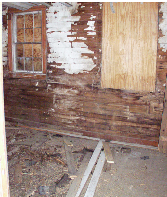
Figure 24 View south in Room 201. (NPS-SERO-CRS, 2001)
