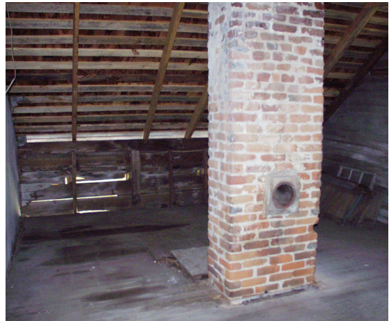
Figure 26 View west in Room 202. (NPS-SERO-CRS, 2002)
