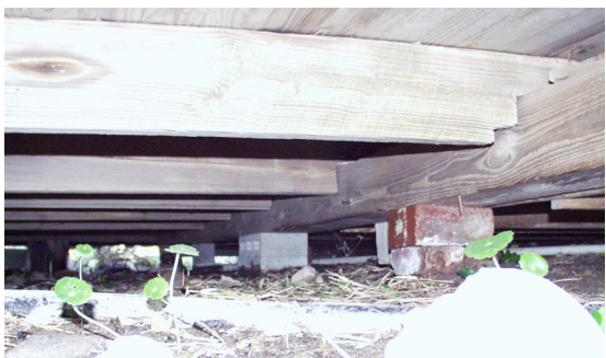
Figure 20 View west under Room 101. (NPS-SERO-CR, 2003)
