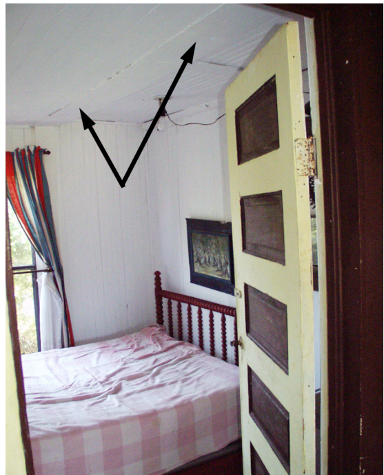
Figure 32 View east in Room 102, with arrows indicating line of wall that was relocated to create this room. (NPS-SERO-CR, 2003)
