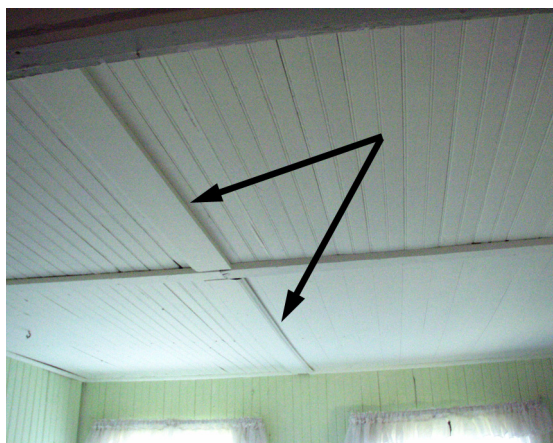
Figure 30 View of ceiling in Room 101, with arrows indicating location of wall that originally divided the space. (NPS-SERO-CR, 2003)
