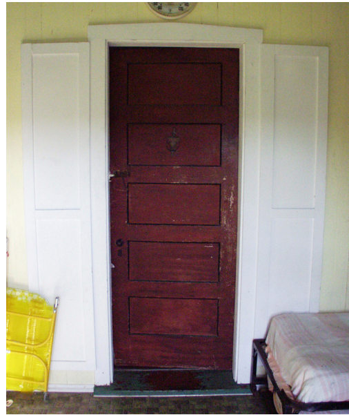
Figure 22 View of front door. Shutters and possibly the shaped header are modern additions. (NPS-SERO-CR, 2003)
