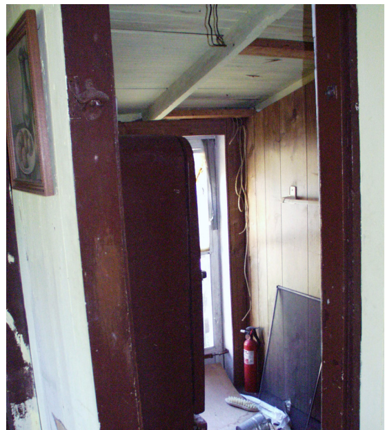
Figure 40 View to north of Room 105. (NPS-SERO-CR, 2003)
