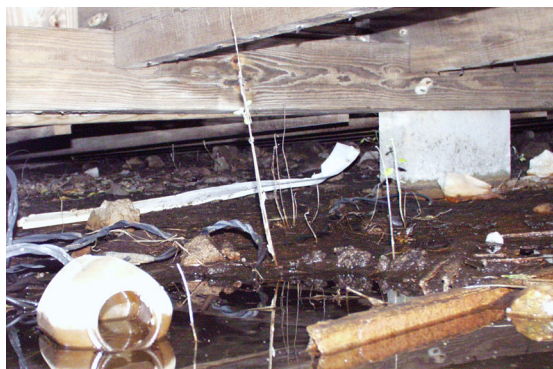
Figure 19 View south under Room 101, showing front sill of house. (NPS-SERO-CR, 2003)
