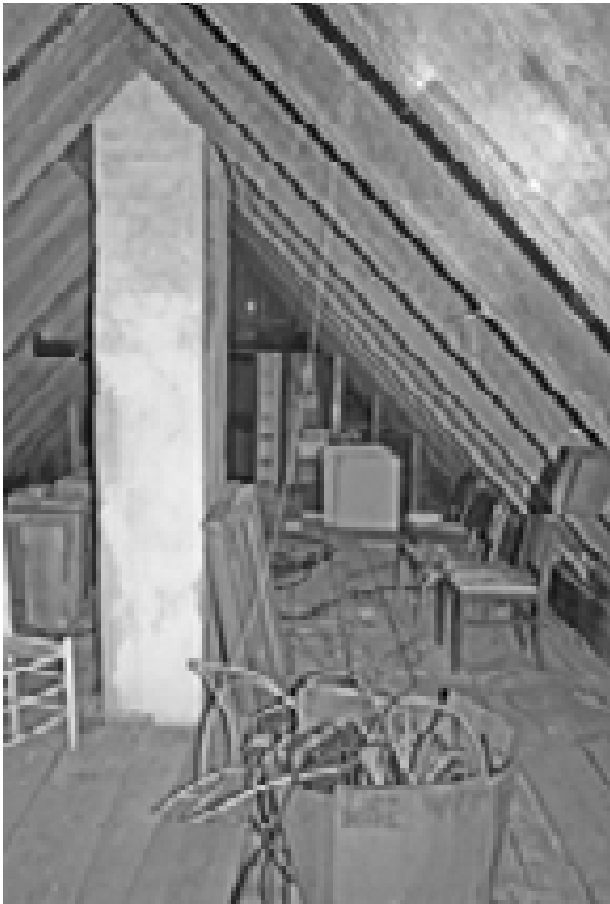
FIGURE 144. View northeast in attic. (T. Jones, NPS, 2005)
