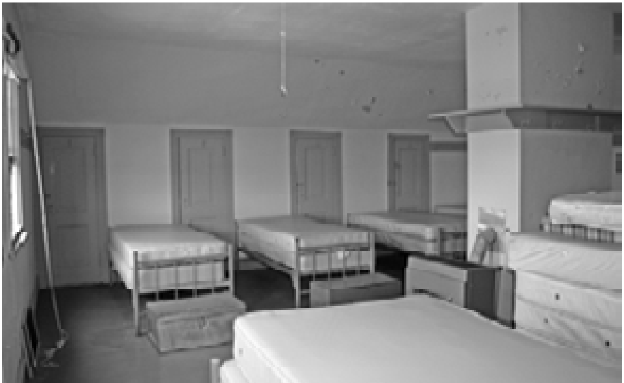
FIGURE 132. View north in Room 201. (T. Jones, NPS, 2005)
