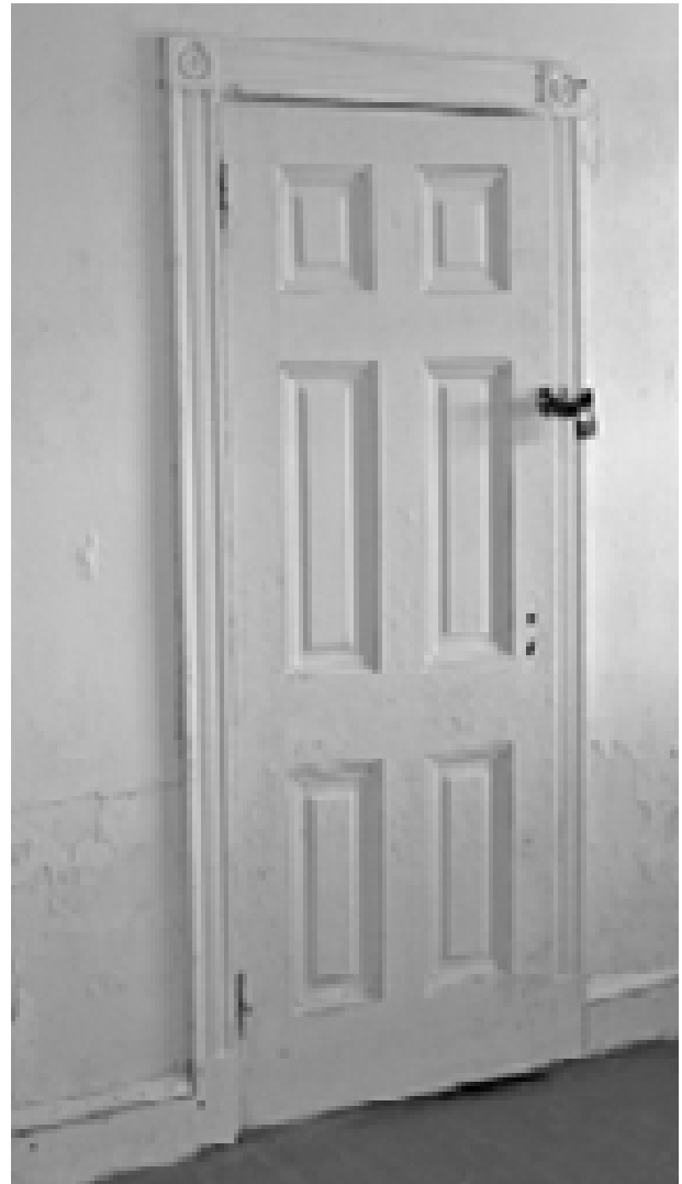
FIGURE 91. Typical six-panel door and casing. (T. Jones, NPS, 2005)
