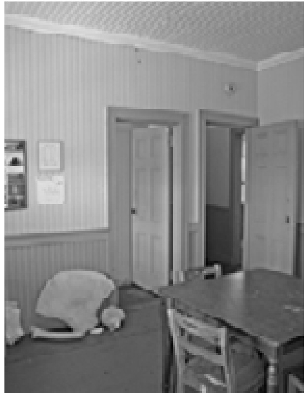
FIGURE 100. View north in Room 102. (T. Jones, NPS, 2005)
