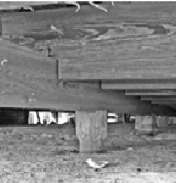
FIGURE 63. View west under boat room. (T. Jones, NPS, 2005)
