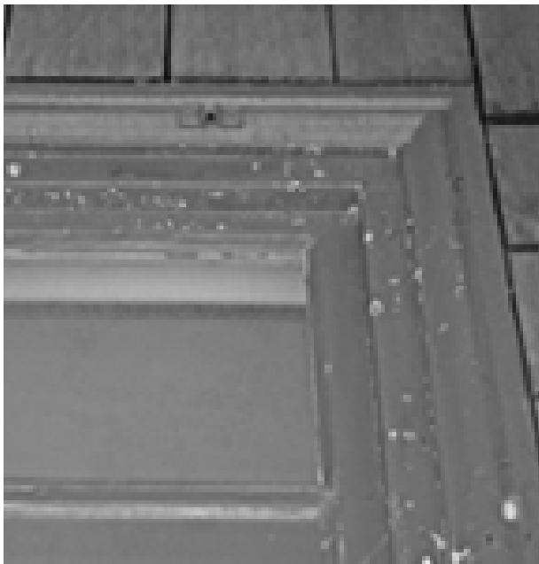
FIGURE 75. View of typical window casing. (T. Jones, NPS, 2005)
