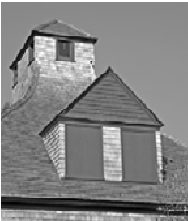
FIGURE 69. View of lookout and large dormer on northeast side of building. (T. Jones, NPS, 2005)
