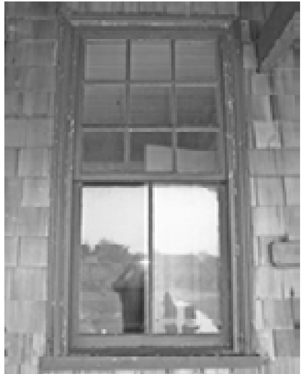
FIGURE 76. View of W-2, a typical nine-over-two window. (T. Jones, NPS, 2005)
