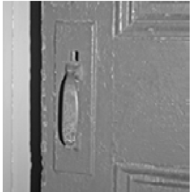
FIGURE 83. View of historic handle and escutcheon on door D-2. (T. Jones, NPS, 2005)
