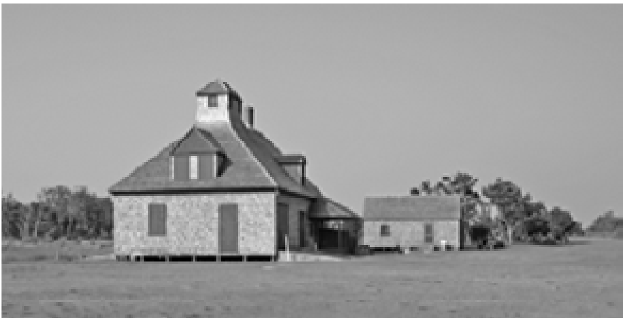
FIGURE 57. View southwest of station (T. Jones, NPS, 2005)
