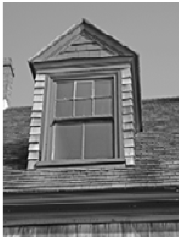
FIGURE 77. View of southeast dormer. (T. Jones, NPS, 2005)
