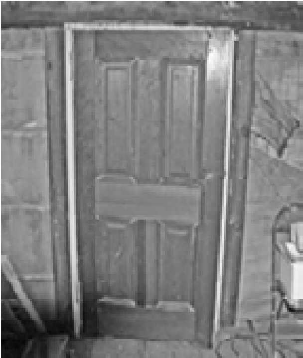
FIGURE 146. View of attic door. (T. Jones, NPS, 2005)
