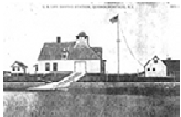
FIGURE 7. Tolman's station at Quonochontaug, Rhode Island, the prototype for the Portsmouth station. (From York, Architecture of the United States Life-Saving Service )
