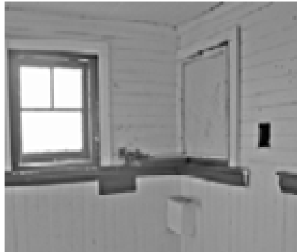
FIGURE 151. View of east corner of room. (T. Jones, NPS, 2005)
