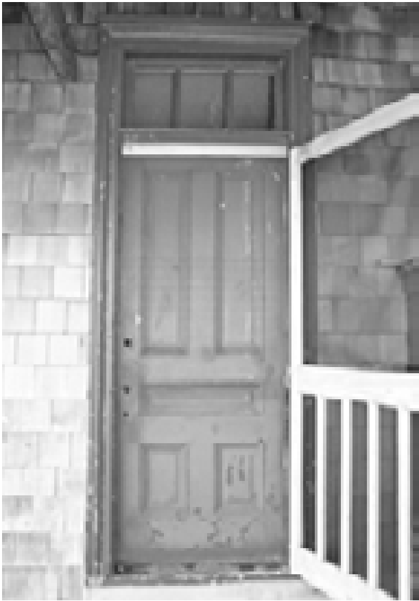
FIGURE 78. Door D-1 on northwest side of house. (T. Jones, NPS, 2005)
