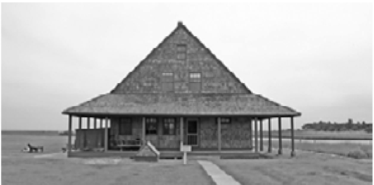
FIGURE 70. View porch wrapping northwest end of building. (T. Jones, NPS, 2005)
