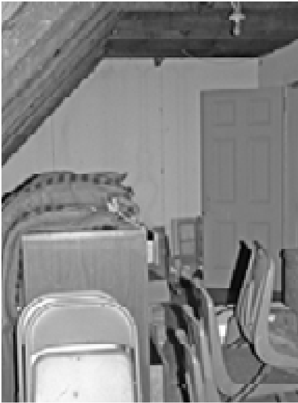
FIGURE 139. View northwest in Room 203. (T. Jones, NPS, 2005)
