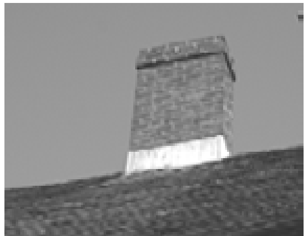
FIGURE 60. View of southeast side of chimney. (T. Jones, NPS, 2005)
