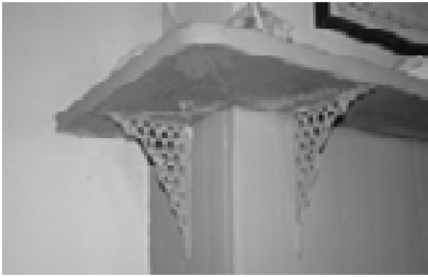
FIGURE 106. View of mantel shelf in Room 104. (T. Jones, NPS, 2005)
