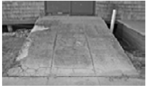
FIGURE 59. View of ramp to Boat Rooms doors D-5. (T. Jones, NPS, 2005)
