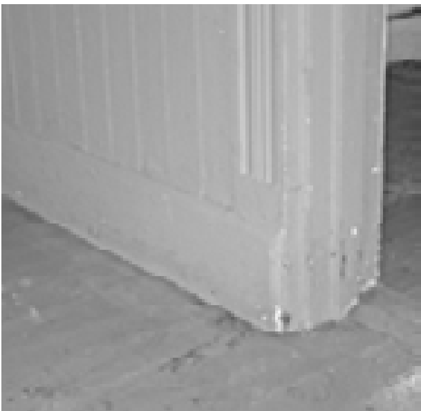
FIGURE 90. View of typical flooring, wainscot, and baseboard. (T. Jones, NPS, 2005)
