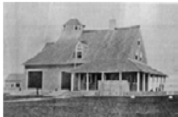
FIGURE 8. View of Core Bank Life-Saving Station prior to its expansion and remodeling in 1934. Note the stone foundation, which the Portsmouth station did not have. (CALO Coll.)
