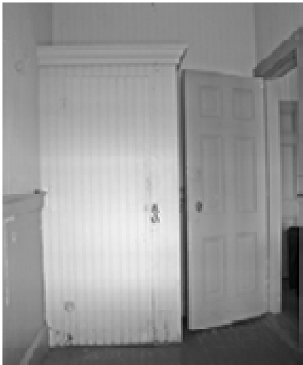
FIGURE 94. View northeast in Room 101. (T. Jones, NPS, 2005)
