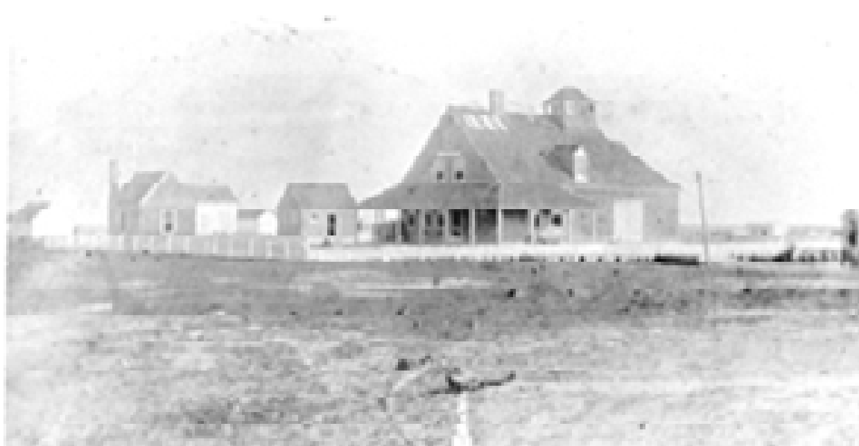
FIGURE 29. Portsmouth Coast Guard Station, c. 1920. (CALO Coll. A-01)
