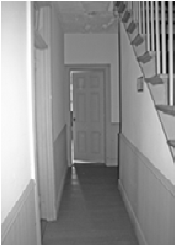
FIGURE 111. View northeast in Room 105. (T. Jones, NPS, 2005)
