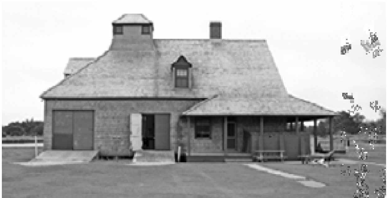
FIGURE 58. View southeast. (T. Jones, NPS, 2005)
