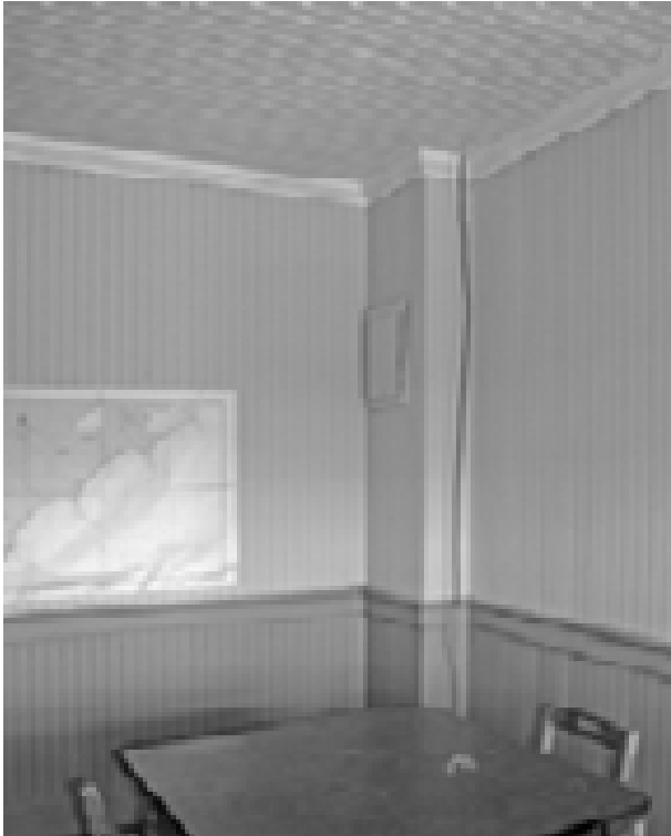
FIGURE 97. View east in Room 102. (T. Jones, NPS, 2005)
