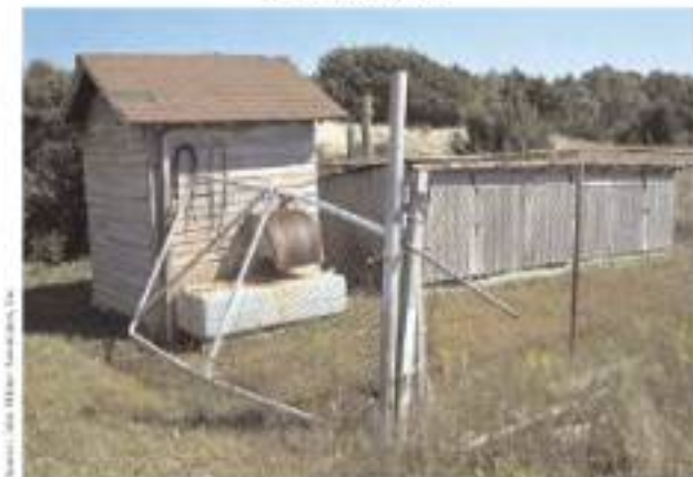
Figure 3-146. Adjacent to a village residence, chain-link fencing surrounds an area that may have been used as a dog penning.
