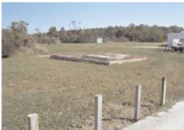
Figure 5-133. Wood post bollards edge the Concrete Road as it leads into the former Coast Guard Station.
