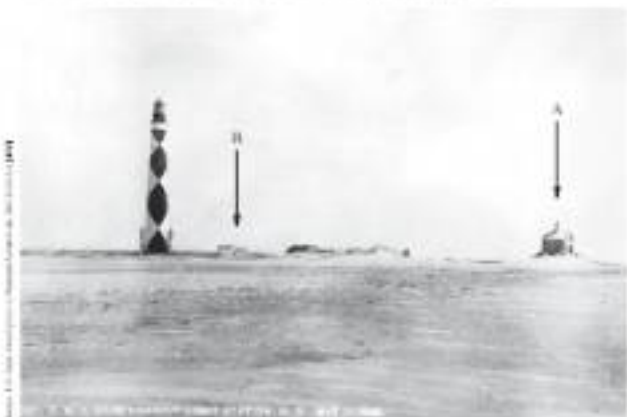
Figure 2-6: Cape Lookout Light Station, 17 May 1909, looking north. The 1875 Knappe's Dwelling is directly behind the lighthouse; at right (A) is the original circa 1812 Knappe's Dwelling. The 1889 wooden outbuildings (H) are also visible. The 1812 lighthouse likely stood on the dunes at center.
