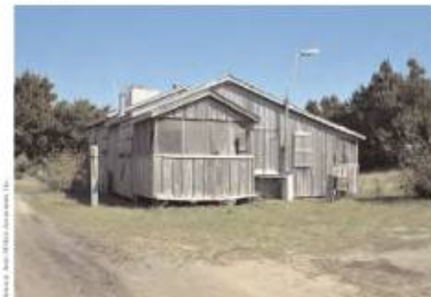
Figure 3-147. Overhead lighting lights the exterior of their residence.
