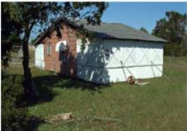
Figure 5-15. The Cook II Clothing House has screened porches across the front and back.
