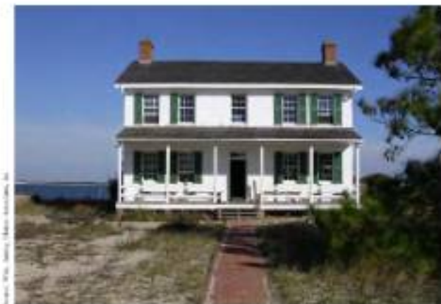
Figure 3-66. The Lighthouse Keeper's Quarters has been rehabilitated for use as a visitors' station.
