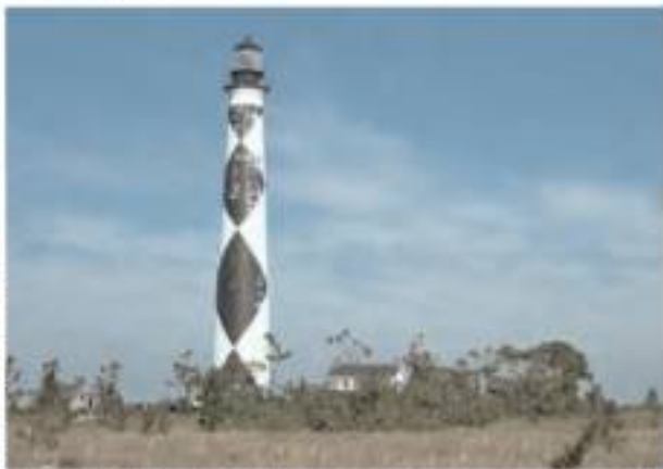
The same view in 2003. Note that the tall pine trees enclosing the Lighthouse have grown considerably, and the point on the lighthouse is peeling. The utility pole on the left in the photo has been removed.
