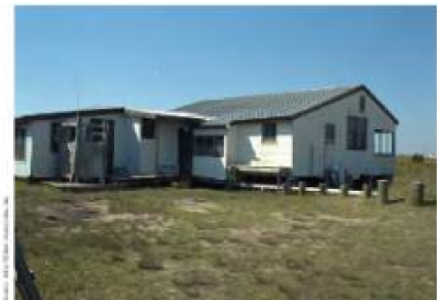
Figure 3-82. Jitty Workers House II has an irregular addition at the rear.
