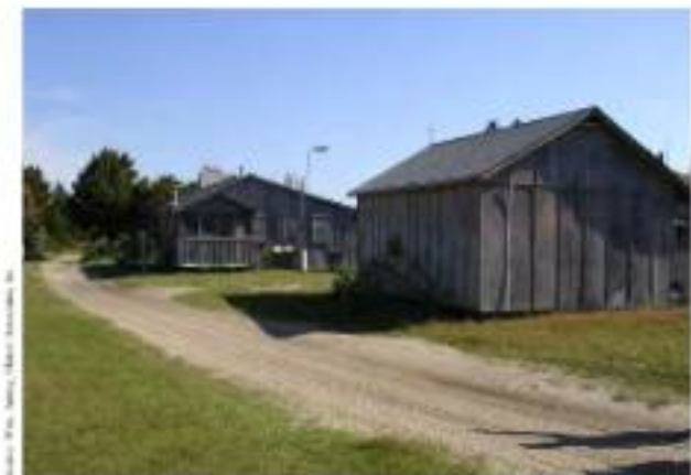
Figure 3-B6. The Service Delivery Home and its garage are clad with unpainted wood board and batten siding.
