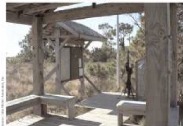
Figure 5-118. A bulletin board type kiosk in the picnic area can be used to post information.
