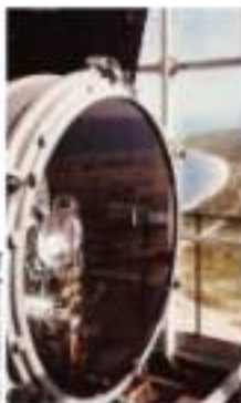
Figure 2-38. The new electric lantern of the Cape Lookout Lighthouse, installed in 1979, photograph circa 1983.
