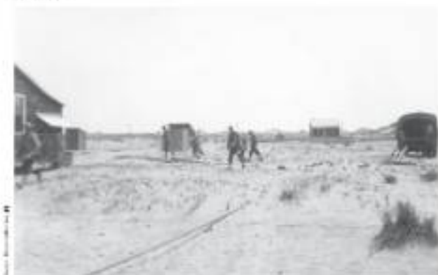
Figure 2-14. Army troops at Cape Leslie Village, circa 1942. The house with the porch visible at the left edge of the photograph is Mrs. Carrie Davis' House (destroyed). The house in the distance is probably the George Bone House (destroyed).
