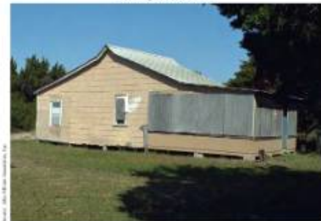
Figure 3-11. The O'Boyle-Bryant House is a typical one-story wood frame cottage.
