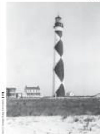
Figure 2-23. Cape Lookout Light Station, view from the southwest, circa 1940s. From left, the buildings are the 1807 Keeper's Dwelling, the 1875 Keeper's Dwelling, the Lighthouse, and an 1890 outbuilding.
