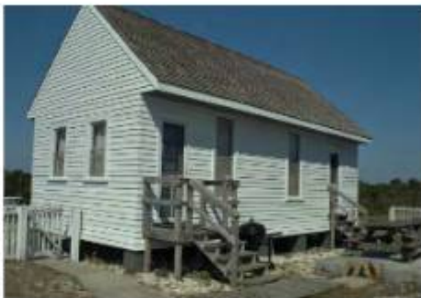
Figure 3-98. The Coast Guard kitchen is a one-story building adjacent to the main building.
