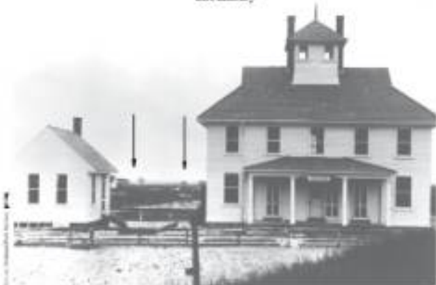
Figure 2-8. The newly constructed Coast Guard Station and kitchen building, circa 1917. A number of buildings in the Cape Lookout Village can be seen in the distance between the two station buildings (arrows). No individual buildings in the village are identifiable in this photograph.
