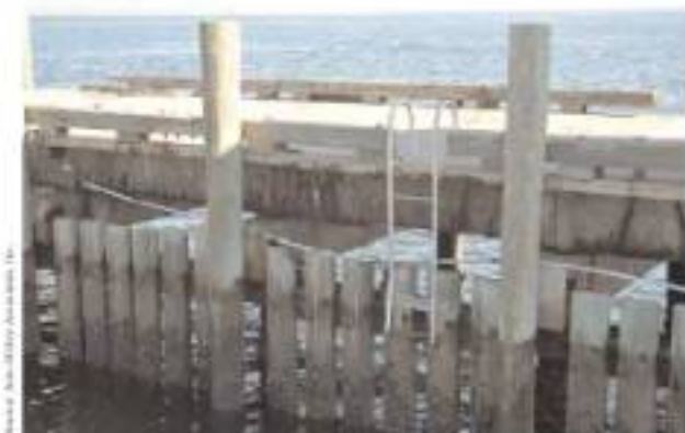
Figure 5-123. A wooden building on the Coast Guard dock for climbing between the dock and boats.
