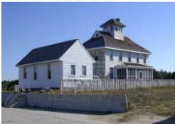
Figure 3-97. The U.S. Coast Guard Station main building was constructed in 1916–1917.
