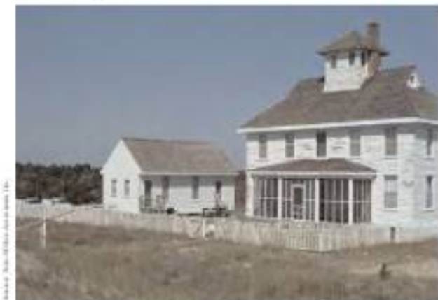
Figure 3-17. The Senior Coast Guard Station also has a hip roof to protect against wind damage during hurricanes.
