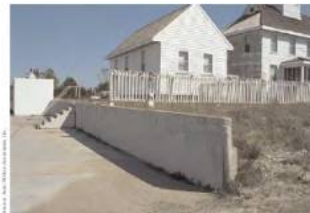
Figure 3-23. A concrete retaining wall along the Fort Stevens Guard Station parking lot.
