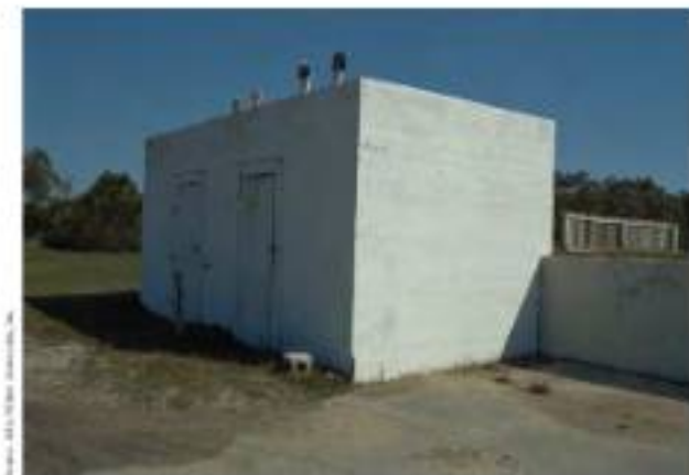
Figure 3-100. Built as the concrete retaining wall at the Coast Guard station is this concrete utility building.
