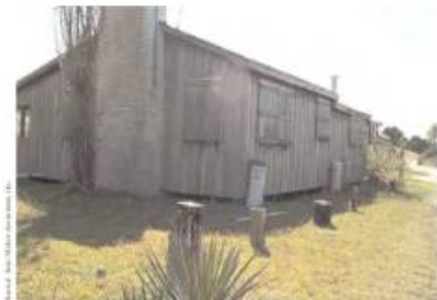
Figure 3-141. The fuel siding composed of logs set into the ground edges this house in the village.
