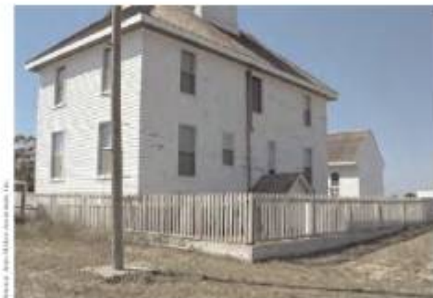
Figure 3-135. A white-painted wooden picket fence encloses the yard around the former Coast Guard Station building.
