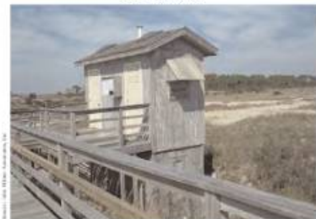
Figure 5-122. Signs and temporary information bulletins are posted on the visitor access station building near the beach.
