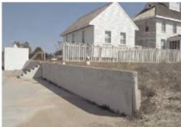
Figure 3-137. A concrete block retaining wall edges the parking area below the Coast Guard Station concrete kitchen.
