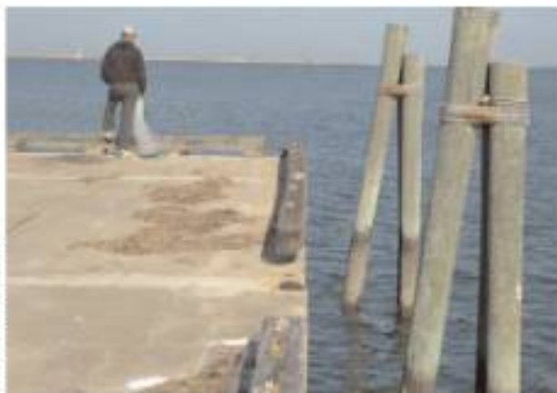
Figure 3-61. The Coast Guard dock is a concrete slab mounted on wooden pilings and edged by bolted pilings.
