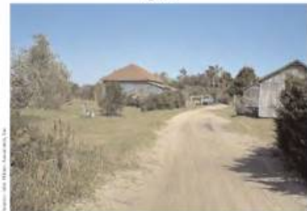
Figure 3-53. Foundation plants edge many of the buildings within the village as seen on the left.
