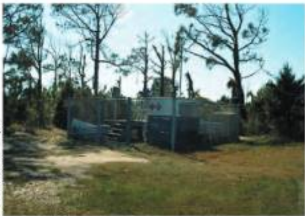
Figure 3-35. Existing condition of chain-link fence surrounding material storage.
