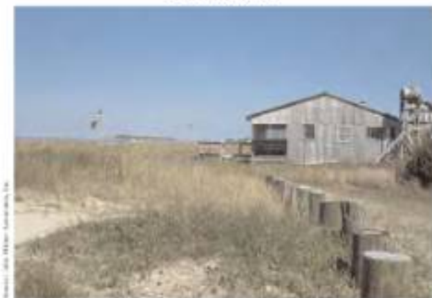
Figure 5-142. Rustic edging composed of treated pilings.
