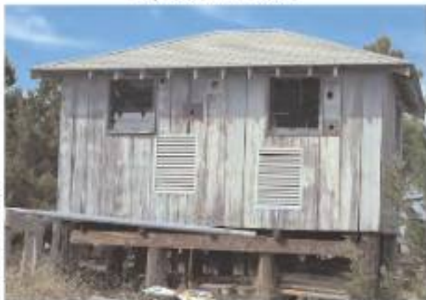
Figure 3-20. Another example of a building located on the cape with a low-angle hip roof, raised foundation, and wood construction.
