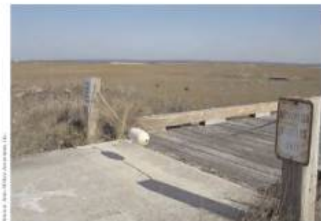
Figure 5-111. Signs along the Concrete Road note that only authorized vehicles are permitted to access the road leading to the dock.
