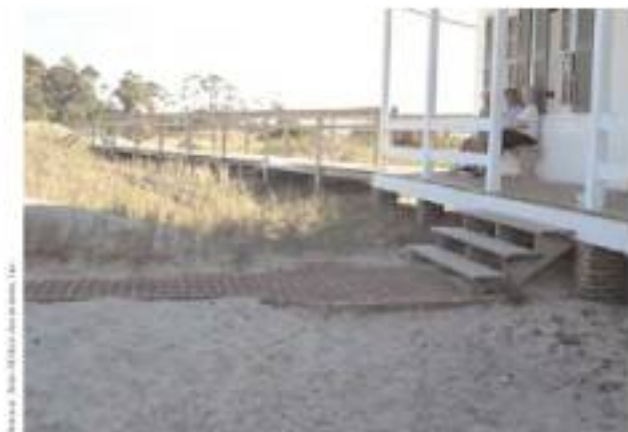
Figure 5-127. Wood benches without backs are located on the front porch. A brick walk provides access from the right side beach.
