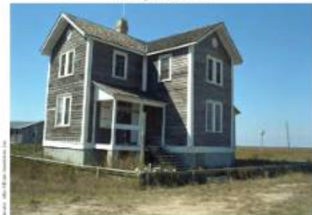
Figure 3-79. The kitchen porch of the Barden House.
