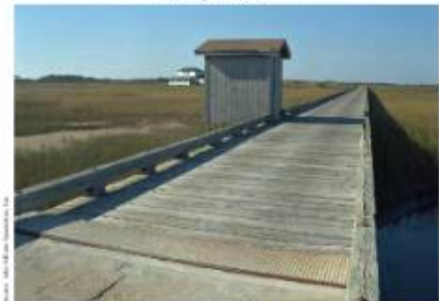
Figure 5-107. One NPS storage shed is near the shoreline at the Coast Guard dock.
