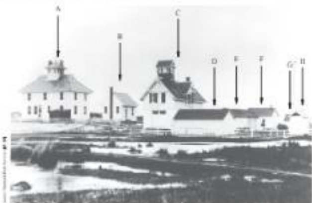
Figure 2-8a. The Coast Guard Station, circa 1917, looking south. Note the standing water and swampy conditions in the foreground. A: 1917 Coast Guard station/main building; B: 1917 kitchen; C: 1907 Life-Saving Station, relocated 1916; D: 1902 Icehouse; E: 1902 stable; F: 1902 kitchen, relocated 1917; G: 1908 storage building, relocated 1917; H: privy.
