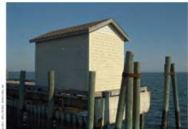
Figure 5-108. A second NPS storage shed is on the dock itself on pilings in the light.
