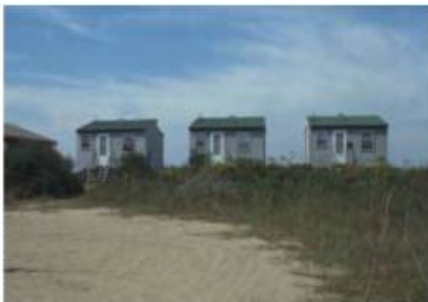
Figure 3-74. The three small wood cabins at the Moore complex are identical wood frame buildings.
