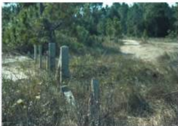
Figure 3-33. Additional concrete fence posts survive behind the summer kitchen. These may be useful when reconstructing or interpreting the missing fence line around the lighthouse precinct.
