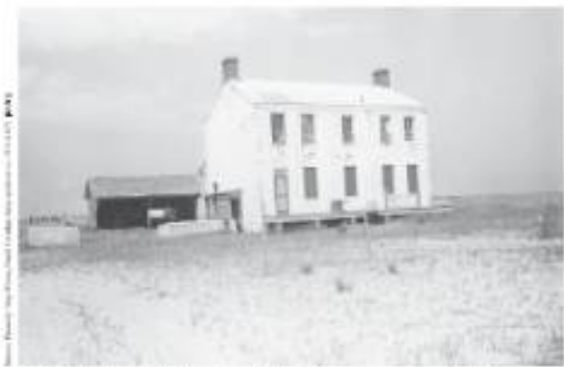
Figure 2-33. 1878 Keeper's Dwelling and coal shed, 1970 condition survey photograph. Note the wooden lean-to at the west gable with a full chimney and the absence of a porch across the south side of the building.
