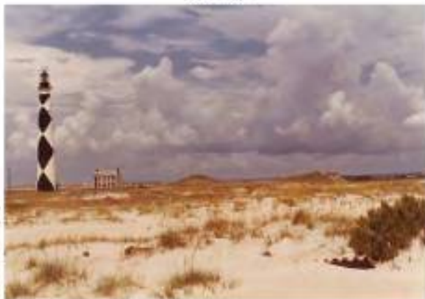
Figure 2-28. Cape Lookout Light Station, view from the southeast, circa 1960s.
