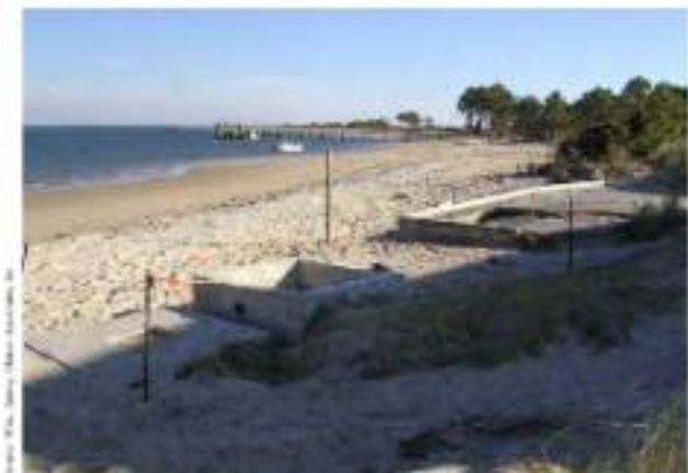
Figure 3-68. The concrete and steel foundation is next to a concrete cistern in the foreground of this photograph.
