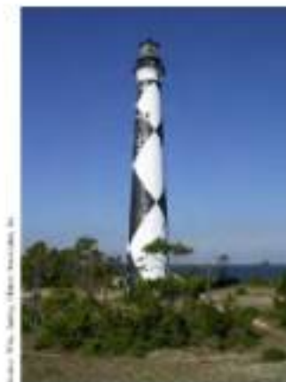
Figure 7-64. The Cape Lookout lighthouse is a brick masonry structure painted with a black and white diagonal checker pattern.
