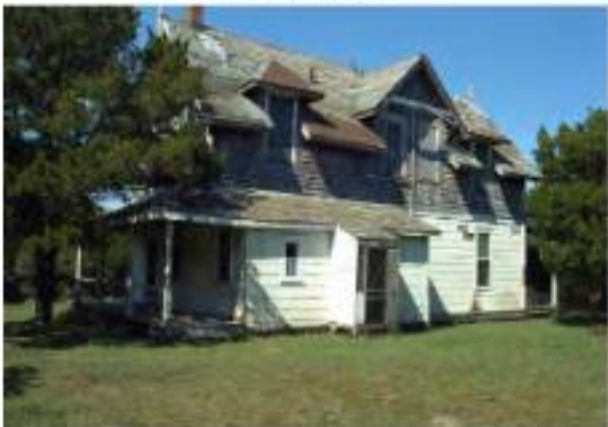
Figure 3-85. The 1937 Life-Saving Station (Wells-Branch House) was moved to its current site at the north end of the village in 1958.
