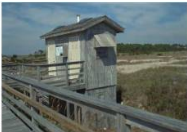
Figure 3-70. The conflict station near the ocean beach is a recent wood frame building constructed by NPS.
