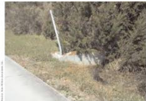
Figure 5-139. A small foundation constructed of concrete block with brick along the top is located across from the former Coast Guard Station garage.
