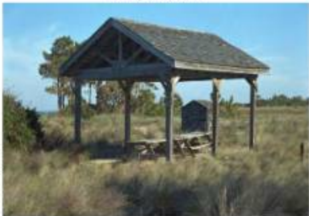
Figure 3-71. Atypical timber picnic shelter, constructed by NPS.
