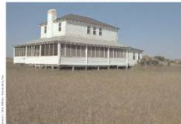
Figure 3-16. Castiblanco is a typical cape residential structure—wooden, balloon-framed, with a low-angle hip roof and set on a raised foundation.
