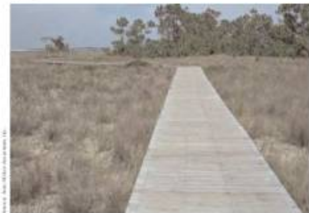
Figure 3-49. A new boardwalk crosses the closed grassland area between the lighthouse precinct and beach access/boardwalk area.
