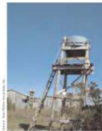
Figure 3-21. One of the elevated building tanks for storage of fresh water on Cape Lookout.
