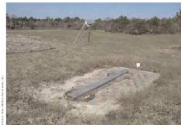
Figure 3-153. Water-related utility features include cisterns or septic features associated with the concrete and metal manhole covers around the Entrance Guard Station.
