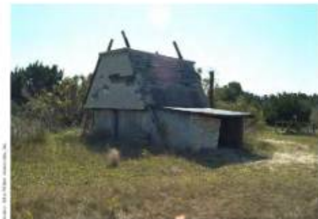
Figure 3-80. There is a small storage shed adjacent to the Barden House.
