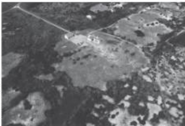
Figure 2-31. Aerial view of the Coast Guard Station, circa 1970s. Many of the buildings at the station had been demolished or razed to new sites in the years following 1945. The site is surrounded by pine trees.
