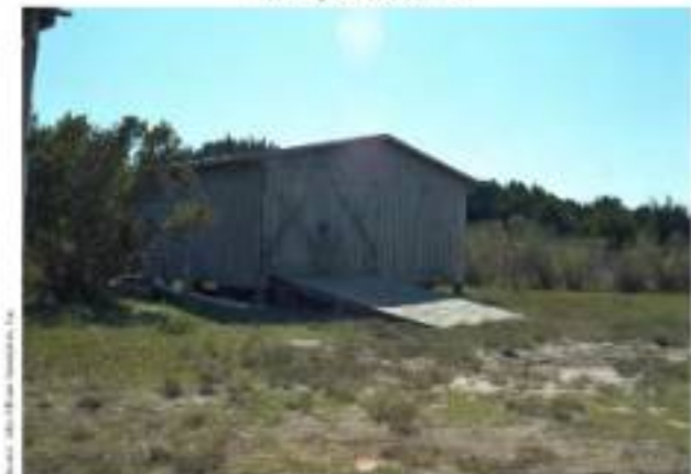
Figure 3-43. There is a separate garage building adjacent to Jetty Workers House II.
