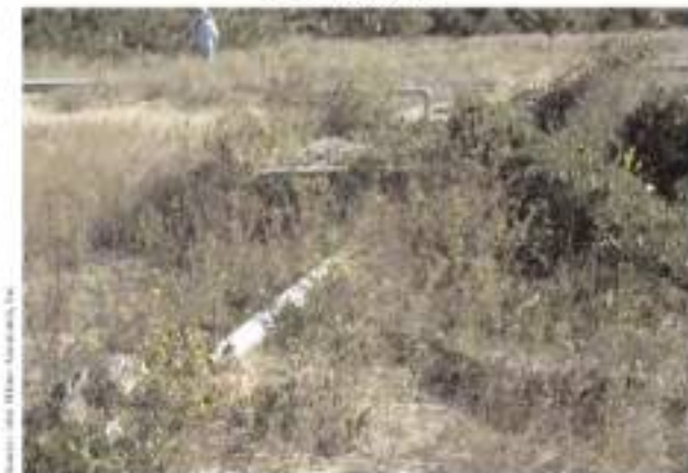
Figure 3-156. Other utility features include a galvanized standing pipe and exposed PVC pipe near the lighthouse.
