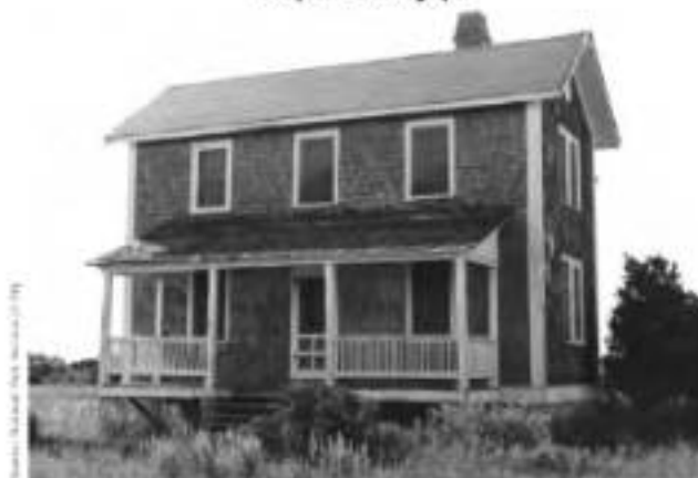
Photo Pair 10. Front view of Barker house, looking east, ca. 1970s, showing front porch.
