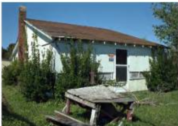
Figure 3-90. The Lathier Craftsman House (Craftsman Cottage) is a one-story wood frame cottage.
