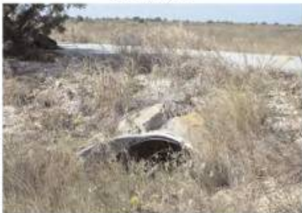
Figure 5-132. A metal culvert runs under the Concrete Road and helps drain an area that is subject to frequent flooding.
