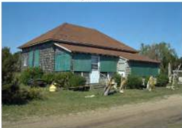
Figure 3-89. The Coast Guard Station boathouse (Voinovich House) has a hip roof and is clad with painted wood shingles.
