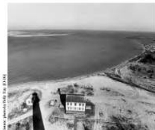
Figure S-12. The same view, 1979. Significant erosion over this six year period suggests the need for a shoreline management plan.
