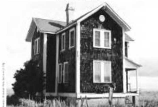
Photo Pair 11: View of Hamilton House, looking southeast, ca. 1970s
