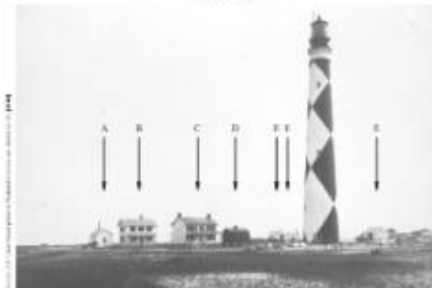
Figure 2-7. Cape Lookout Light Station, view from the southwest, 10 July 1913. The buildings on land the lighthouse are: A, 1907 annex kitchen; B, 1907 Keeper's Dwelling; C, 1873 Keeper's Dwelling; D, circa 1907 iron oil house; E, various 1900 outbuildings.
