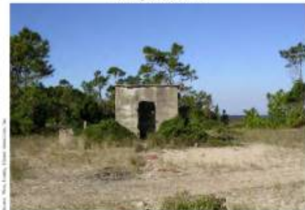
Figure 3-65. The oil shed adjacent to the lighthouse is a cast-in-place concrete building.
