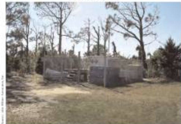
Figure 3-150: Chain-link fencing edges utility boxes near the former Coast Guard Station.
