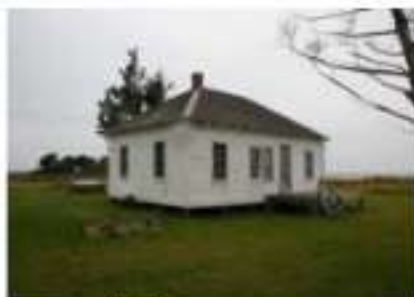
FIGURE 92. Frank Gaskill House.
