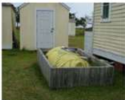
FIGURE 125. An above-ground septic tank and wooden enclosure at the Jesse Robb House.
