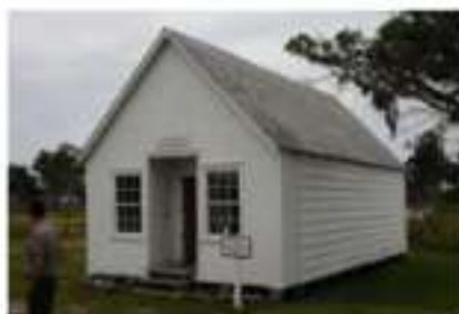
FIGURE 87. Portsmouth Post Office.
