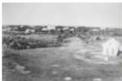
FIGURE 105A. View of Portsmouth Village looking west from the Portsmouth Life-Saving Station watchtower, circa 1906.
