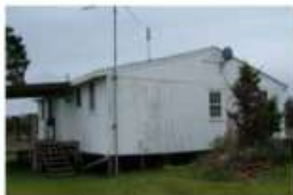
FIGURE 185B. The same view in 2006. Note the addition to the building along its rear facade, the removal of the screened porch, replacement of the siding, and the addition of a deck.
