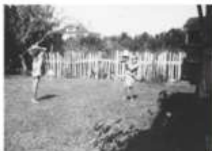
FIGURE 101A. Looking toward the Dixon-Salter House from the immediate front of the Robert Wallace House, circa 1942.
