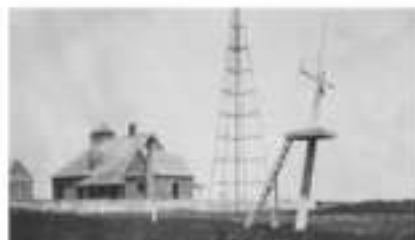
FIGURE 101A. Looking east toward the Portsmouth Life-Saving Station and kitchen, including the station's wreck pole, coastal warning display tower, and oil house, circa 1916. Wood board fencing enclosed the complex.
