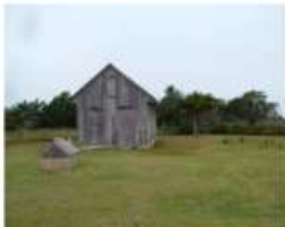
FIGURE 108. The well house near Portsmouth Life-Saving Station stable.
