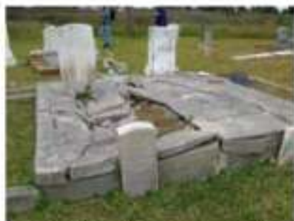
FIGURE 208. Cracking and displacement of concrete vaults can allow water to percolate, accelerating deterioration of the features.
