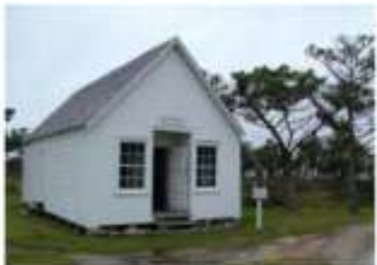
FIGURE 187B. the same view today. Changes since the 1930s include the loss of the addition, and removal of the porch and overhang. The vent pipe in the rear is also gone. The side door indicates the former connection between this building and the missing addition.
