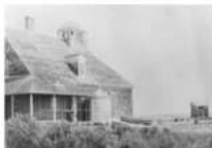
FIGURE 100A. View toward the southeast side of the Portsmouth Life-Saving Station, circa 1942.
