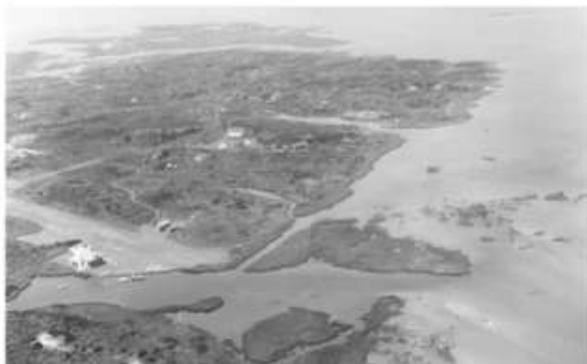
FIGURE 26. Aerial photograph of Portsmouth looking northwest, 1963. The Life-Saving Station is visible in the left foreground, with the cleared landing strip separating the station from its stable and shed. The church is at the center of this view, and the schoolhouse is visible at the left edge of the photograph.
