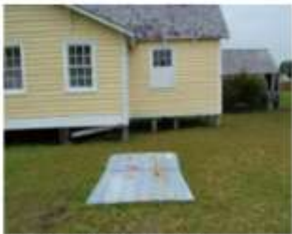
FIGURE 124. The Dennis Mason septic tank.
