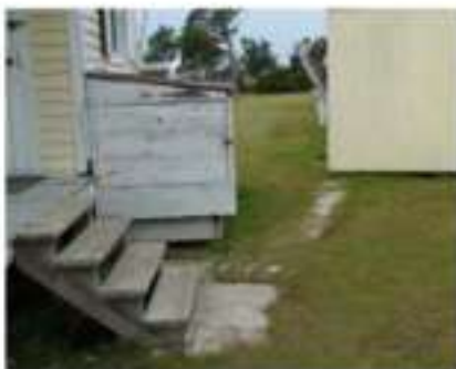
FIGURE 101. The Jesse Rabb water box is attached to the side of the house.
