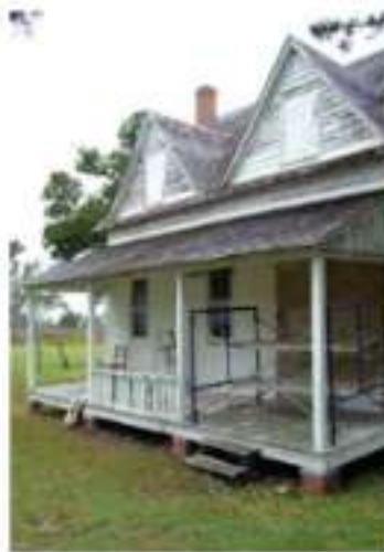
FIGURE 178B. The same view in 2006. Note the replacement of the central dormer with two dormers and alteration of the porch posts and railing. Woodwork beneath the porch is no longer present.
