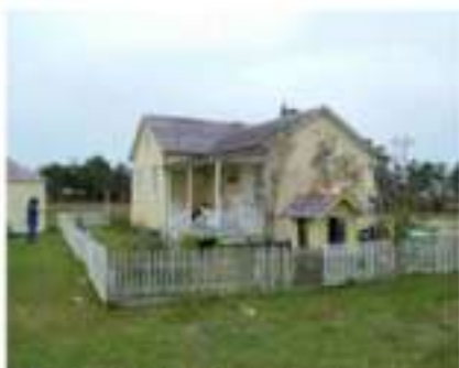
FIGURE 116. The picket fence around the McWilliams-Dixon House precinct.
