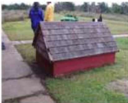
FIGURE 109. The pump house near the Portsmouth Life-Saving Station.
