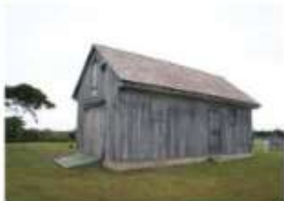
FIGURE 78. The stable at the Life-Saving Station.
