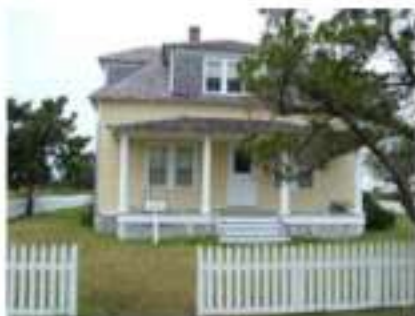
FIGURE 176B. The same view in 2006. Note the shingling of the second story, change in lattice under the porch, the addition of the picket fencing, and the loss of some
