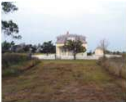
FIGURE 116. The picket fence around the Styron-Bragg House precinct.
