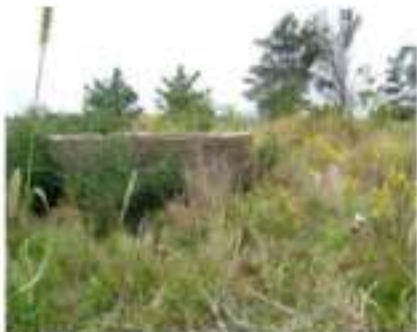
FIGURE 99. The concrete cistern near the Keller Seyron Cemetery.
