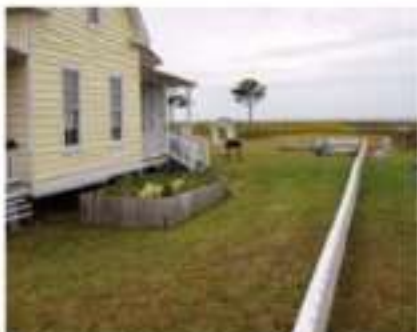
FIGURE 126. An above-ground septic tank and wooden enclosure at the Henry Pigott House.
