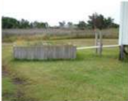
FIGURE 123. An above-ground septic tank at the Y. Y. Potter House.
