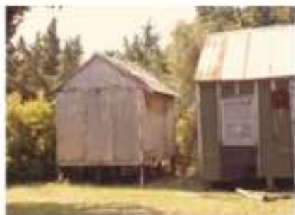
FIGURE 164A. Looking southeast toward a storage shed east of the Carl Dixon House outbuilding, circa 1979.
