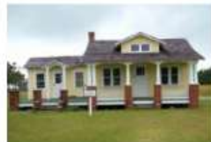
FIGURE 189B. The same view in 2006. Note the loss of the decorative trellis on the porch, the pickets along the side addition, the low fencing like that at the Tallie House, and the change in mortar associated with the brick.
