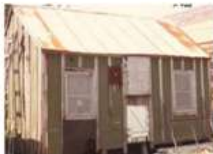
FIGURE 102A. The north facade of the outbuilding east of the Carl Dixon House, circa 1978.
