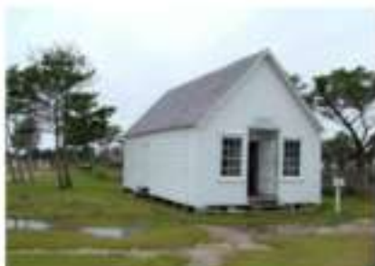
FIGURE 188B. The same view today. Changes since the 1930s include the loss of the addition, and removal of the porch and overhang. The vent pipe in the rear is also gone.
