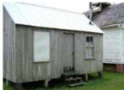
FIGURE 102B. The same shed in 2006. Changes visible between the photographs includes the boarded window, different cladding of the shed, the addition of a vent pipe, replacement of the door, addition of wooden steps, lack of paint, and the addition of the widow's walk to the roof of the adjacent Carl Dixon House.
