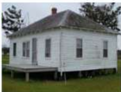
FIGURE 184B. The same view today. Note the loss of the roof overhang associated with the porch and the wood stain and landing along the side of the house. The vegetation is now mown cool-season grass, whereas the earlier view suggests native warm-season grasses were present previously. Cabling is currently stabilizing the structure.
