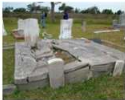
FIGURE 131. The condition of some of the concrete vault covers in the Community Cemetery is poor.
