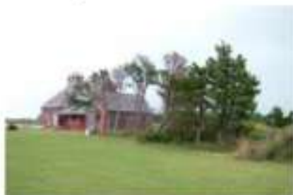
FIGURE 101B. The same view in 2006 indicating the loss of the wreck pole, warning tower, board fencing, and oil house. There is more vegetation within the vicinity today than during the period of significance.
