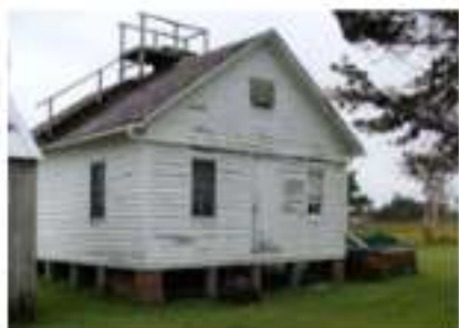
FIGURE 163B. The Carl Dixon House in 2006. Changes since 1979 include loss of the front porch, addition of the widow's walk, replacement of the roof, and a change in paint color.
