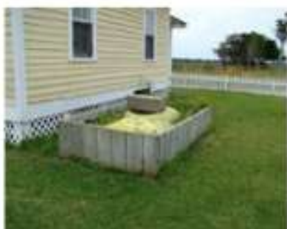
FIGURE 41. Above-ground septic systems are typically used for wastewater treatment and management in association with most buildings.
