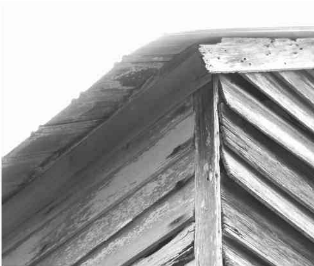
FIGURE 53. View of north corner of house, showing typical treatment of eaves and corners. Light areas appear to be paint but may actually be due to the presence of lichen or other natural discoloration. (NPS-SERO-CR, 2002)
