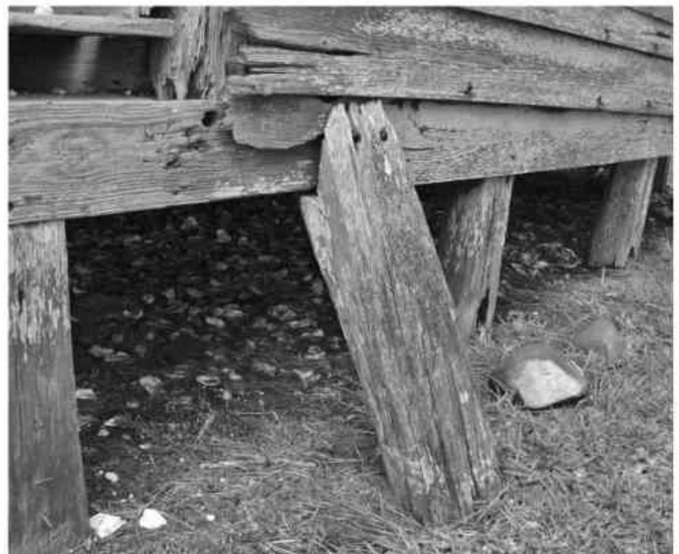
FIGURE 35. View of a typical "bird's-mouth" hurricane brace on north side of house. (NPS-SERO-CR, 2002)
