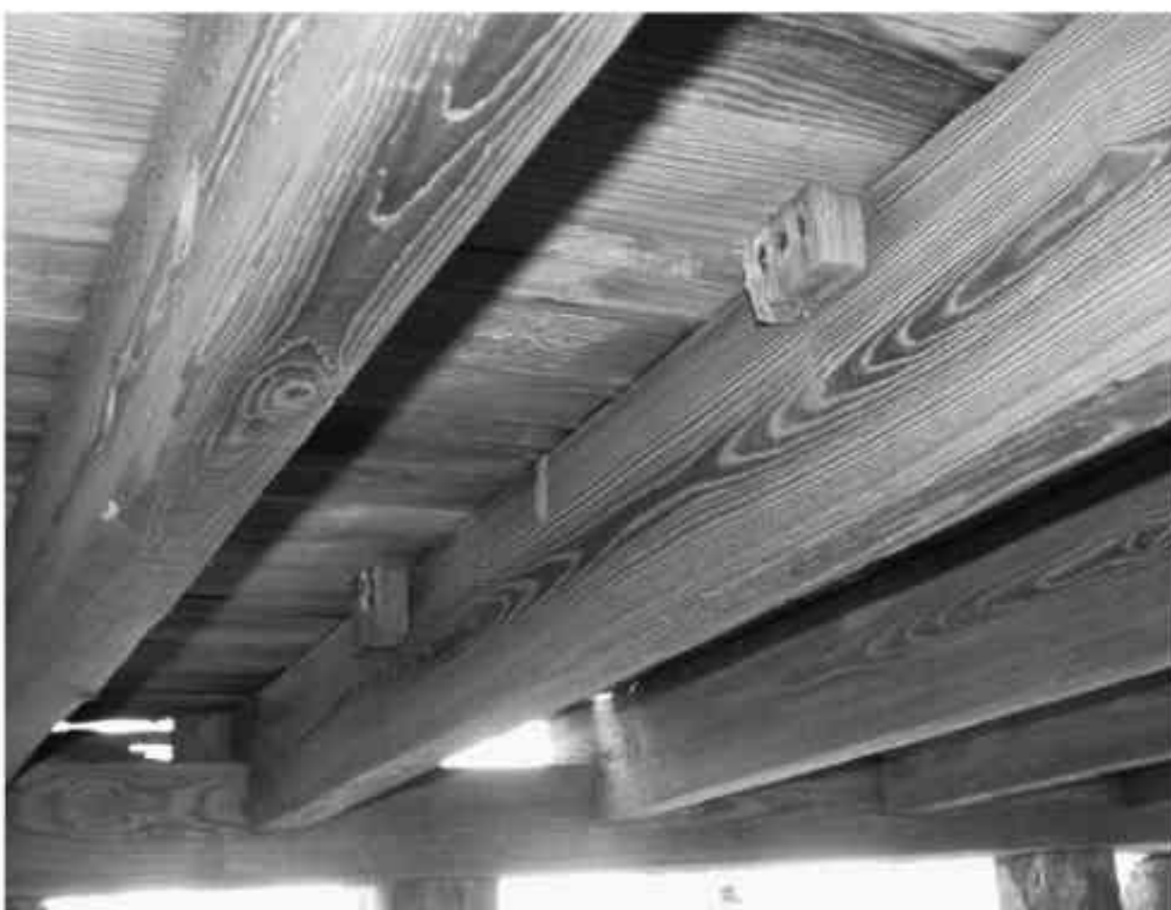
FIGURE 40. View of connection of wall studs and floor joist on east side of Room 101. (NPS-SERO-CR, 2003)
