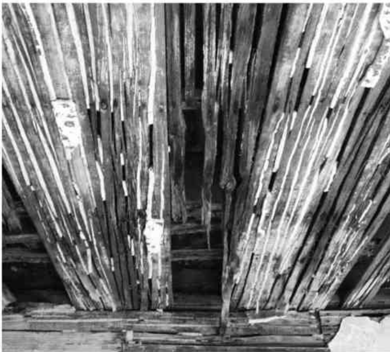
FIGURE 56. View of ceiling in Room 101, showing typical split-board plaster lath. (NPS-SERO-CR, 2002)
