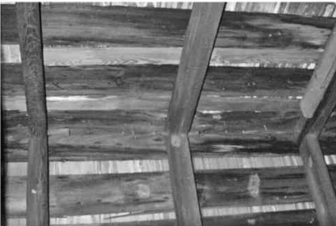
FIGURE 45. View of typical rafter connections at ridge. (NPS-SERO-CR, 2002)
