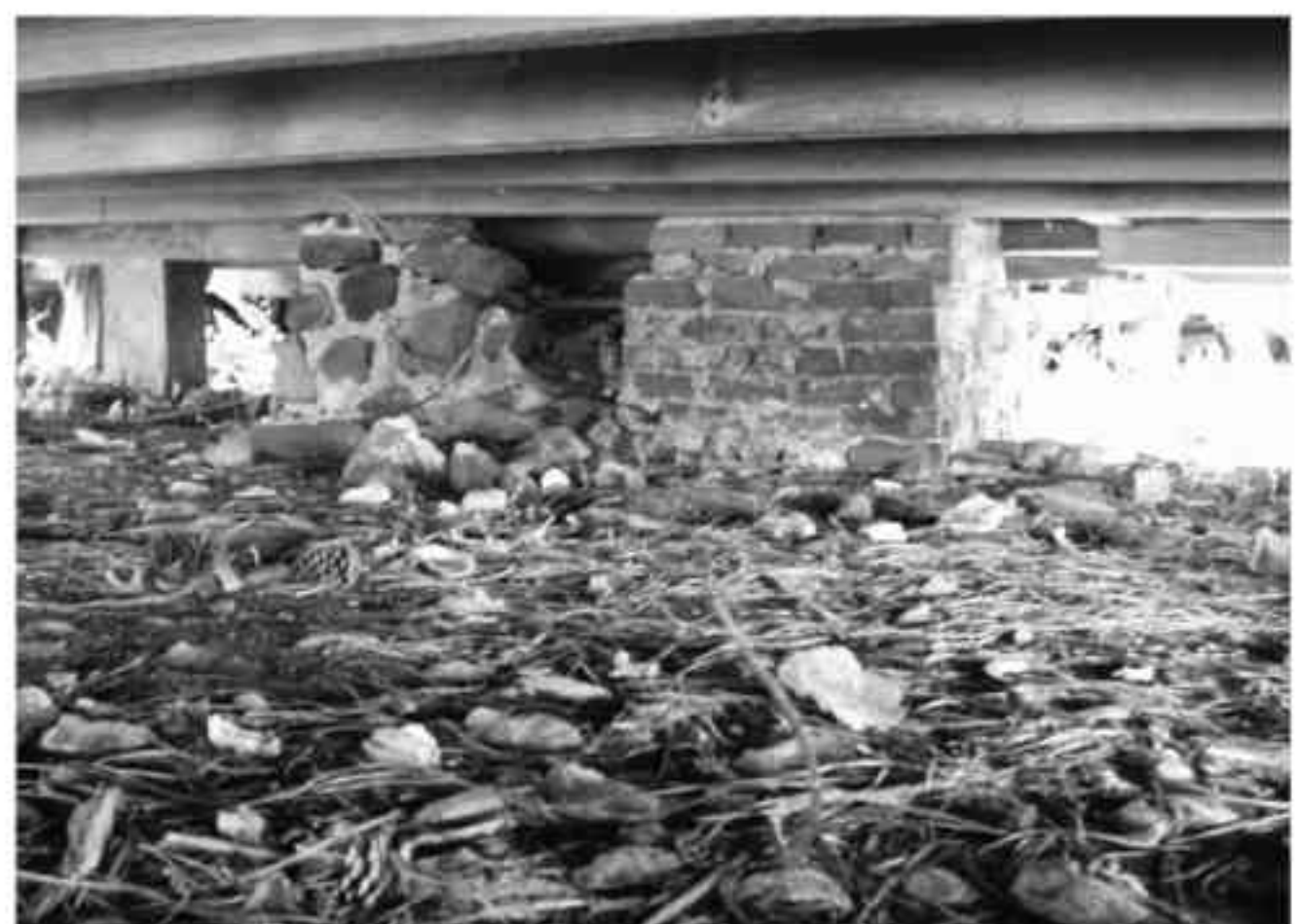
FIGURE 36. View of chimney foundation, with brick at right marking existing chimney base and stone at left marking larger extent of original chimney. (NPS-SERO-CR, 2002)
