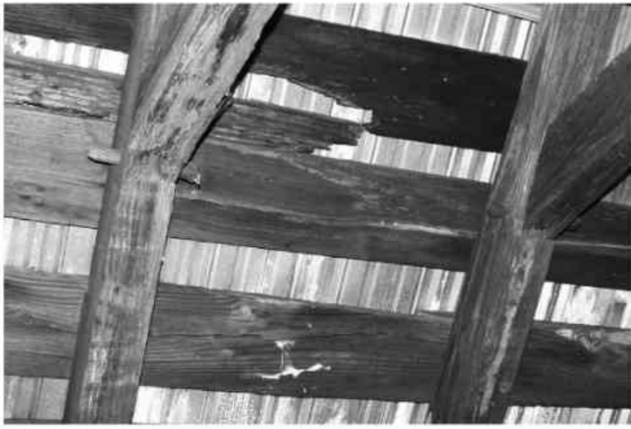
FIGURE 44. View of typical connection of collar beams and rafters. (NPS-SERO-CR, 2002)
