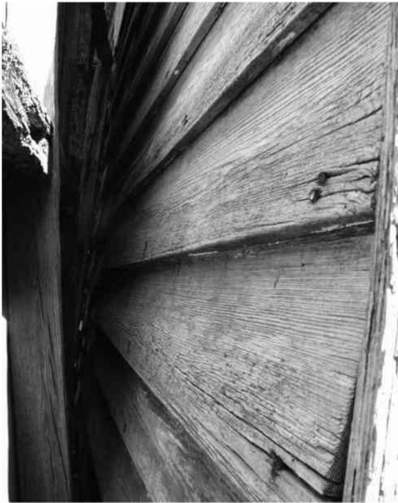
FIGURE 52. View of original beaded siding remaining on north west side of main block at kitchen addition. All of this siding was replaced in 2003. (NPS-SERO-CR, 2002)
