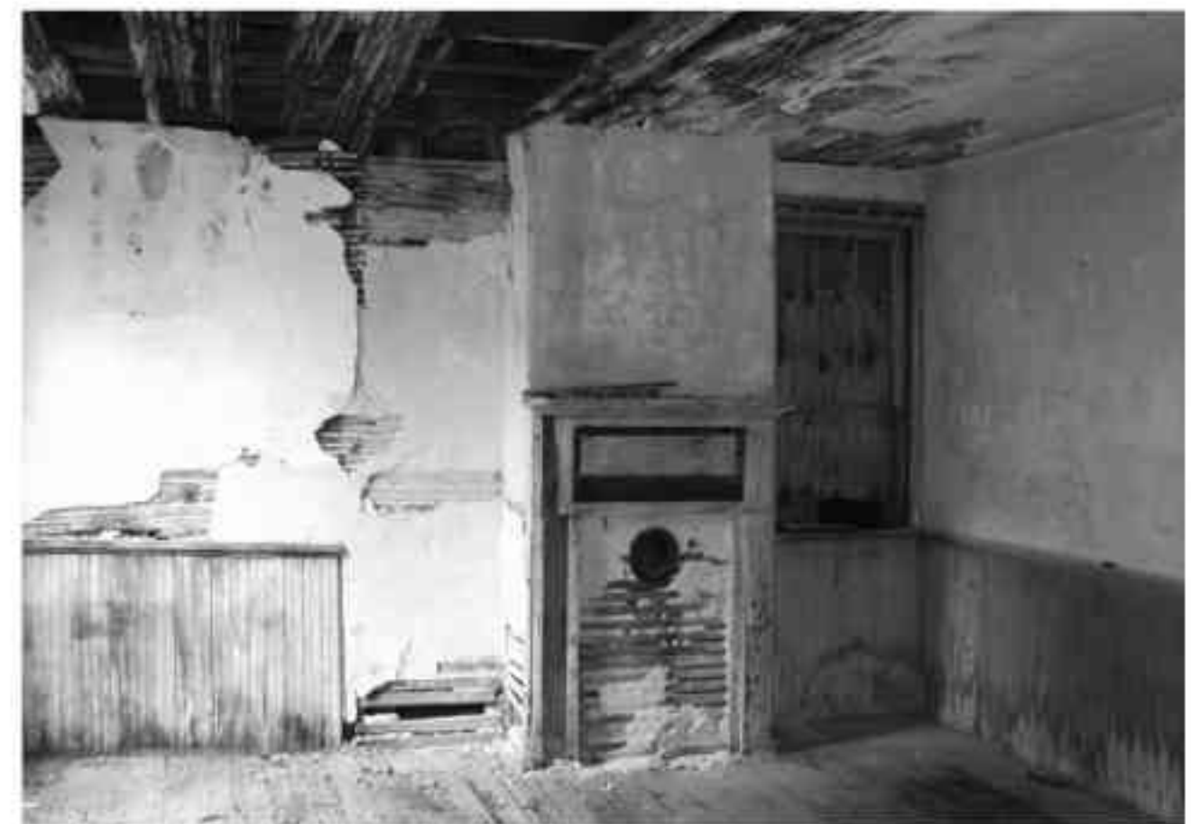
FIGURE 18. View of chimney in Room 103, absence of wainscot indicating extent of original chimney. (NPS-SERO-CR, 2003)
