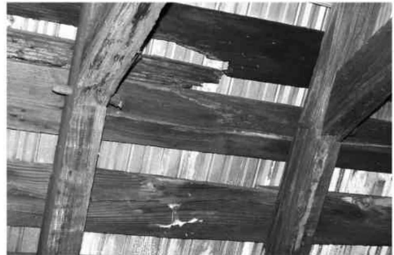
FIGURE 42. View of typical connection of collar beams and rafters. (NPS-SERO-CR, 2002)
