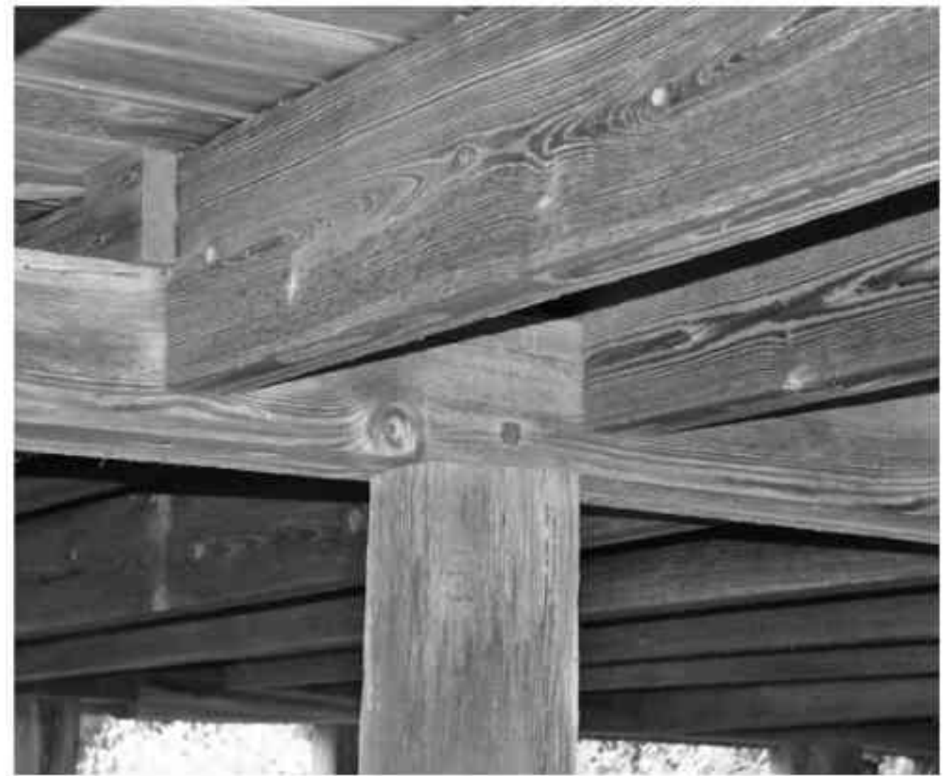
FIGURE 34. View of typical joist and pier connections at center beam. (NPS-SERO-CR, 2002)
