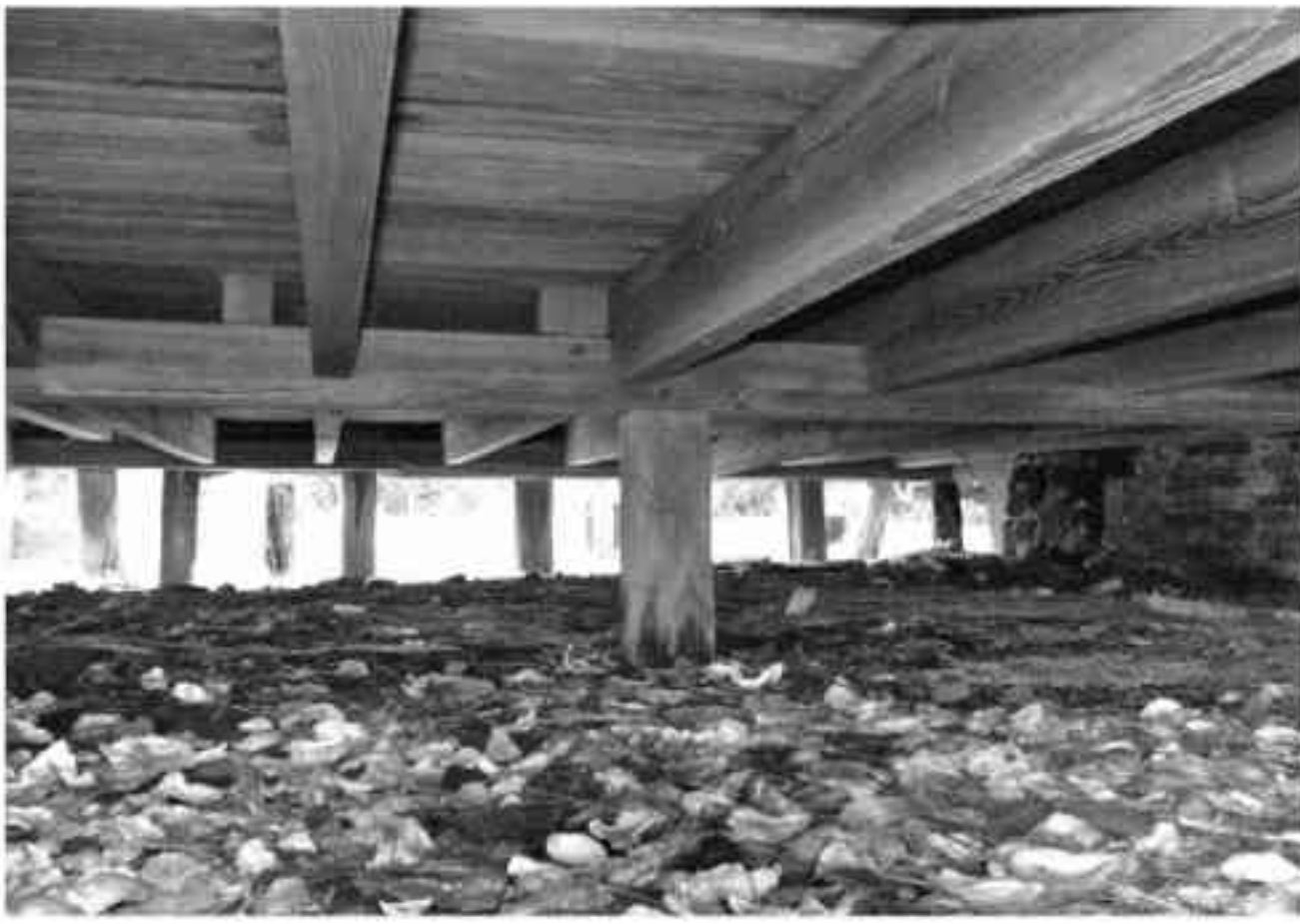
FIGURE 37. View southwest under main block of house, showing shells used to stabilize the ground under the house. (NPS-SERO-CR, 2002)
