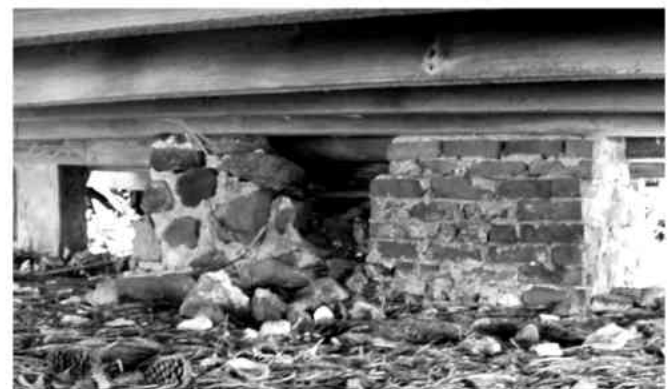
FIGURE 20. View of chimney base, with original stone chimney base at left, existing brick chimney at right. (NPS-SERO-CR, 2003)
