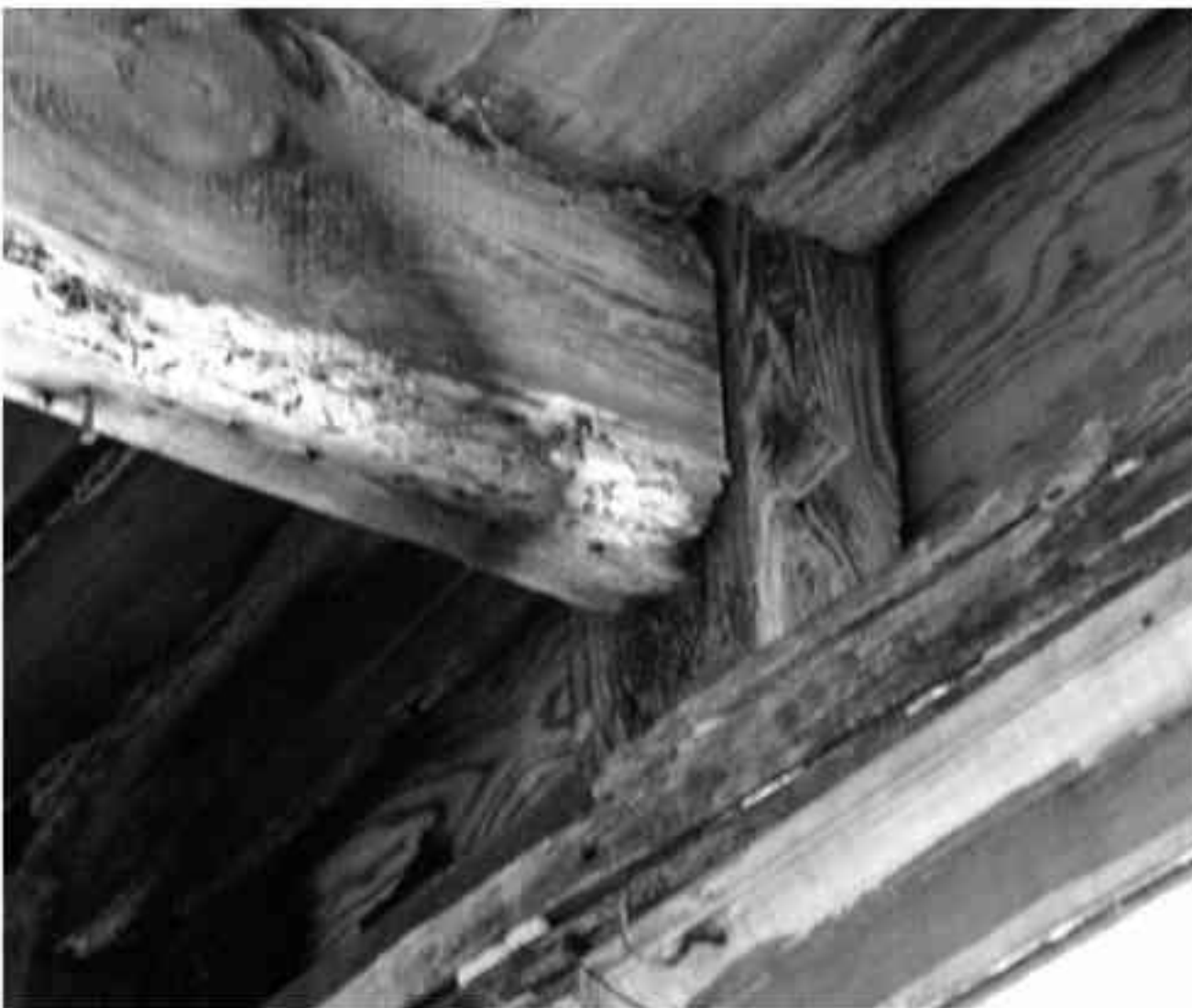
FIGURE 39. View of typical connection of second floor joists and studs. (NPS-SERO-CR, 2002)
