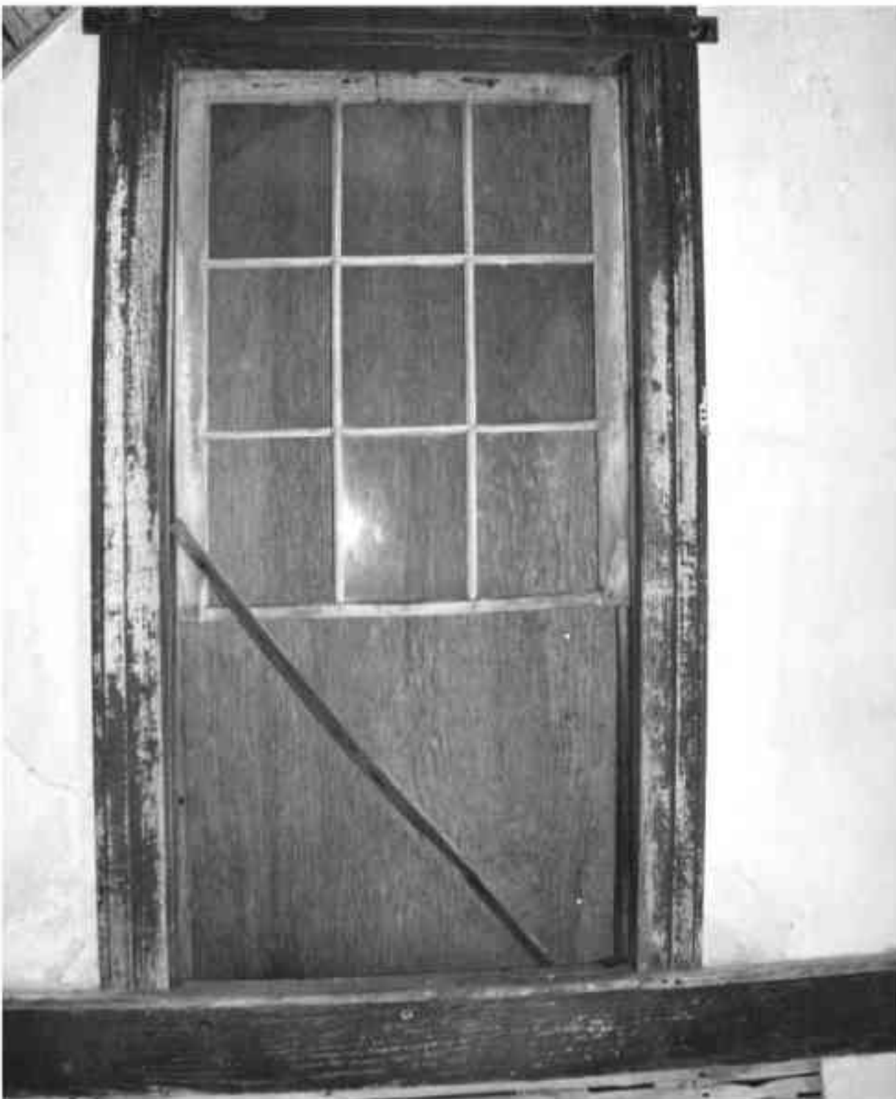
FIGURE 50. View of W-2 with sash and trim typical of first floor windows. (NPS-SERO-CR, 2002)
