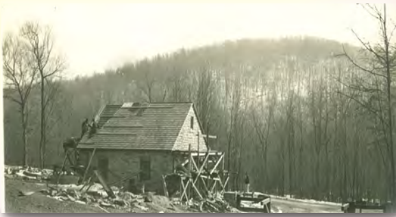
Building the Visitor Center in 1941.
