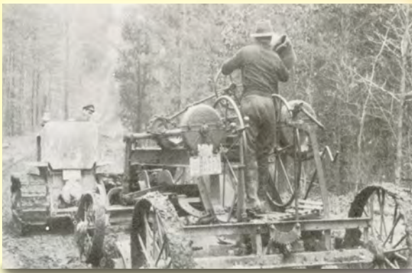
Members of the CCC working on road construction.
