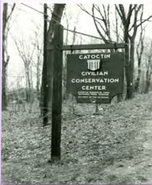
Historic Park Sign
