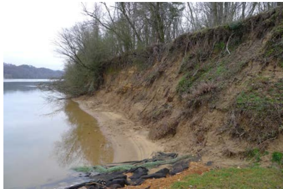
Figure 3.15: Riverbank erosion at Mallards Dozen site, 2012 (The Jaeger Company)
