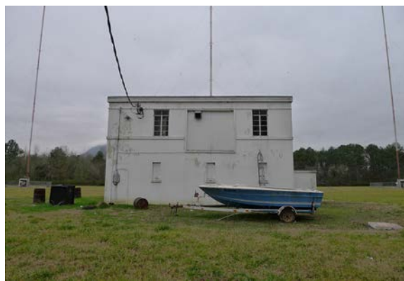
Figure 3.41: Two-story building at WDEF radio towers site, 2012 (The Jaeger Company)
