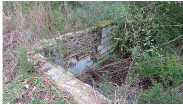
Figure 3.49: Figure 3.50: Remnant concrete wall, 2012 (The Jaeger Company)
