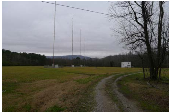
Figure 3.40: WDEF radio towers site, 2012 (The Jaeger Company)
