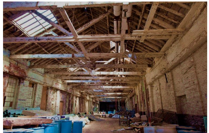
Interior of one of the forge/foundry buildings
