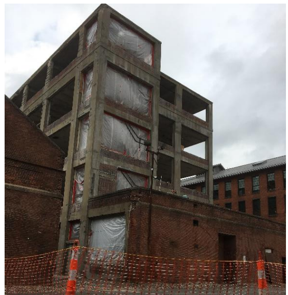
(North Armory under construction)
