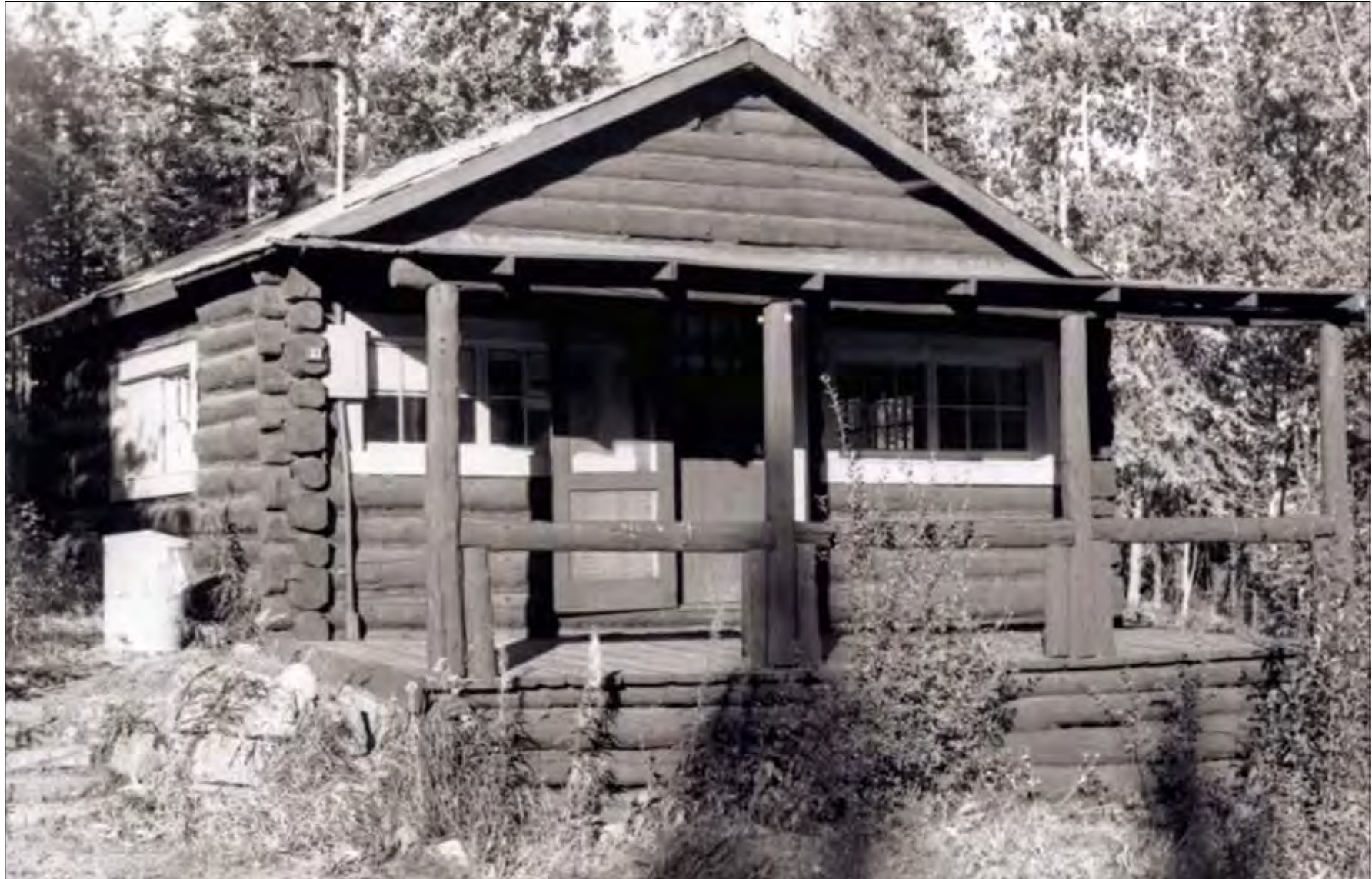
Figure 32. Building 22 (Office Building), view to the northeast, Catalog No. DENA 2225, n.d. (Denali National Park and Preserve Museum Collection Archives)
