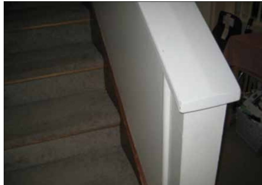
Stair Banisters in all units
