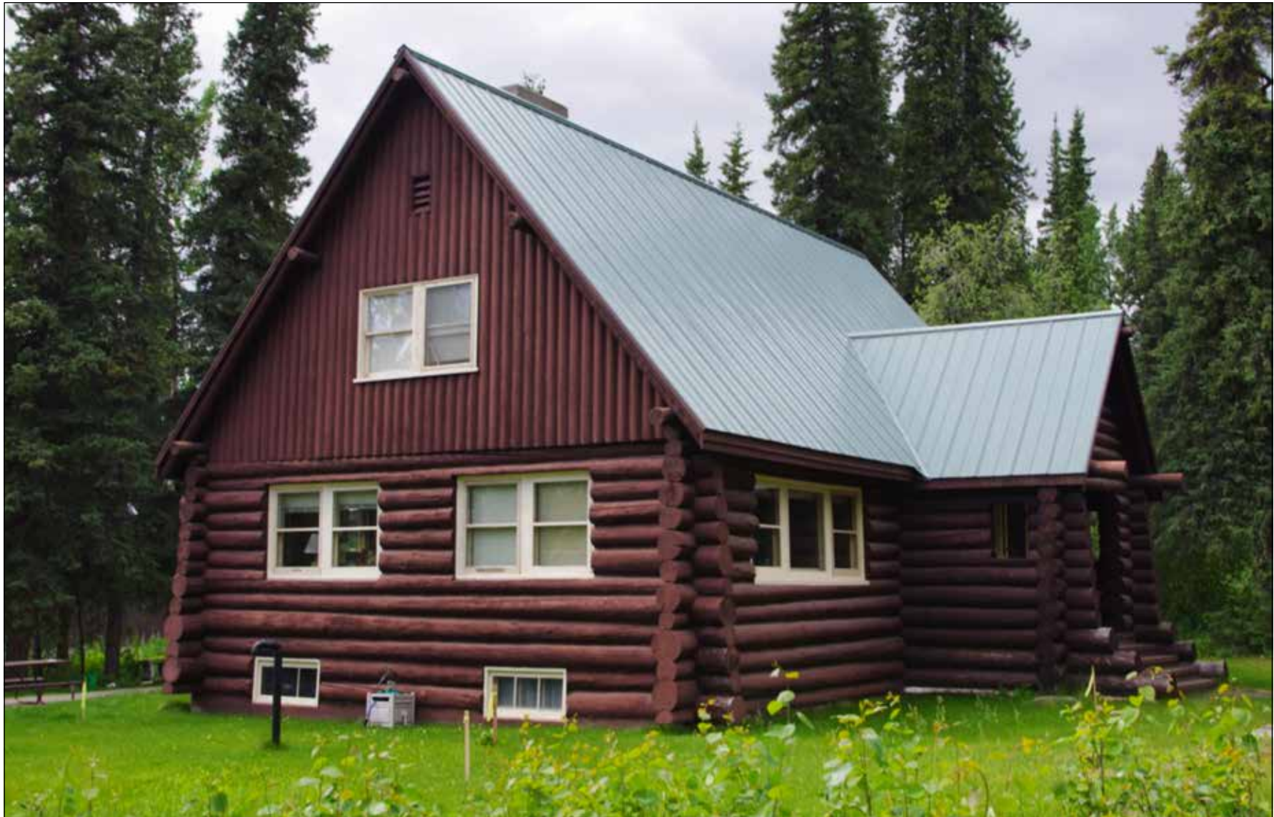
Figure 36. Building 23, view to the east, 2014 (NPS Alaska Regional Office files)
