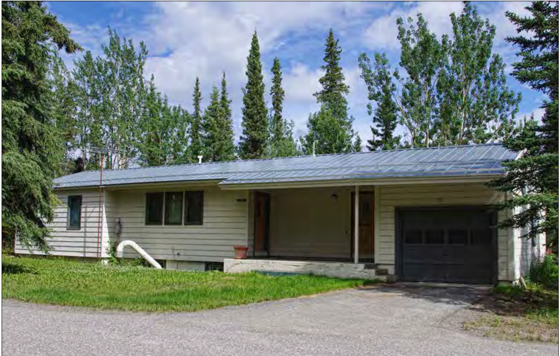
Figure 6. Building 27, view to the northeast, 2014 (NPS Alaska Regional Office Files)
