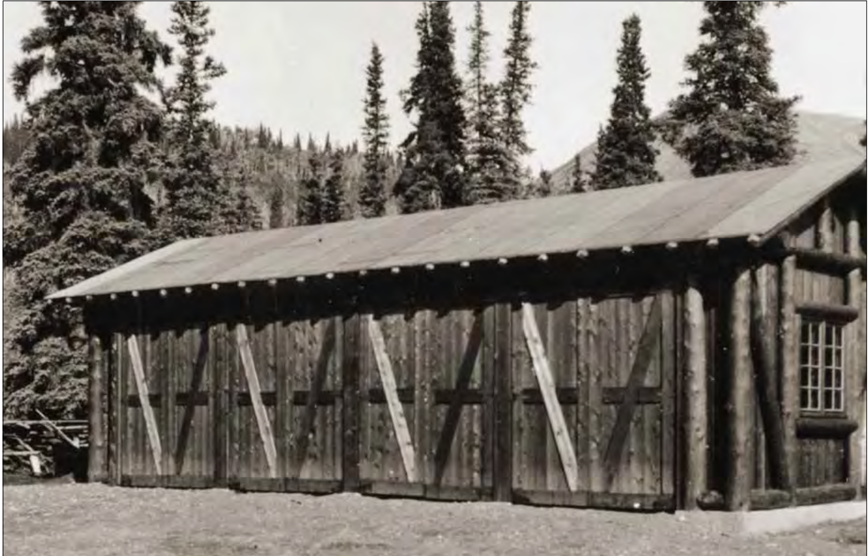
Figure 44. Building 103 (Garage), view to the northwest, Catalog No. DENA 21931, 1937 (Denali National Park and Preserve Museum Collection Archives)
