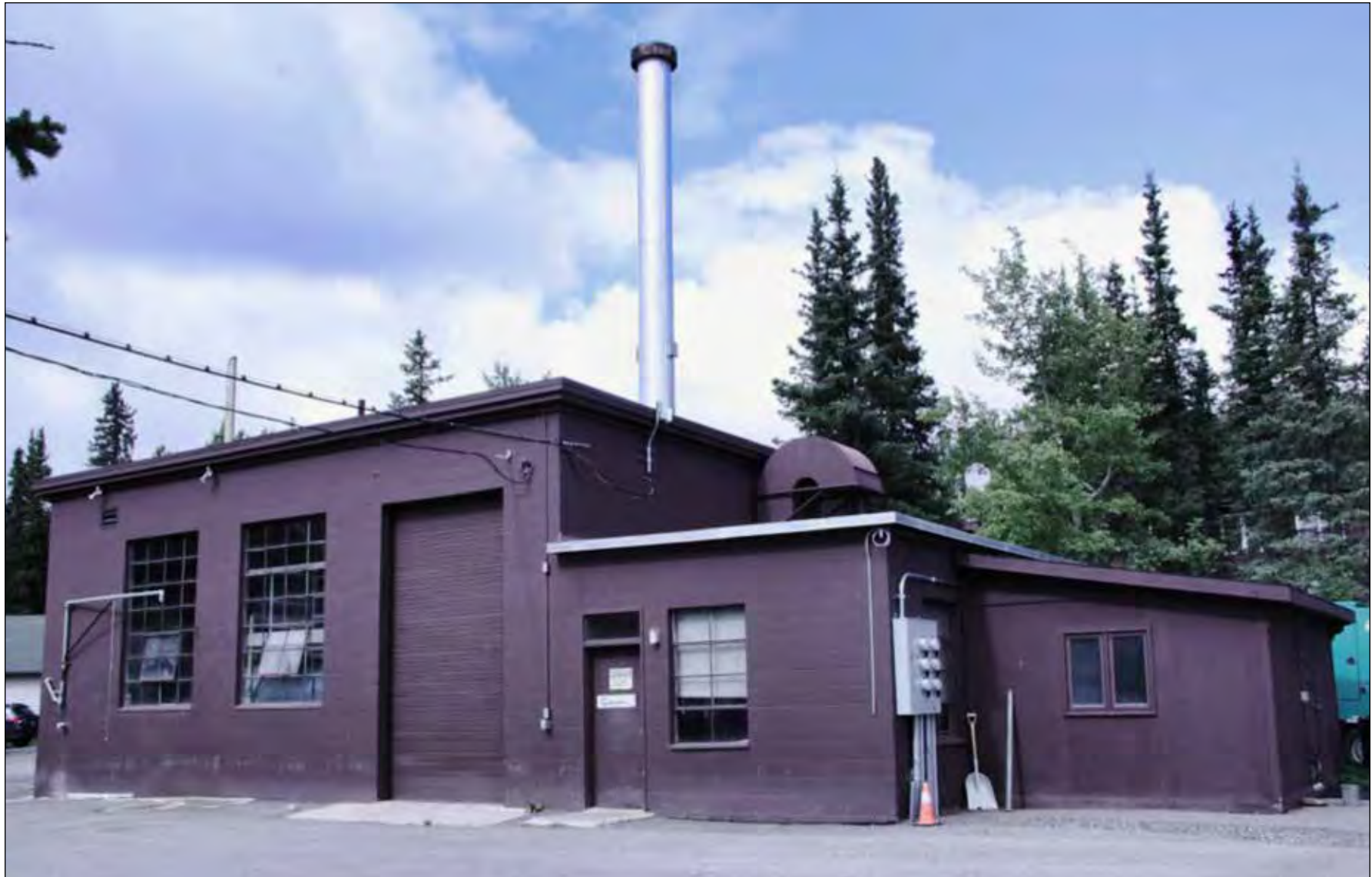
Figure 18. Building 54, North Elevation, 2011, AKRO Files
