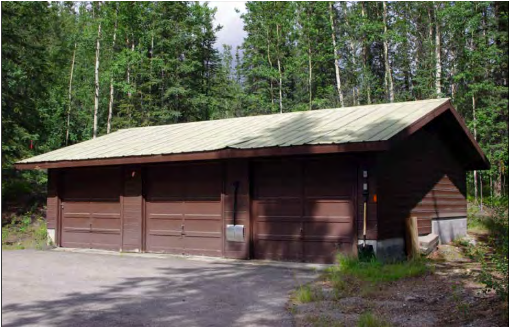
Figure 21. Building 217, South Elevation, 2014, AKRO Files
