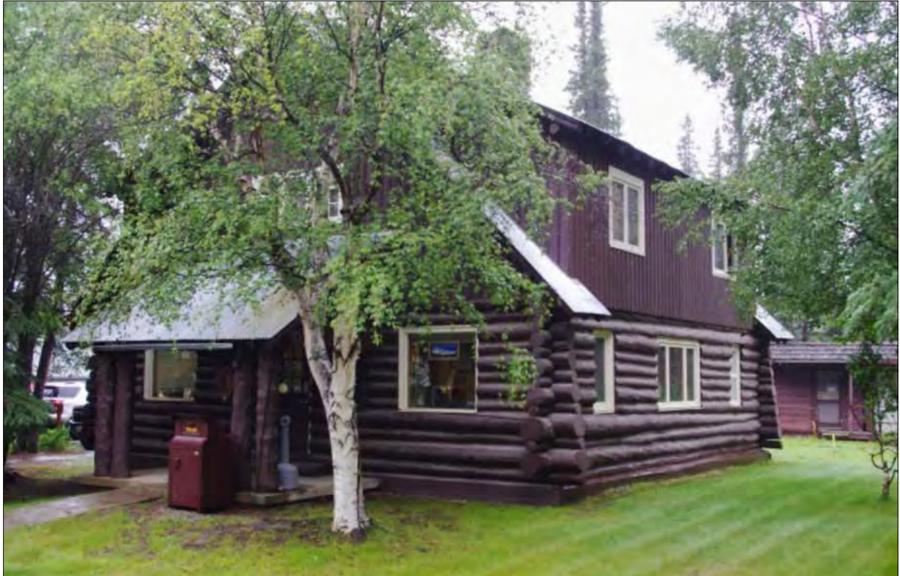
Figure 30. Building 21, view to the southwest, 2014 (NPS Alaska Regional Office files)
