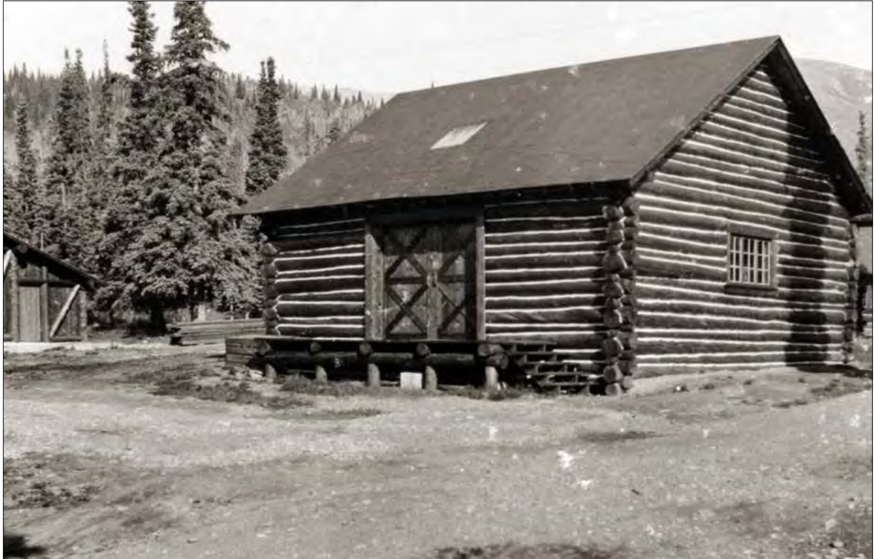
Figure 38. Building 101 (Warehouse), to the northwest, Catalog No. DENA 21198, 1932 (Denali National Park and Preserve Museum Collection Archives)
