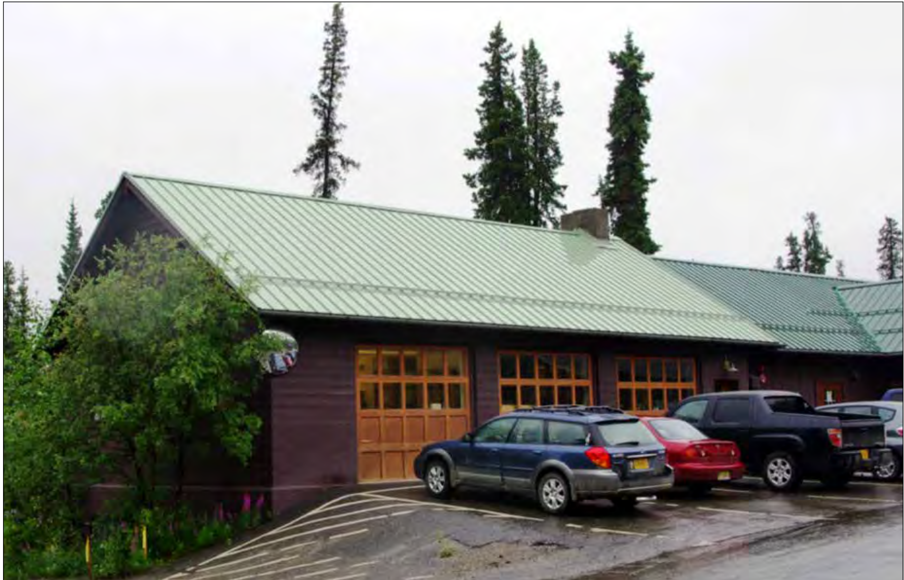
Figure 42. Building 102, view to the southwest, 2014 (NPS Alaska Regional Office Files)
