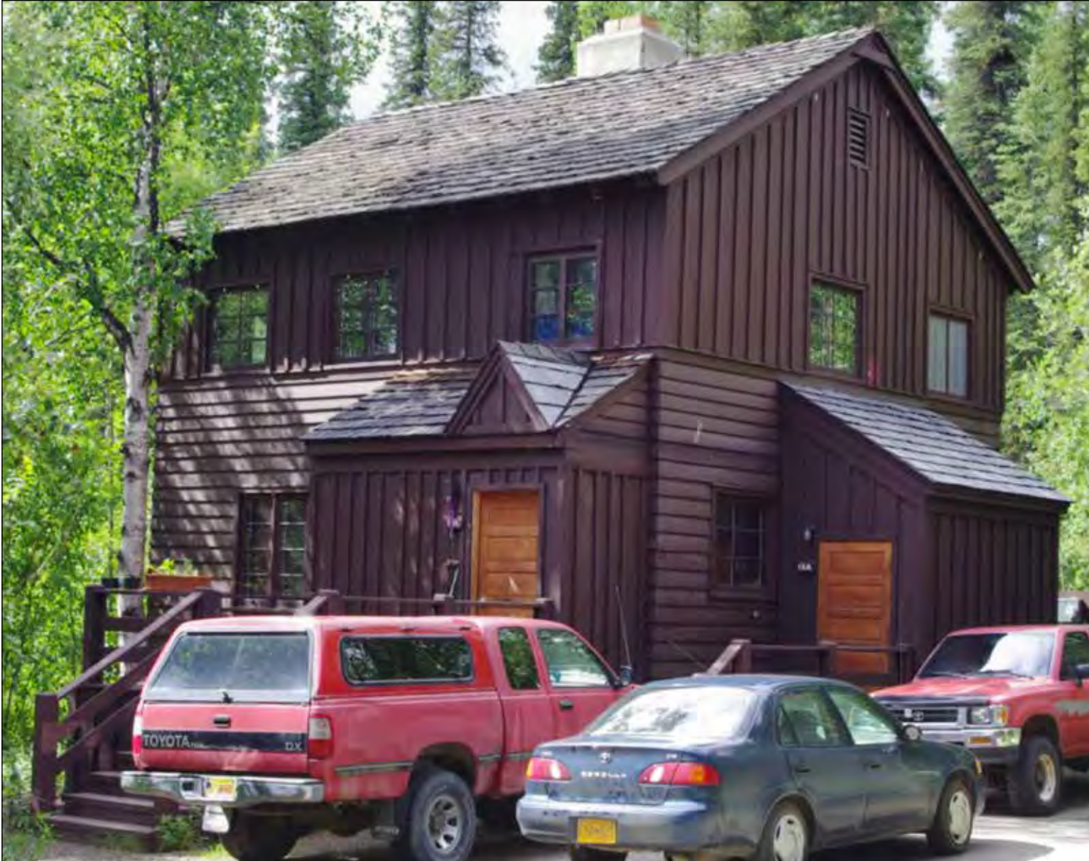
Figure 27. Building 13, view to the southwest, 2014 (NPS Alaska Regional Office files)
