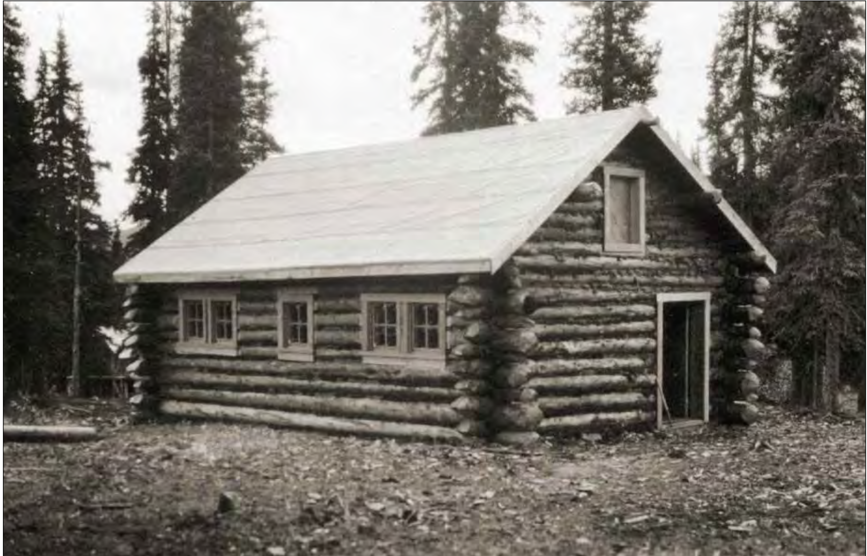
Figure 55. View southeast of the barn (Building 106), prior to 1931 (DENA 3974, Denali National Park and Preserve)
