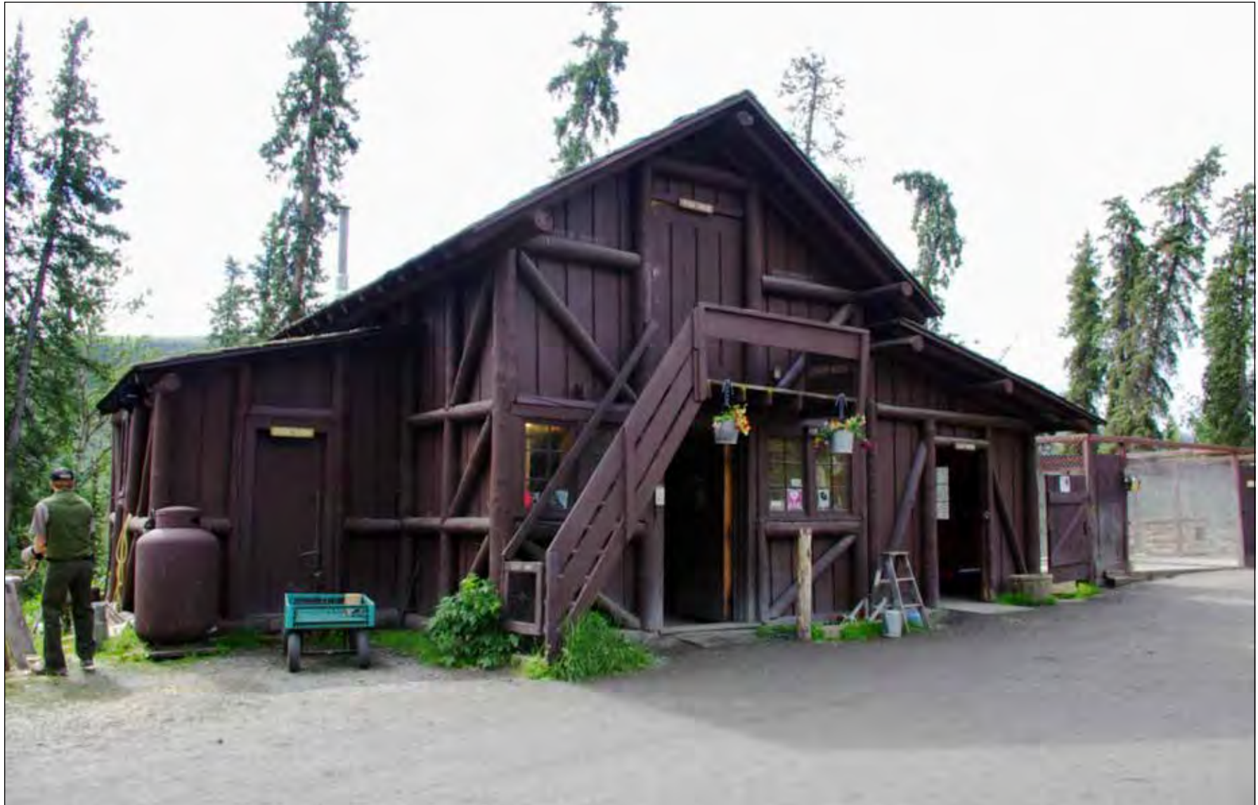
Figure 48. Building 105, view to the southwest, 2014 (NPS Alaska Regional Office Files)
