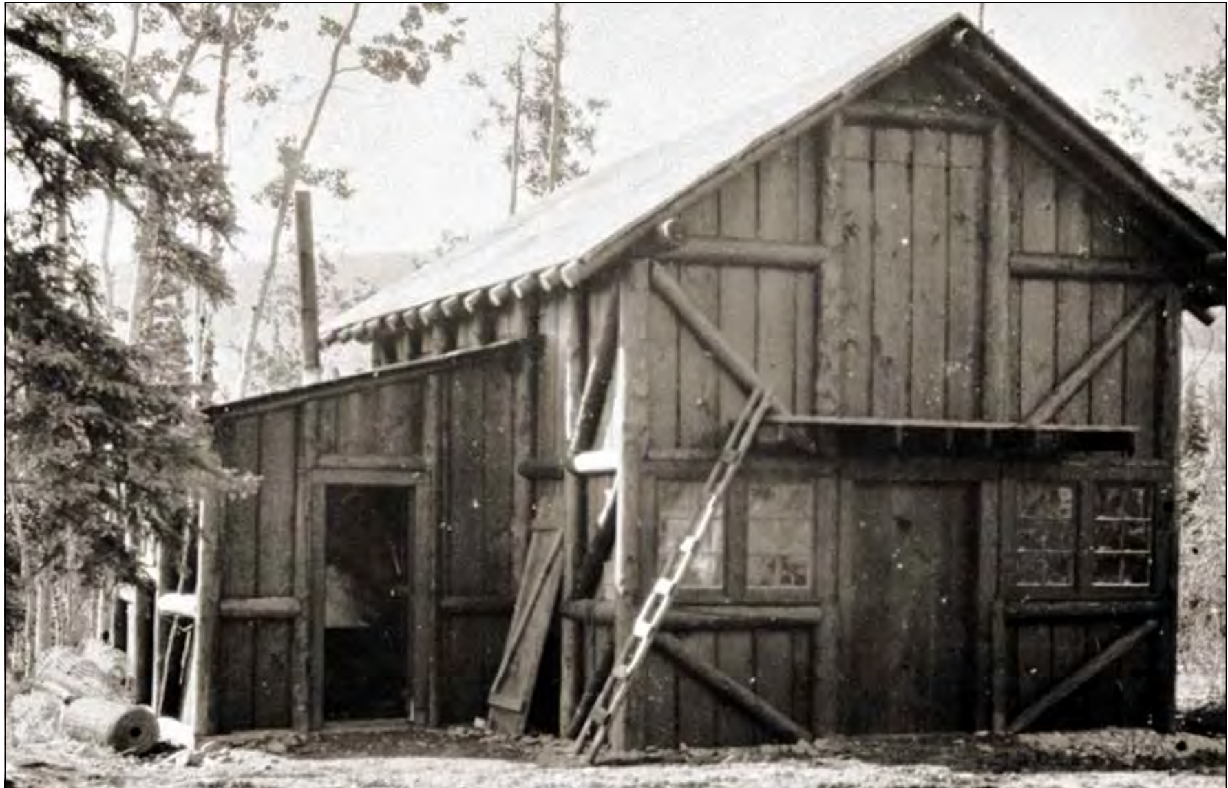
Figure 47. Building 105 (Dog Feed Cache and Sled Storage), view to the southwest, Catalog No. DENA 4323, n.d. (Denali National Park and Preserve Museum Collection Archives)
