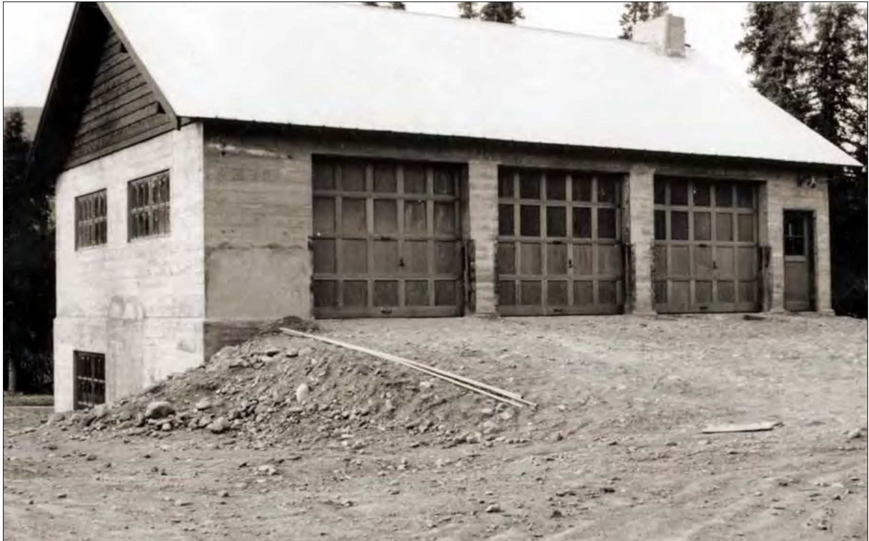
Figure 41. Building 102 (Garage and Repair Shop), view to the southwest, Catalog No. DENA 21158, 1939 (Denali National Park and Preserve Museum Collection Archives)
