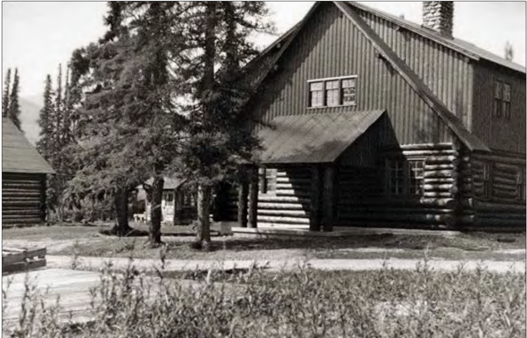
Figure 29. Building 21 (Ranger's Dormitory), view to the southwest, (Denali National Park and Preserve Museum Collection Archives)
