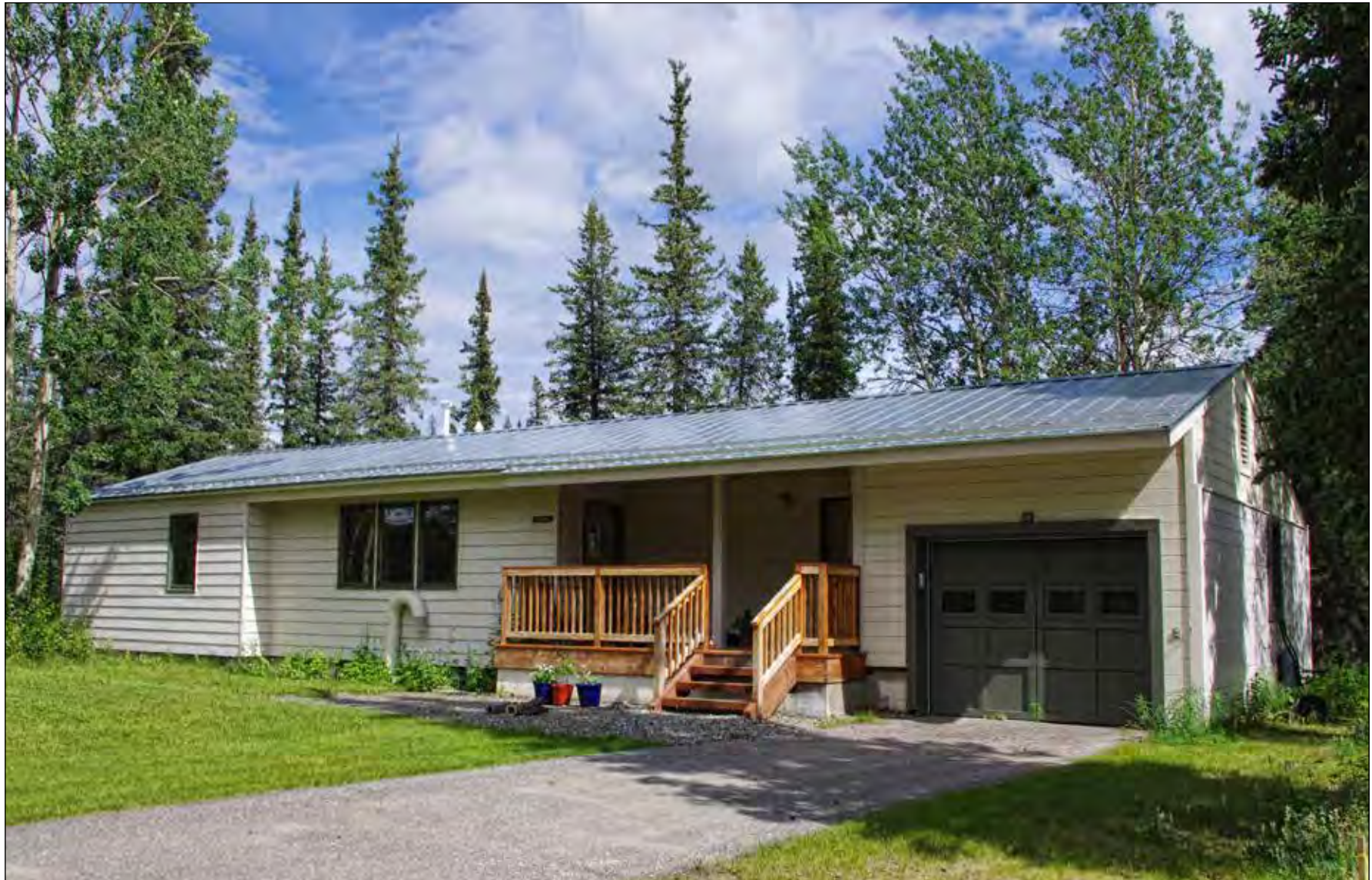
Figure 9. Building 28, view to the northeast, 2014 (NPS Alaska Regional Office Files)
