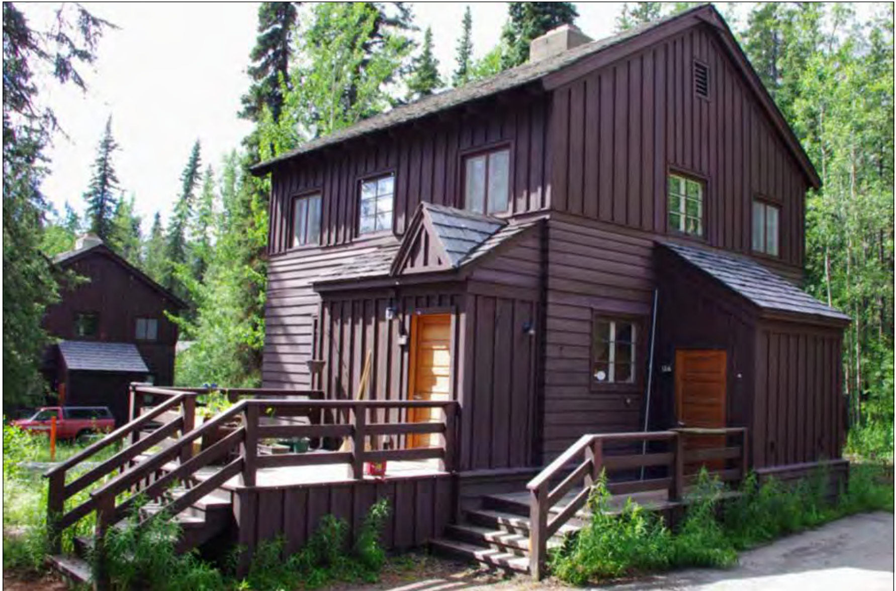
Figure 24. Building 12, view to the southwest, 2014 (NPS Alaska Regional Office files)
