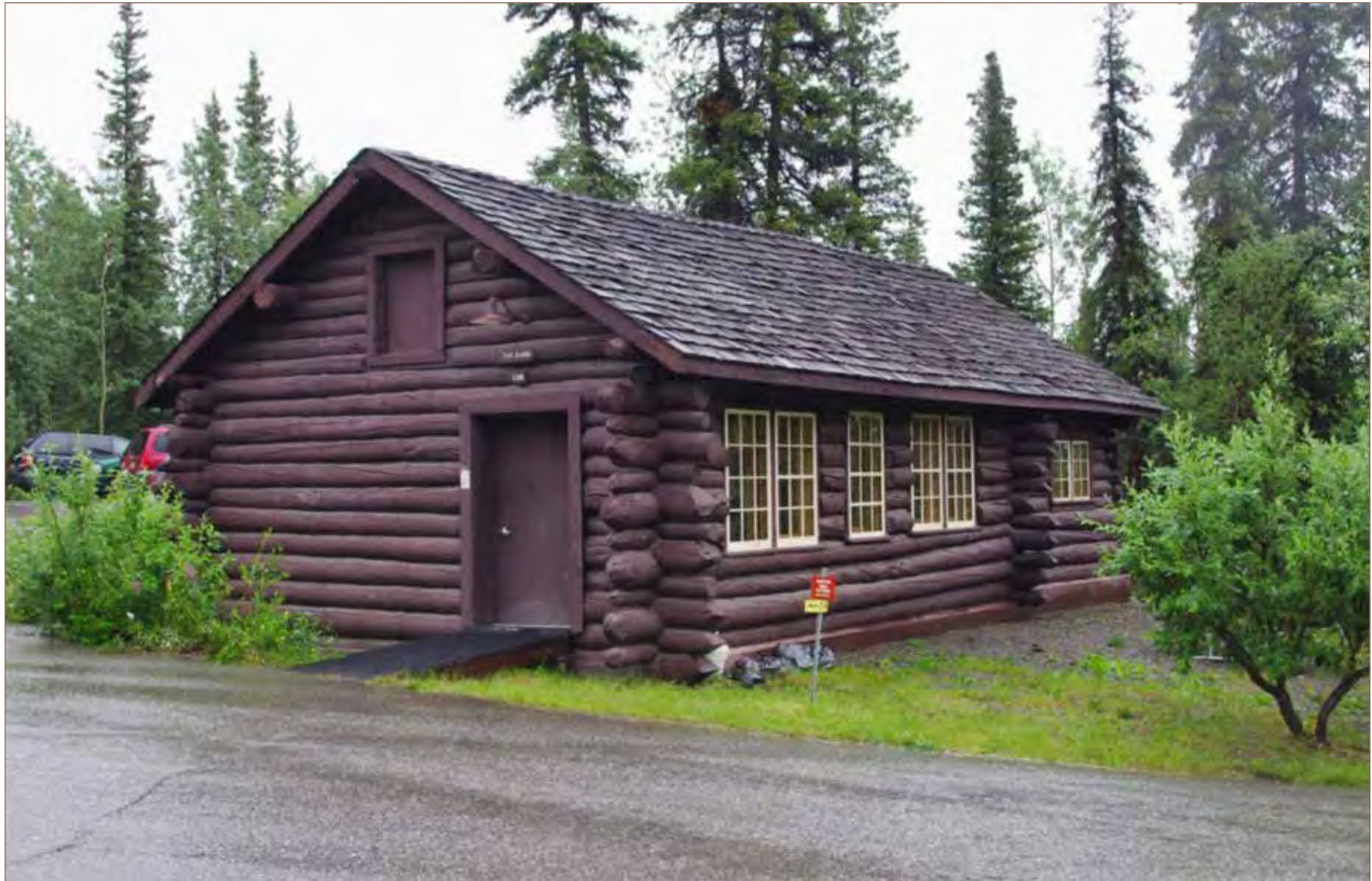
Figure 56. Building 106, view to the northeast, 2014 (NPS Alaska Regional Office Files)
