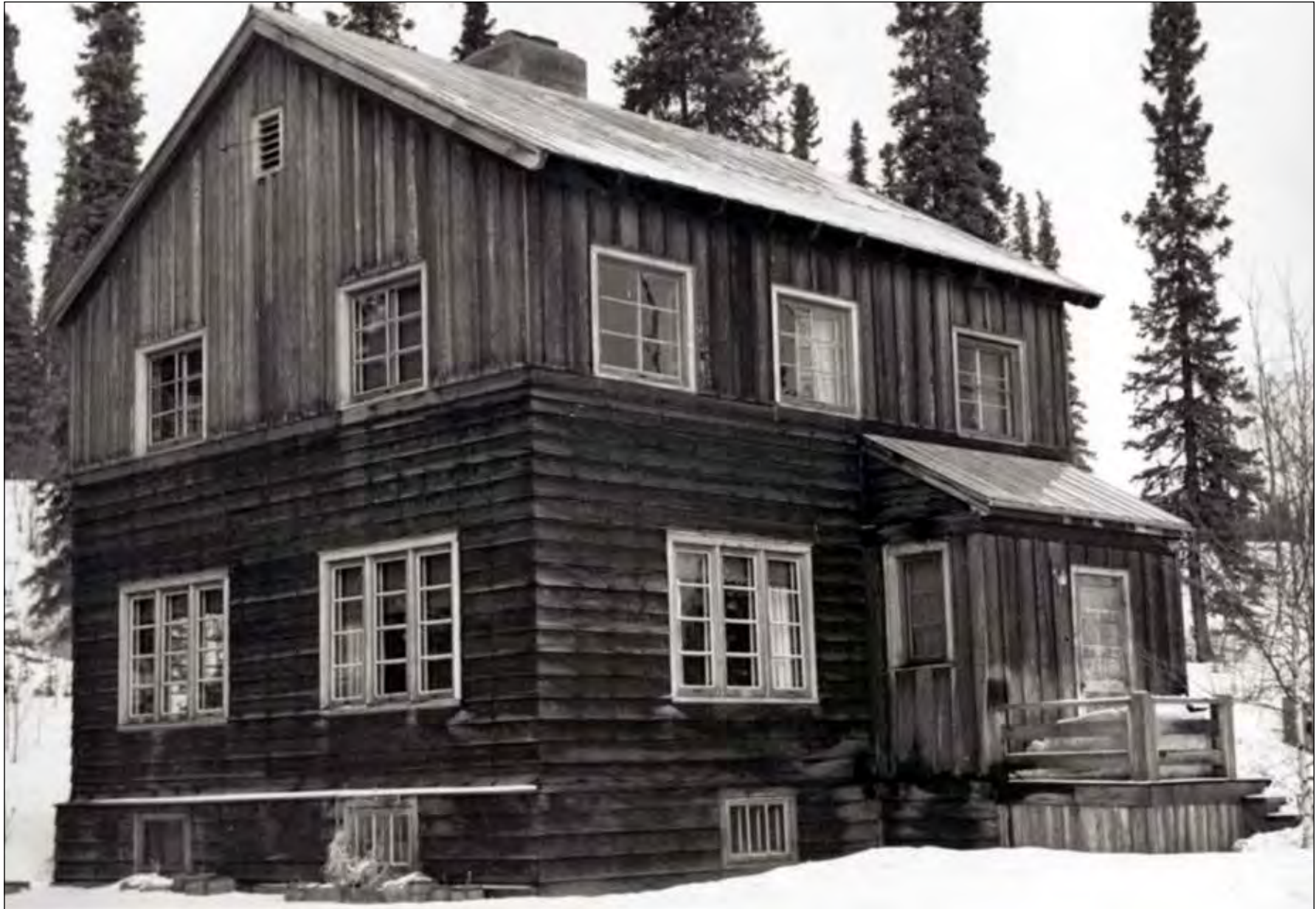
Figure 23. Building 12 (Employee Residence – Apartments), view to the southwest, Catalog No. DENA 9101.12.6, 1951 (Denali National Park and Preserve Museum Collection Archives)
