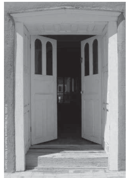
The painted wooden trim around windows and doors in Casa San Ysidro is part of the Territorial building style.
