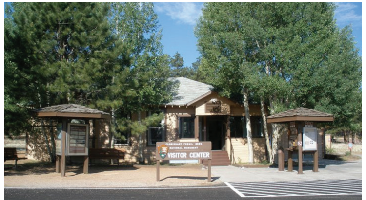
The original visitor center at Florissant Fossil Beds National Monument was previously part of the Baker property. The current Visitor Center and Paleontology Lab was built on the same footprint in 2013.
