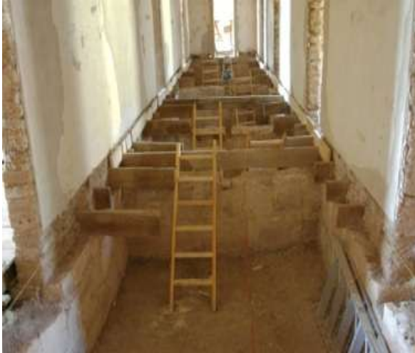
Post Hospital Restoration
