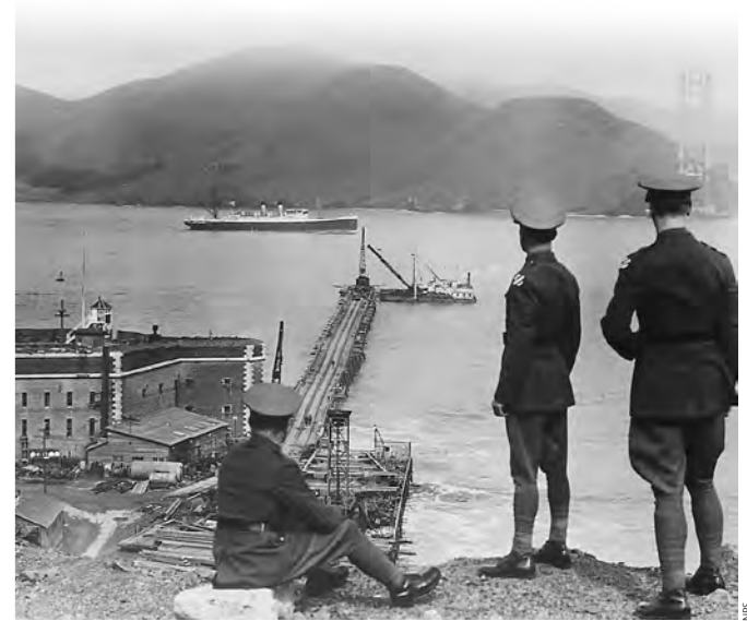
Golden Gate Bridge tower foundation construction, 1933.
