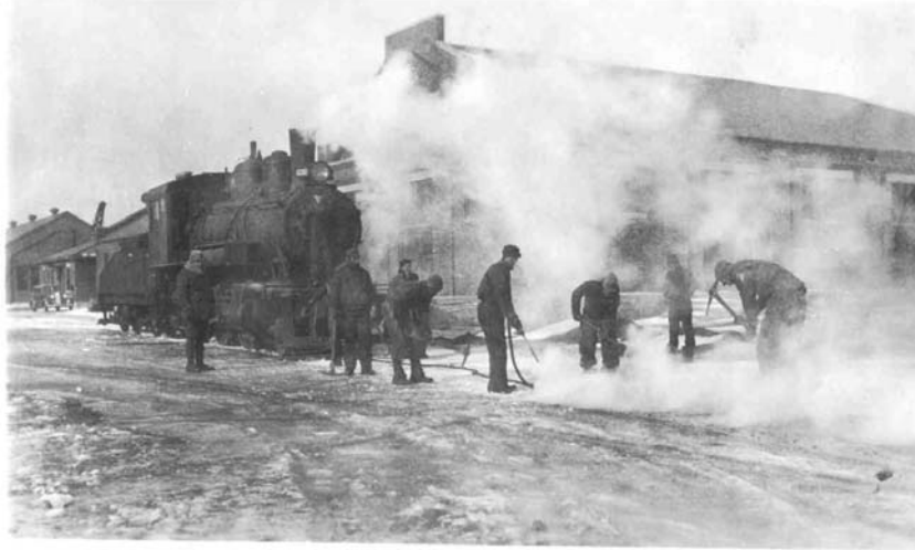
Steam pipe being used off railroad engine to de-ice the tracks. Photo is taken in the former Proving Ground Shop area.
