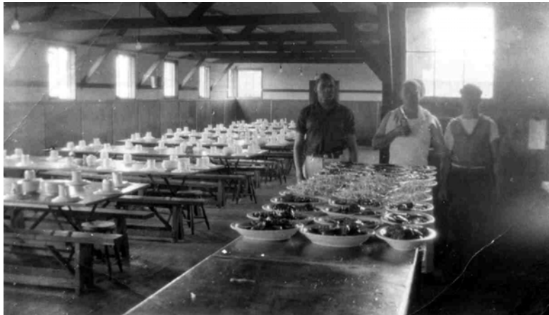
Mess hall at CCC Camp Lowe.
