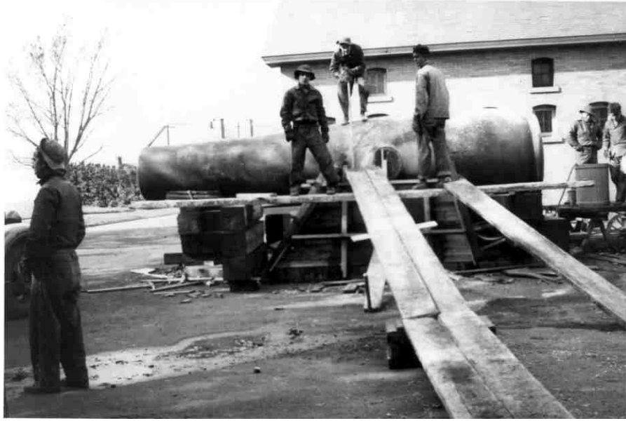
CCC Crew moving 20-inch Rodman gun to its current location. They also constructed the base it sits on.
