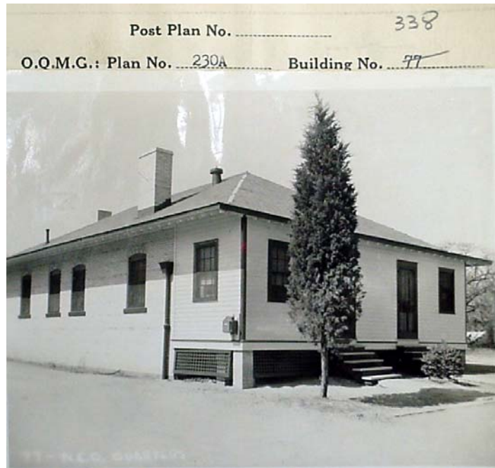
Building 338 where Mr. Mulhern's family lived from 1908-1927 Images Courtesy of NPS/Gateway NRA
