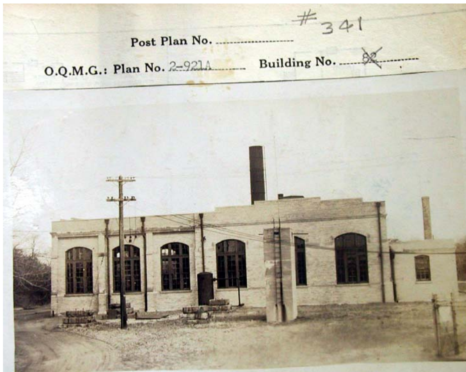
Fort Hancock Post Record Book image of Water Treatment Plant circa 1940.
