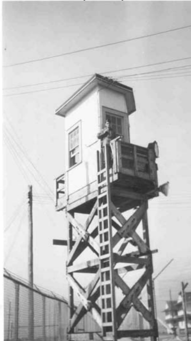
Guard watchtower at U.S. Disciplinary Barracks, Fort Hancock.
