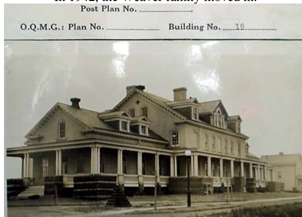
Fort Hancock Post Hospital in 1940.
