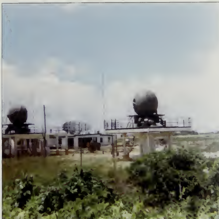
Figure 4.18. View looking west at target tracking radars (417 and 473), Control Area #1, NIKE radar site, circa 1962. A combination of bare sand and grass species was typical around the buildings and structures at the radar site. The vegetation in the foreground is in front of the perimeter fence and therefore outside the radar site (GATE 22043).
