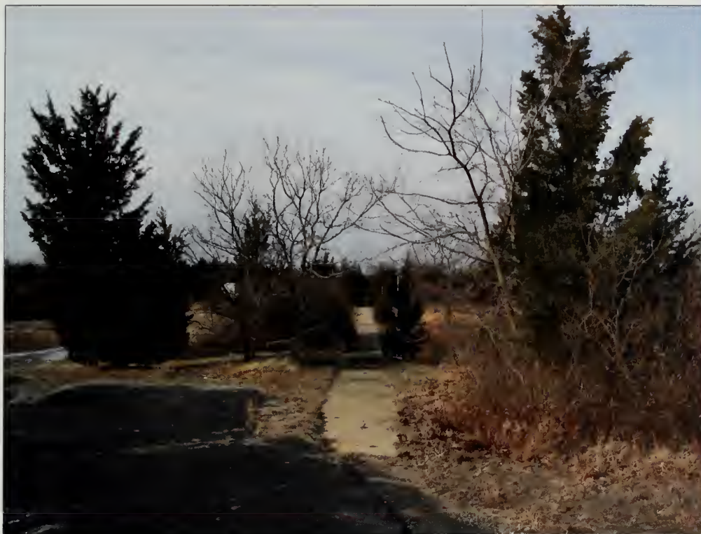
Figure 5.104. View looking north of sidewalk from Control Area #2 to the Ready Barracks, NIKE radar site. Asphalt, concrete, and gravel-surfaced circulation features should be cleared of woody vegetation six-feet off of all sides. Once woody vegetation, like the eastern red cedars seen in this photograph, has been removed, the six foot width can be easily maintained with a small tractor and brush hog mowing deck (Olmsted Center, January 2009).
