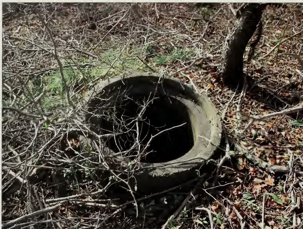
Figure 5.93. Concrete pipe on southern slope of Battery Mills. The concrete pipe should be capped to prevent possible injury and reduce water entering into or around the underground structures (Olmsted Center, January 2009).
