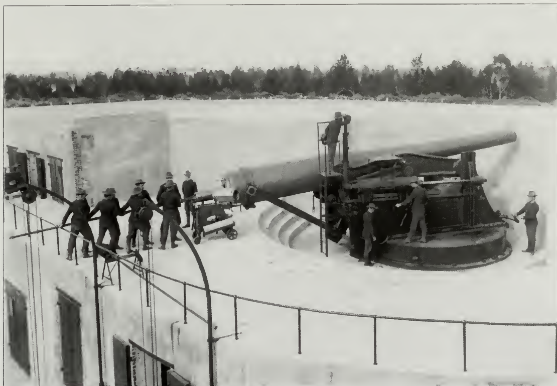
Figure 5.63. Battery Granger, circa 1900. Note the growth of woody vegetation beyond the limits of the engineered slopes. Great effort was made to disturb as little pre-existing vegetation in front of the battery as possible in order to conceal the structure from enemy fire (GATE 7778).
