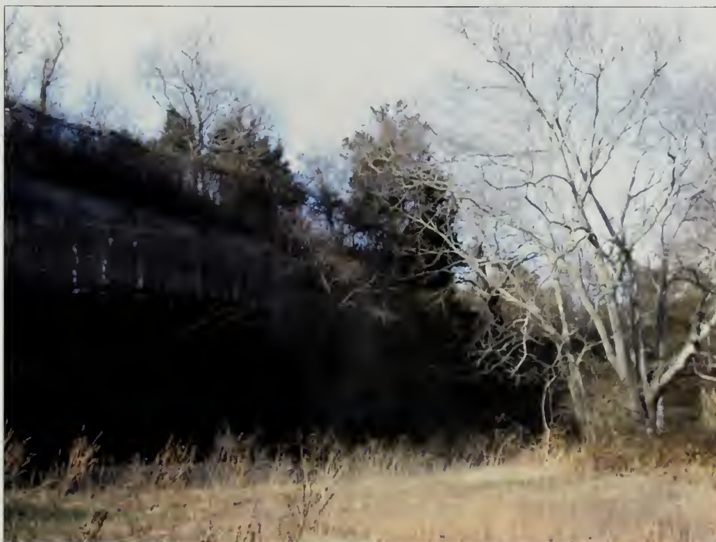
Figure 5.84. View looking northwest at the south gun emplacement, Battery Kingman. Vegetation removal to restore the historic field of fire should focus on the slopes against the battery's concrete facades as the level area in front of the guns is relatively free of tree and shrub vegetation (Olmsted Center, January 2009).
