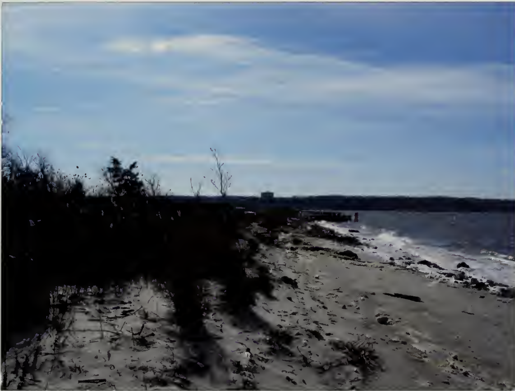
Figure 3.45. View looking south at eroded vehicular route, Battery Mills. On the west side of Battery Mills a portion of the road encircling the battery, approximately 200-feet, has been washed away by Sandy Hook Bay (Olmsted Center, January 2009).
