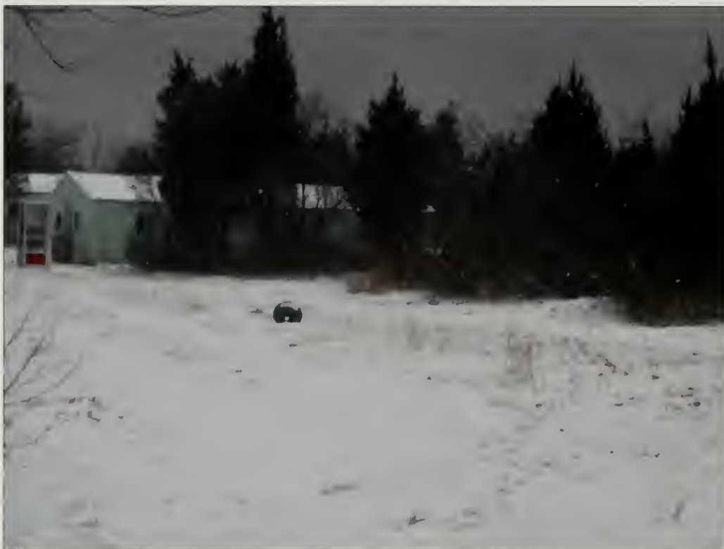
Figure 5.111. Existing light fixture between building 404 and 405, NIKE radar site. The fallen fixture should be reset and will most likely require a new concrete footing and tubular pole. The new pole should match the existing in material, dimensions, and finishing. The fixture's other components should be inspected at this time and repaired or replaced based on their condition (Olmsted Center, January 2009).
