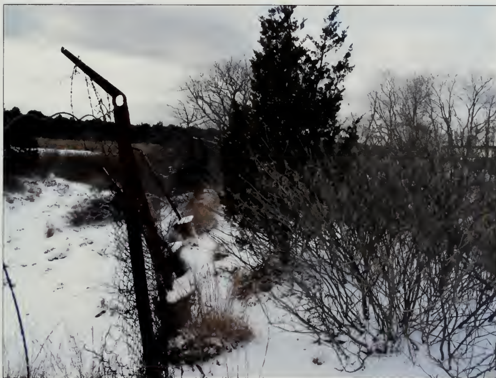
Figure 5.105. Existing perimeter fence, NIKE launch site. The existing perimeter fence at the radar and launch sites should be clearly delineated and maintained by removing all woody vegetation a minimum of four-feet off either side of the fence. The vegetation removals will also aid in inspection and repairs of the existing fence (Olmsted Center, January 2009).
