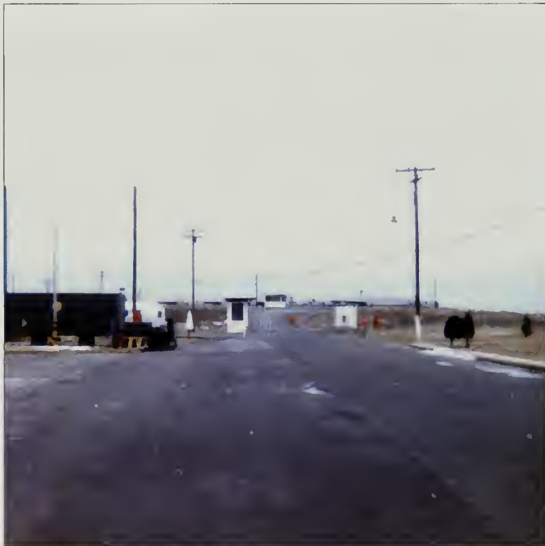
Figure 4.21. View looking east at the Missile Magazines and Missile Maintenance Area, circa 1958. The access road to the Missile Magazines and Missile Maintenance Area was paved with asphalt as part of alterations to the launch site for the Hercules missile. The road is presently extant and in good condition (GATE 22042).
