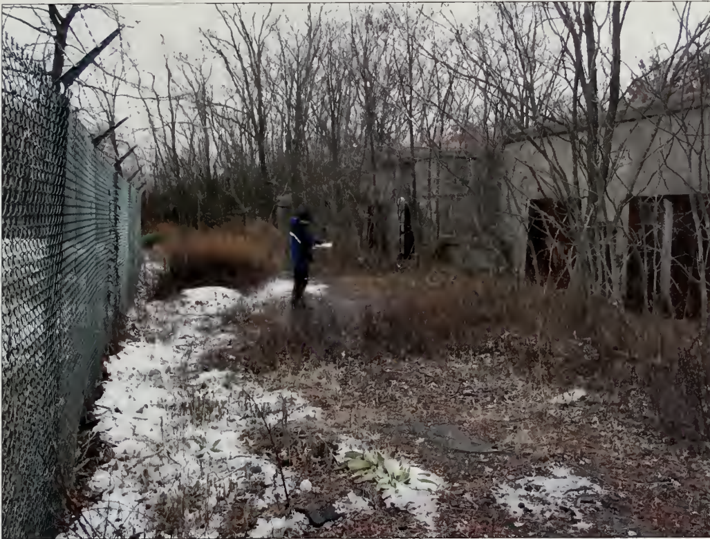
Figure 3.5. View looking west at U.S. Coast Guard perimeter fence and Battery Morris. There is currently no vehicular access to Battery Morris and staff and visitors wishing to see the structure walk on a trail surface comprised of broken asphalt and accumulated leaf litter and debris. Emerging woody vegetation obscures a clear definition of the trail and makes access difficult (Olmsted Center, January 2009).
