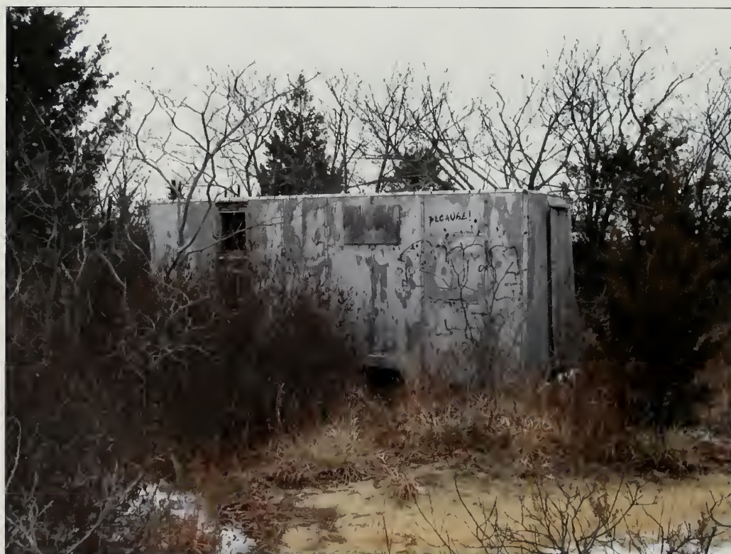
Figure 3.12. View looking north at a post World War II trailer, Batteries Engle and Peck. Northeast of Battery Engle, a communications trailer sits abandoned. The trailer is a frequent target for graffiti (Olmsted Center, January 2009).
