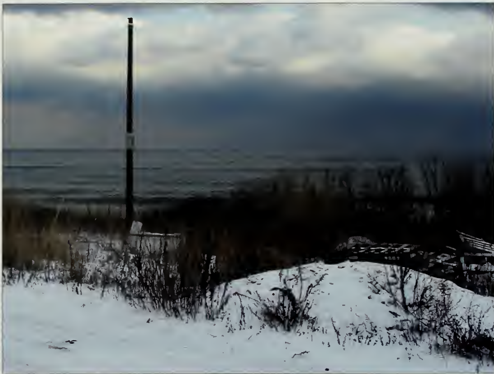
Figure 5.102. View looking northeast at CODAR antenna, NIKE launch site. The launch site has become home to a variety of uses for other institutions. An antenna and monitoring equipment have been set up for collecting weather and tide information. A pile of shells and palettes on the right are for a shellfish seeding program (Olmsted Center, January 2009).
