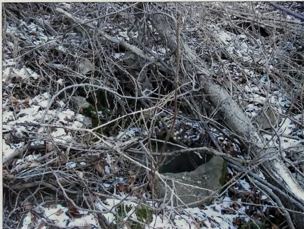
Figure 5.86. Concrete pipe on north slope of Battery Kingman. The concrete pipe should be capped to prevent possible injury and reduce water entering into or around the underground structures (Olmsted Center, January 2009).
