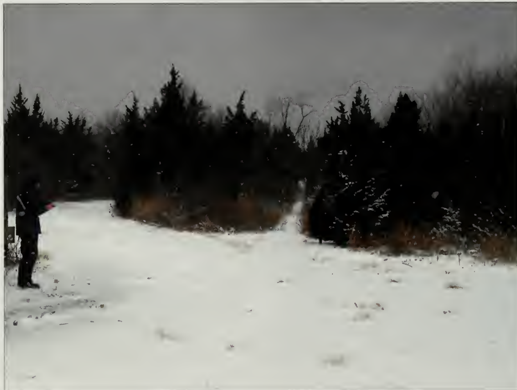
Figure 4.17. View looking northwest at pedestrian walkway, Control Area #1, NIKE radar site. The concrete walkways connecting the control areas and Ready Barracks are presently extant and in fair condition. Some portions of the sidewalks are being covered by encroaching woody vegetation (Olmsted Center, January 2009).
