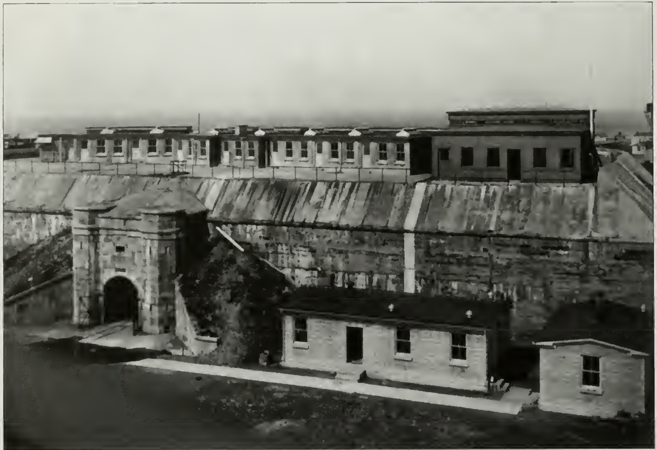
Figure 2.30. West facade of Battery Potter showing switchboard rooms, circa 1907. In order to support the communications between the fire control buildings and various batteries, the Army built two switchboard rooms at the southwest corner of Battery Potter in 1907. The two buildings required further removal of the engineered earthwork along the battery's west facade (GATE 7814).
