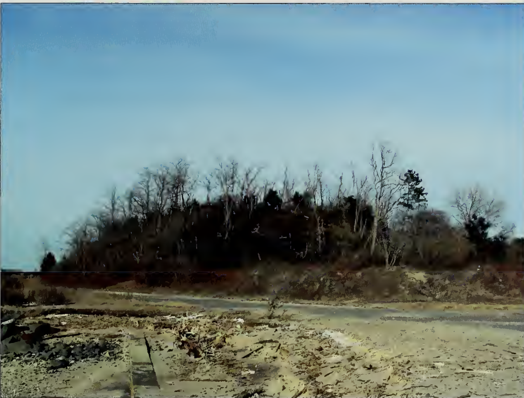
Figure 3.46. View looking northeast at Battery Kingman. The major constructed feature of Batteries Kingman and Mills is the engineered earthwork that rises in stark contrast to the surrounding land (Olmsted Center, January 2009).
