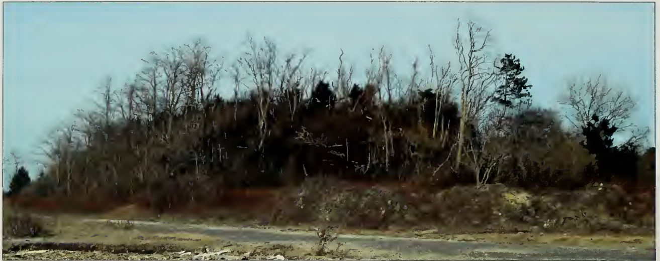
Figure 5.81. View looking northeast at the Battery Kingman engineered landform. This photograph shows the size and quantity of woody vegetation growing on Battery Kingman's engineered slope. All woody vegetation greater than four-inches diameter at breast height should be selectively removed to preserve the historic structure and its sheltering earthwork (Olmsted Center, January 2009).
