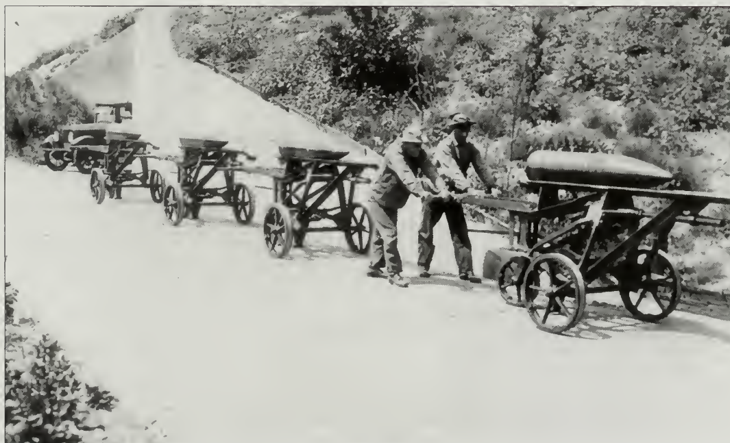
Figure 2.42. View of concrete route to emplacement #1, Battery Kingman, circa 1920s. Soldiers retrieved shells and gunpowder from the casemated storage areas (background) and transported them on hand carts to either circular gun platform (GATE 17820).
