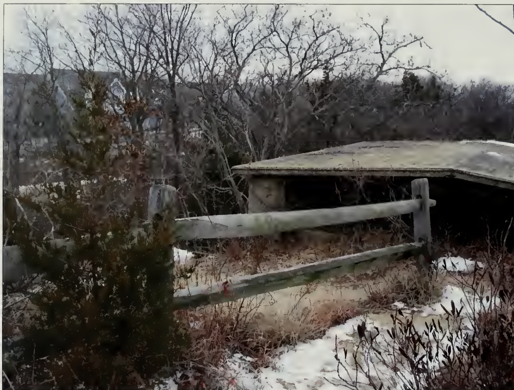
Figure 3.11. View looking northwest at Battery Engle (CRF Station Peck). The concrete coincidence range finder station (CRF) constructed on top of Battery Engle is located west of Battery Peck and features a low-pitched concrete roof. The structure appears in fair condition with some minor efflorescence visible on the roof (Olmsted Center, January 2009).
