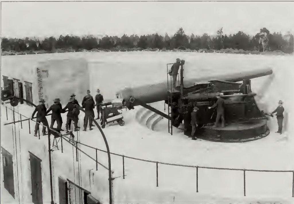
Figure 4.10. View looking northeast at emplacement #1, Battery Granger, 1899. A raised platform on the gun carriage allowed an artillery officer views over the concrete structure to a potential target. Although the gun carriages are not extant, views from a comparable vantage point and from the battery commander's stations are presently obstructed by large woody vegetation (GATE 7778).
