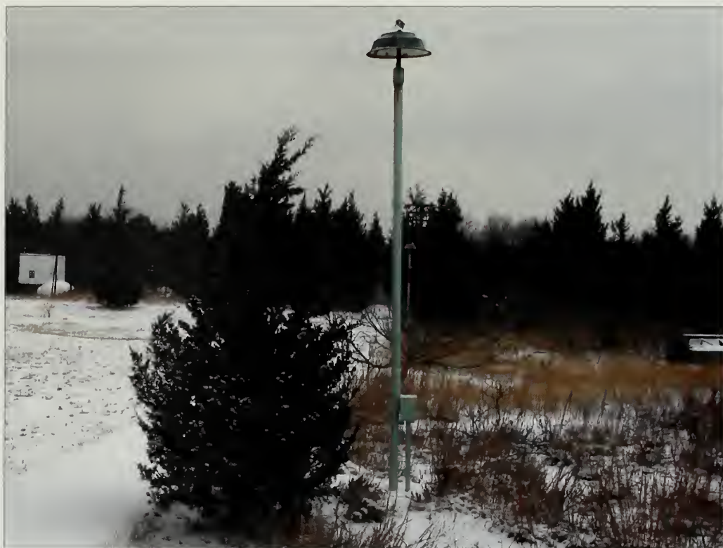
Figure 5.110. Existing light fixture, NIKE radar site. The historic light fixtures should be periodically inspected, have components repaired or replaced as needed, and receive corrosion treatment, priming, and painting to match the historic finish. The eastern red cedar in the foreground should be removed as part of vegetation management along the circulation systems (Olmsted Center, January 2009).
