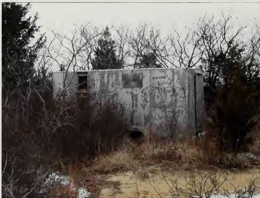
Figure 5.42. View looking north at a post World War II trailer located near Batteries Peck and Engle. The trailer is in a seriously deteriorated condition and, along with an accompanying section of fence, should be removed to improve the visual and spatial connection among Battery Peck's gun emplacements, commander station, CRF station, and the water in the distance (Olmsted Center, January 2009).
