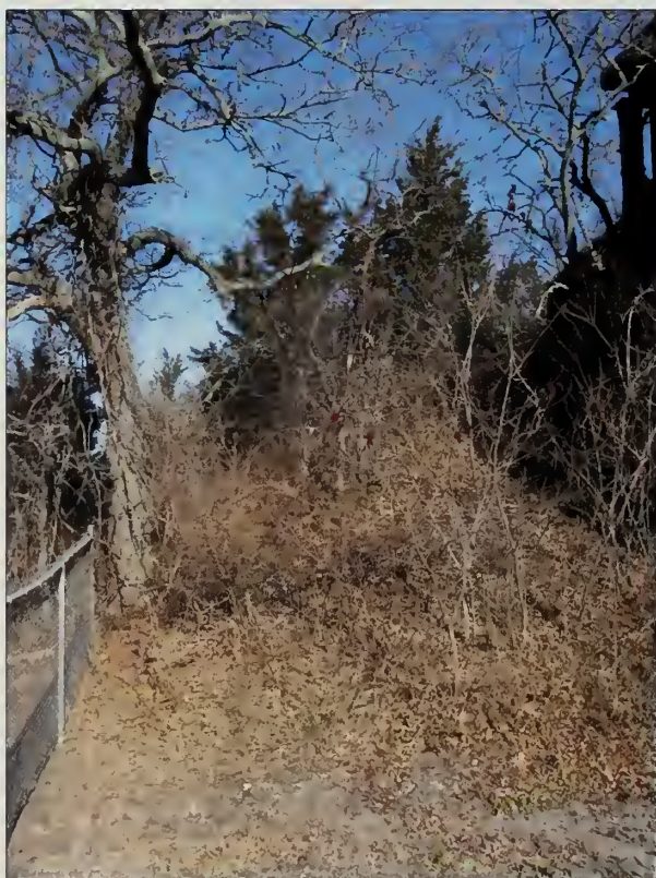
Figure 5.66. View looking northwest at engineered slope to rear of Battery Granger, host to large unmanaged woody vegetation (Olmsted Center, January 2009).
