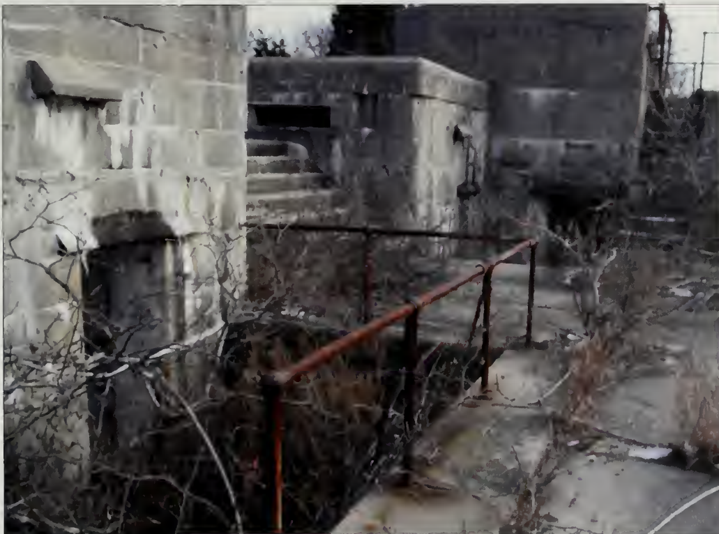
Figure 5.26. Existing historic safety railing at Battery Urmston is fabricated of pipe rail sections and ball joint connectors. After treating corrosion and restoring the historic finish, infill panels should be installed where there is a vertical change equal to or greater than thirty inches in order to provide greater safety at the large openings below the top rails (Olmsted Center, January 2009).
