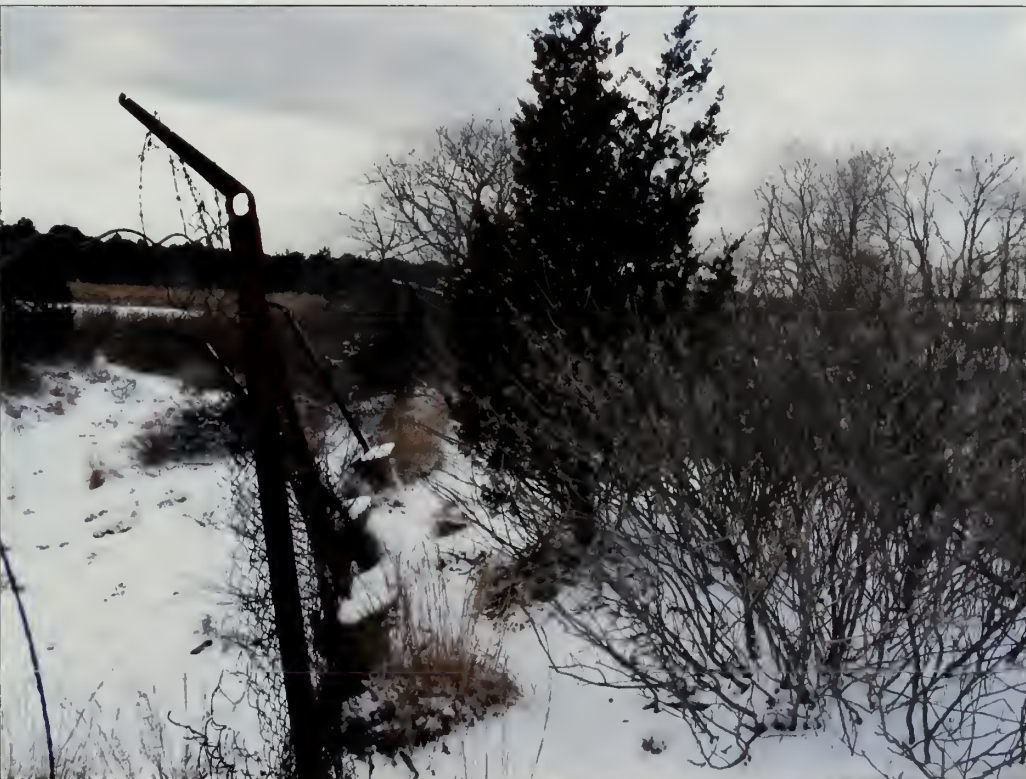
Figure 3.70. Outer fence, NIKE launch site. The inner and outer fences are comprised of chain-link sections secured to H-shaped posts. The top of each post holds a single extension arm that supports strands of barbed wire. This section of fence is in poor condition (Olmsted Center, January 2009).
