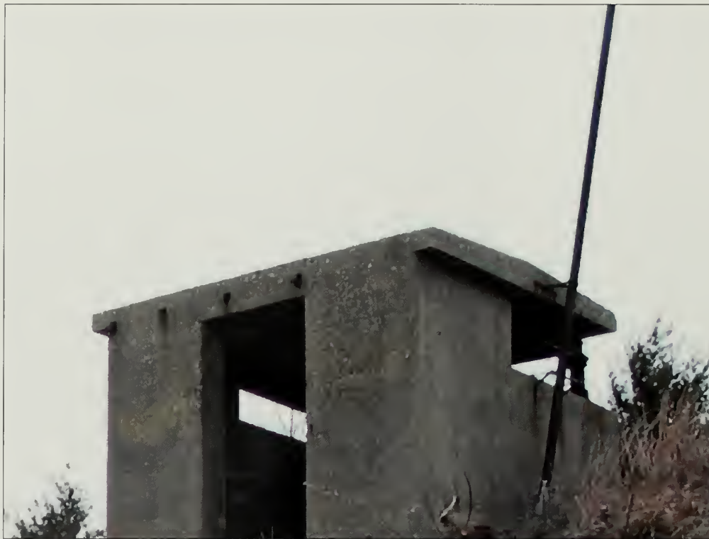
Figure 5.41. View of northwest facade of Battery Peck's commander station. The metal antenna and mounting brackets are features of this structure and should be preserved or replaced in kind. Measured drawings should be prepared to document these features followed by corrosion treatment, priming, and painting to match the historic finish (Olmsted Center, January 2009).
