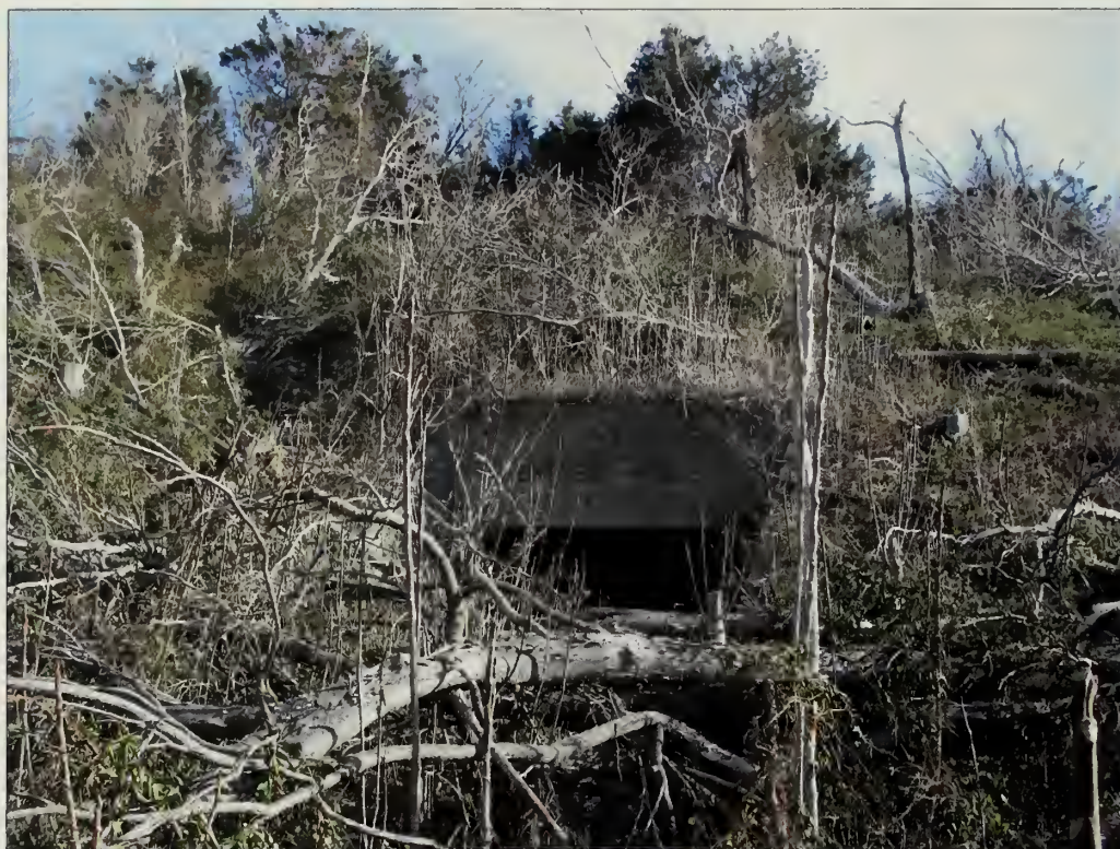
Figure 3.47. View looking east at entry to emplacement #1, Battery Mills. The main entry and entry for emplacement #1 are inaccessible due to the density of woody vegetation (Olmsted Center, January 2009).
