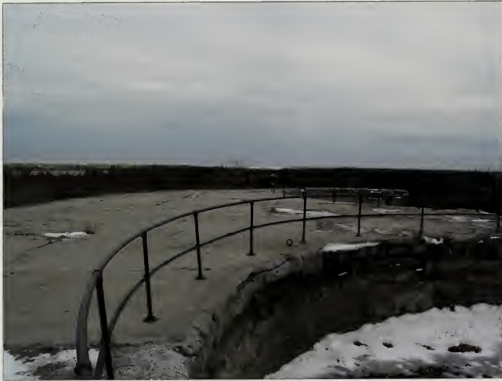
Figure 5.61. Recently installed contemporary safety railing, Battery Potter. Woven-wire may be either installed as infill panel, or the mesh applied with clamps to satisfy life-safety codes (Olmsted Center, January 2009).
