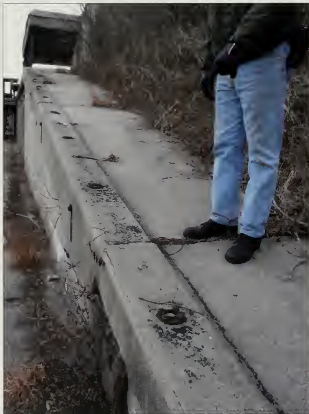
Figure 5.49. View looking northwest at the concrete ramp to gun platform #1, Nine Gun Battery. New safety railings should be installed on the ramp to facilitate visitor access. The rails should either attach to the existing escutcheon plates or be core drilled into the ramp's concrete structure. The new handrail components should match the original pipe railings and ball joint connectors at Nine Gun Battery to the greatest extent practicable (Olmsted Center, January 2009).
