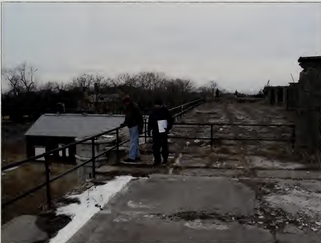
Figure 3.30. View looking north across terreplein, Battery Potter. As an additional safety measure, guardrails are installed on the western portion of the terreplein to prevent access to the sloped portion of the concrete structure (Olmsted Center, January 2009).
