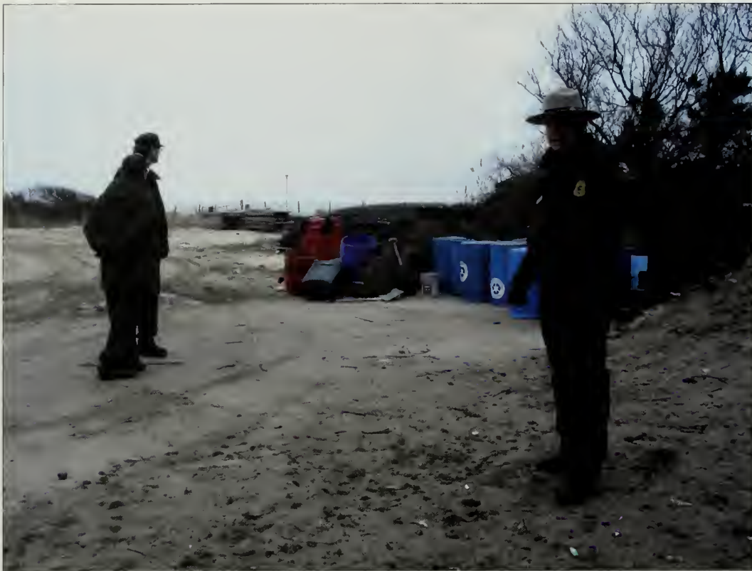
Figure 4.2. View looking east at the south earthwork, Missile Maintenance Area, NIKE launch site. The railroad tie retaining structure and recycling containers cut into a portion of the engineered earthwork (Olmsted Center, April 2008).
