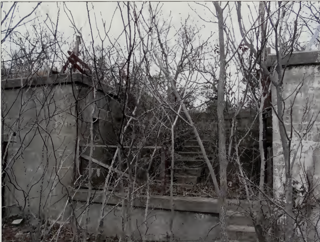
Figure 3.6. View looking north at emplacement #2, Battery Morris. Woody vegetation is growing in and around the stairs to the point where they are difficult to ascend and reach the gun platforms (Olmsted Center, January 2009).
