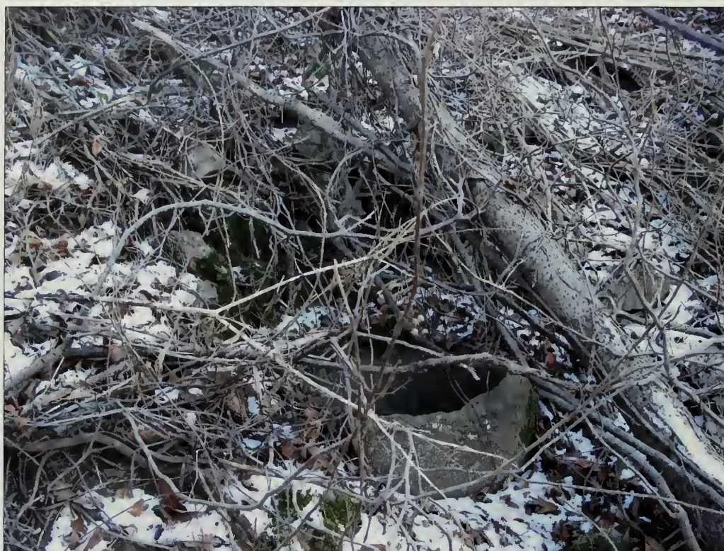
Figure 3.51. Concrete pipe, Battery Kingman. A concrete pipe protrudes through the engineered earthwork northwest of emplacement #2 (Olmsted Center, January 2009).
