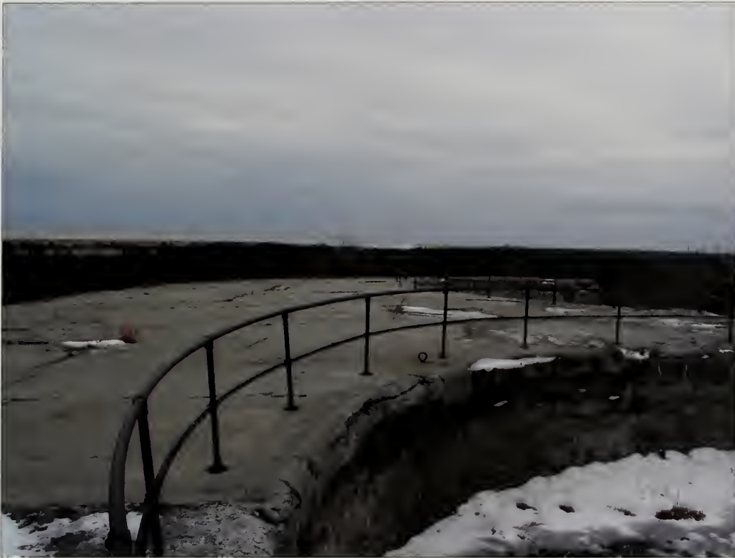
Figure 3.29. View looking south at guardrails, Battery Potter. To increase visitor safety, the National Park Service has recently added guardrails between the superior slope and the terreplein where the guns were emplaced (Olmsted Center, January 2009).
