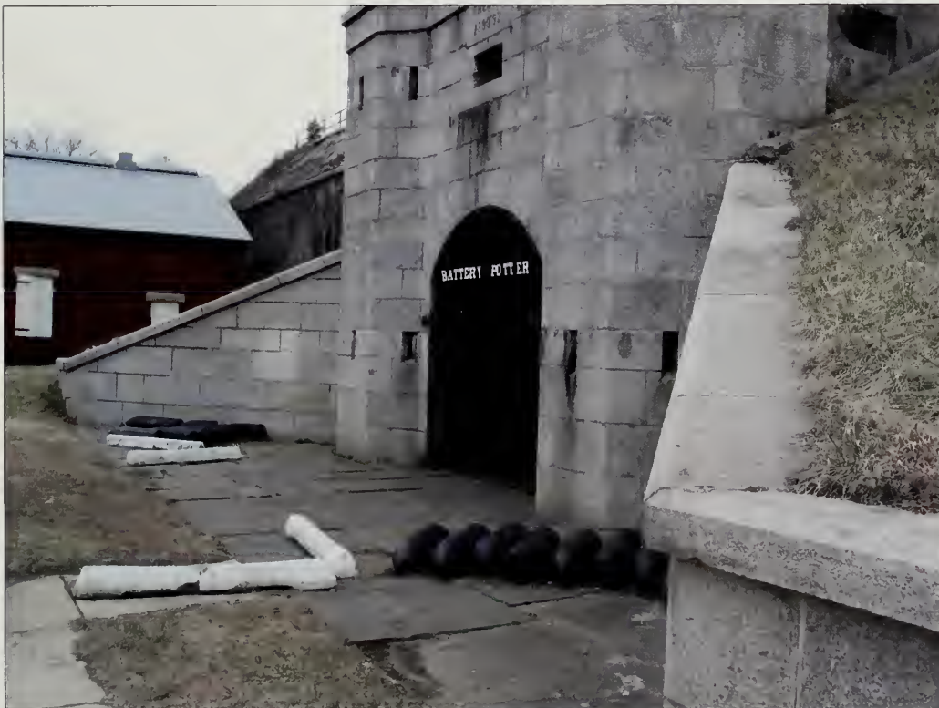
Figure 5.58. View looking north at defensible main entry, Battery Potter. The main entry is through an arched opening flanked by defensive stone towers. Each tower had gun loop slots so machine guns could fire on potential attackers. The entry facade resembles a castle and was constructed from granite blocks salvaged from Sandy Hook's Civil War-era fort (Olmsted Center, January 2009).
