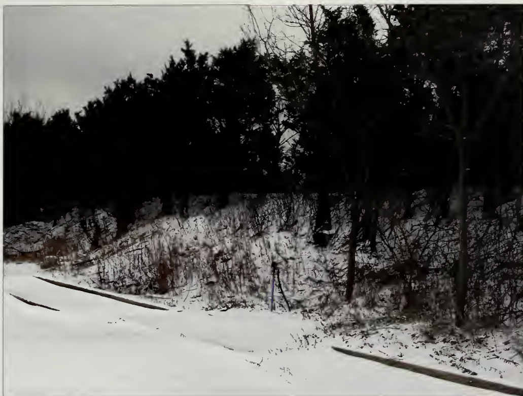
Figure 5.116. View looking southeast at Missile Maintenance Area historic earthwork, NIKE launch site. For the NIKE earthworks, all woody vegetation greater than four-inches diameter at breast height should be selectively removed and the stumps treated with a triclopyr herbicide (Olmsted Center, January 2009).
