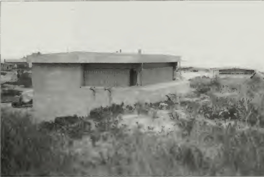
Figure 5.35. Batteries Engle and Peck circa 1920. The battery commander's station for Battery Peck is seen in the foreground. The low concrete structure seen in the background is the coincidence range finder station built into the former gun emplacement of Battery Engle in 1920. Note the low-growing vegetation in this photograph, making possible downrange views and effective operation of the batteries (GATE 7892).
