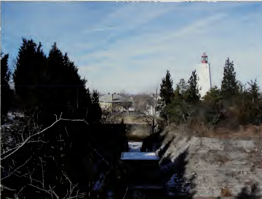
Figure 5.72. View looking northwest above mortar pit, the Mortar Battery. Woody vegetation greater than four-inches diameter should be removed from engineered slopes, and all woody trees and shrubs must not be allowed to grow upon, or within four-feet of a concrete structure or feature (Olmsted Center, January 2009).
