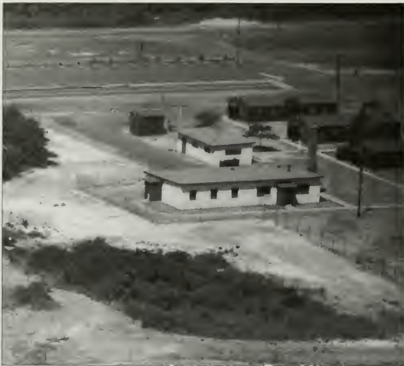
Figure 4.24. Aerial view of the Ready Barracks, NIKÉ launch site, circa 1958. This photograph shows trees growing in the barrack's lawn panels in contrast to bare earth maintained on either side of the fence lines (GATE 5781).
