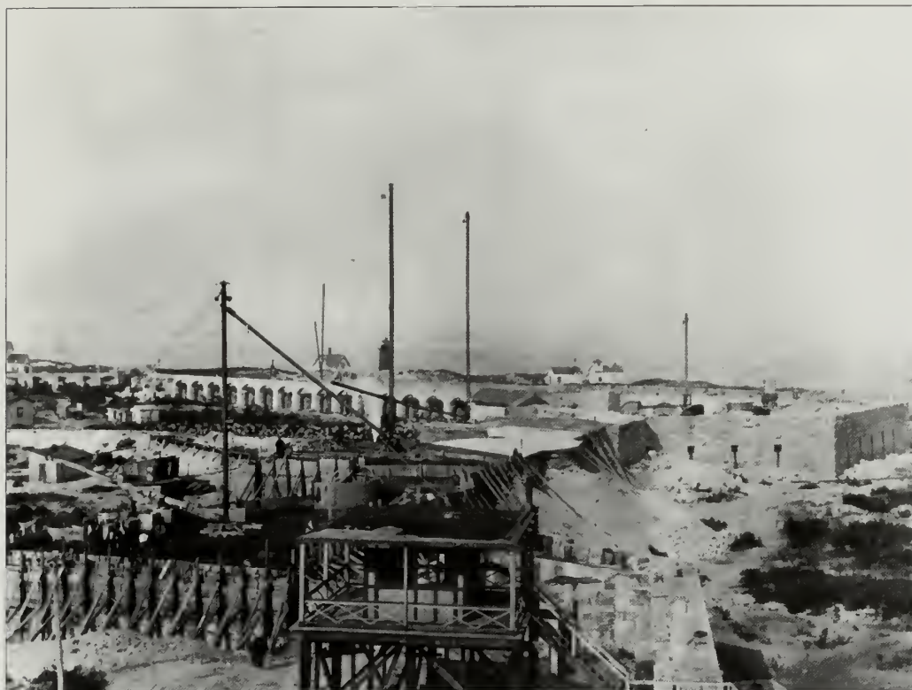
Figure 5.54. Construction of Nine Gun Battery, 1897. The concrete battery structure was built over a Civil War-era granite block fort. The fort's bastions can be seen in the image as the forming of the battery occurs over the fort's eastern wall (GATE 7880).
