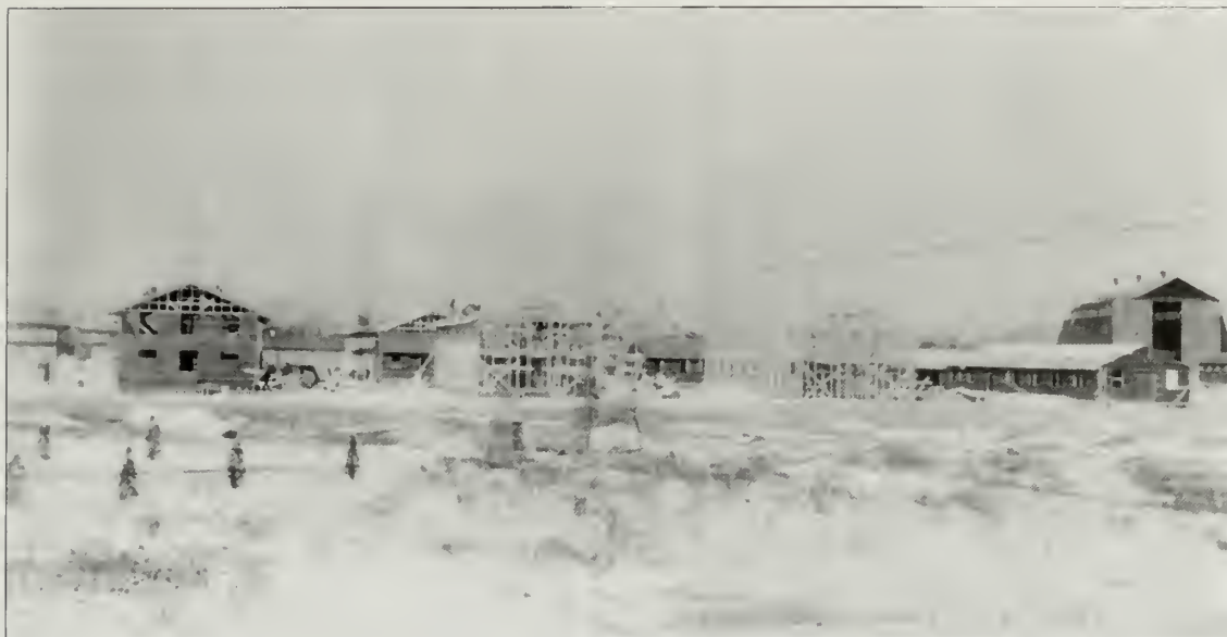
Figure 2.66. Construction of cantonments at Camp Low, circa 1940. To accommodate the personnel increase in preparation for World War II, tent cities were established and a new contingent of wooden barracks and mess halls known as Camp Low was built north of Horseshoe Cove (Thomas Hoffman, Fort Hancock , Charleston, SC: Arcadia Publishing, 2007).
