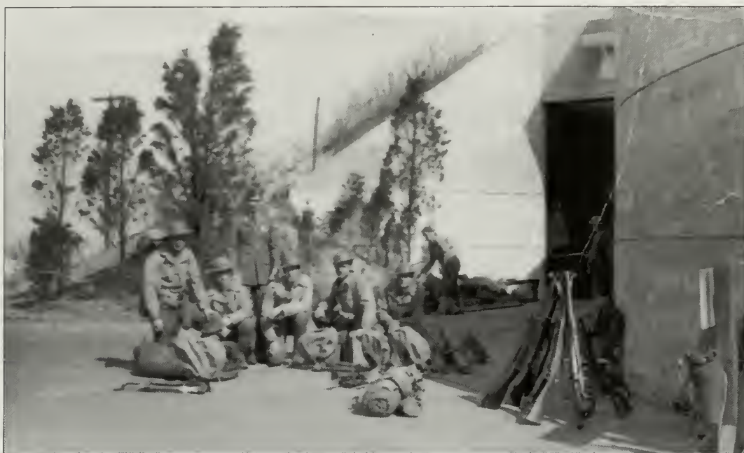
Figure 2.41. View looking northeast at entrance to covered passageway, Battery Kingman, circa 1940. A covered passageway featured standard-gauge railroad tracks embedded into concrete paving to accommodate rail deliveries of shells and gunpowder to the battery (GATE 8092).
