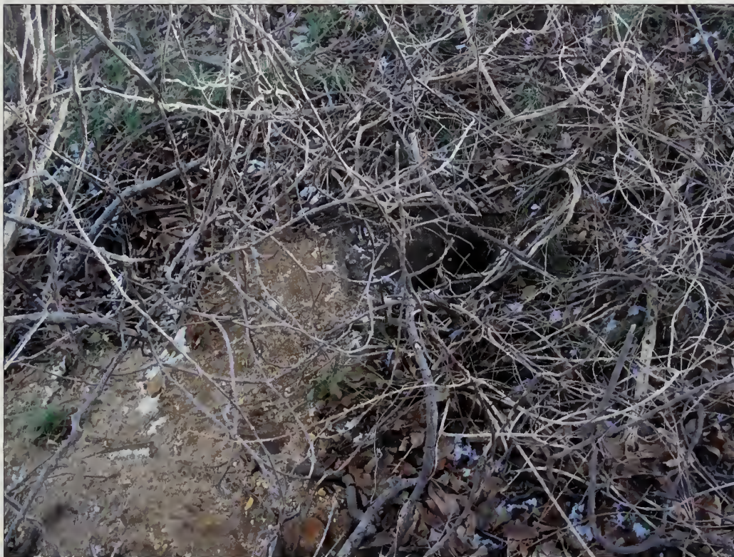
Figure 5.88. Animal burrow on north slope of Battery Kingman. The preferred management recommendation for burrowing animals is to humanely trap the animal and relocate it to an area away from the historic earthwork. The burrow should be filled with soil from a sterile source that does not have the potential to damage archaeological information (Olmsted Center, January 2009).
