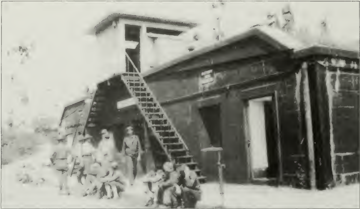
Figure 2.54. View looking northeast at Battery Gunnison, circa 1930-41. Although the east facade featured an engineered earthwork and planting compatible with the surrounding area, the west facade was not camouflaged or concealed. The concrete and metal framework of the structure was clearly visible when approaching from the west (Thomas Hoffman, Fort Hancock , Charleston, SC: Arcadia Publishing, 2007).
