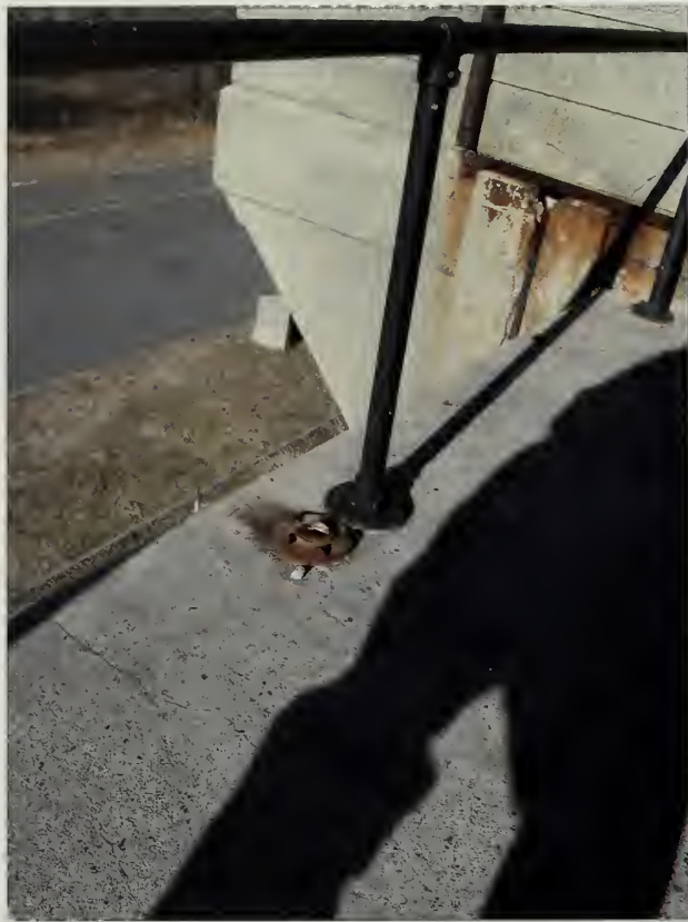
Figure 5.69. Existing safety railings, Battery Granger. At this location and elsewhere throughout Sandy Hook's coastal defense sites, one can see the tangible history of maintenance and repair. This simple railing may be retrofitted with either infill mesh panels or otherwise with woven wire mesh applied with clamps and hardware to satisfy life-safety codes (Olmsted Center, January 2009).
