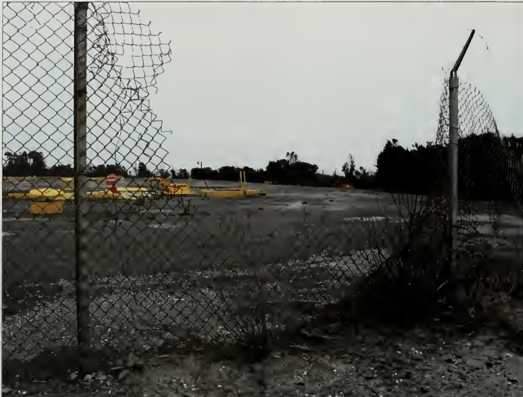
Figure 5.122. View looking northeast across missile magazines, NIKE launch site. After vegetation removals the inner, outer, and kennel fences should be inspected, repaired where needed, and replaced where damaged or severely deteriorated (Olmsted Center, April 2008).
