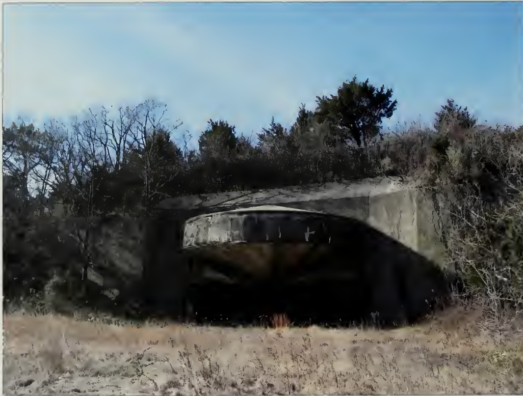
Figure 5.85. View looking southwest at north gun emplacement, Battery Kingman. Although visitors are warned of the hazards of accessing the summit of these batteries, existing chain-link fencing located above the concrete casemate canopies should be maintained for added safety at both Battery Kingman and Battery Mills (Olmsted Center, January 2009).
