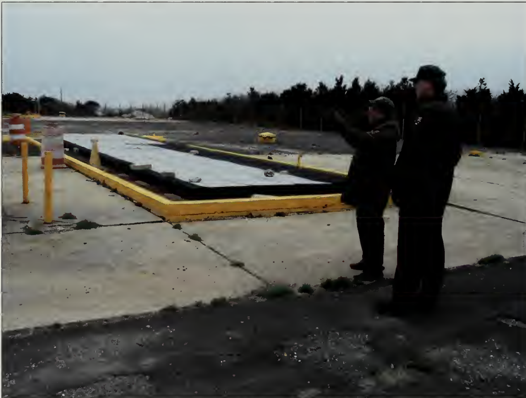
Figure 3.64. View looking west at elevator to missile magazine (425), NIKÉ launch site. The northern section of the launch site contains the underground missile magazines and concrete pads for launching racks. The concrete pads are oriented north to south for firing missiles to the east (Olmsted Center, April 2008).
