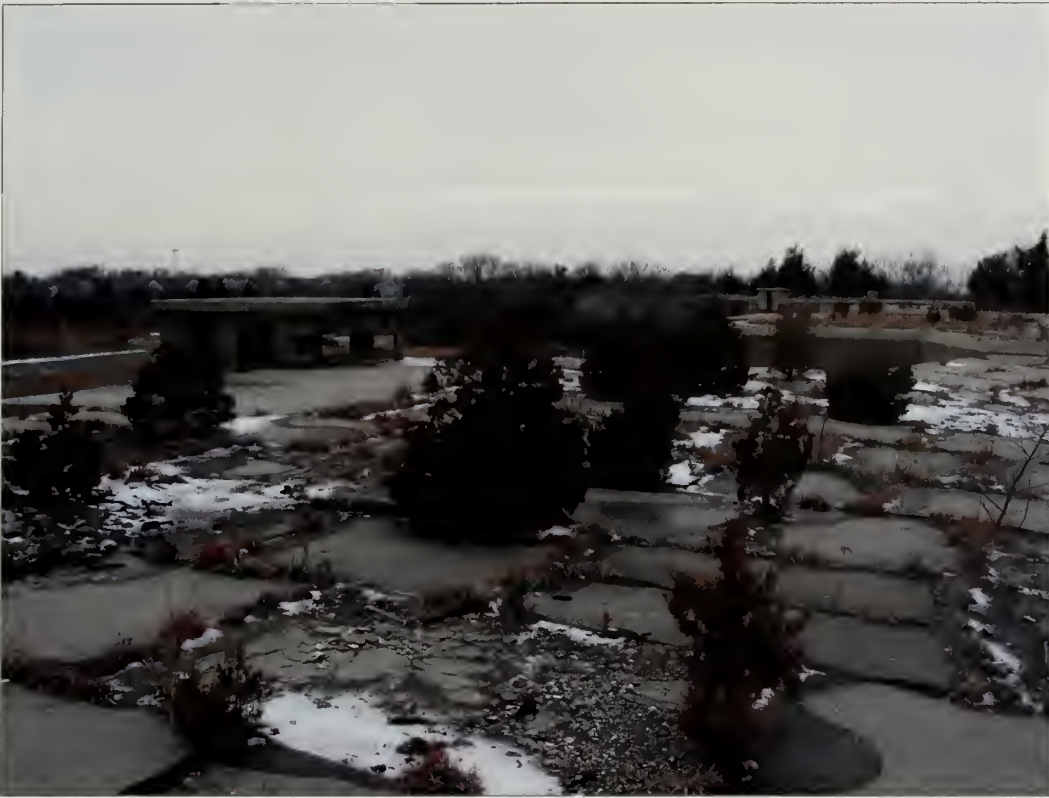
Figure 3.21. View looking west toward battery commander's station Bloomfield, Nine Gun Battery. In addition to growing on the engineered earthwork, eastern red cedars ( Juniperus virginiana ) have emerged in the cracks and cold joints of the battery's horizontal concrete surfaces (Olmsted Center, January 2009).
