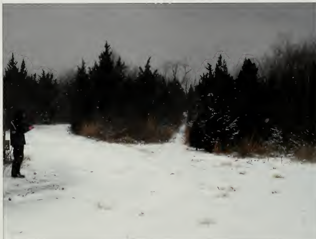
Figure 5.99. View looking northwest at pedestrian walkway, Control Area #1, NIKE radar site. Following the site's closure woody species, especially eastern red cedars, have emerged and are encroaching on pedestrian circulation features as well as buildings and the perimeter fence (Olmsted Center, January 2009).
