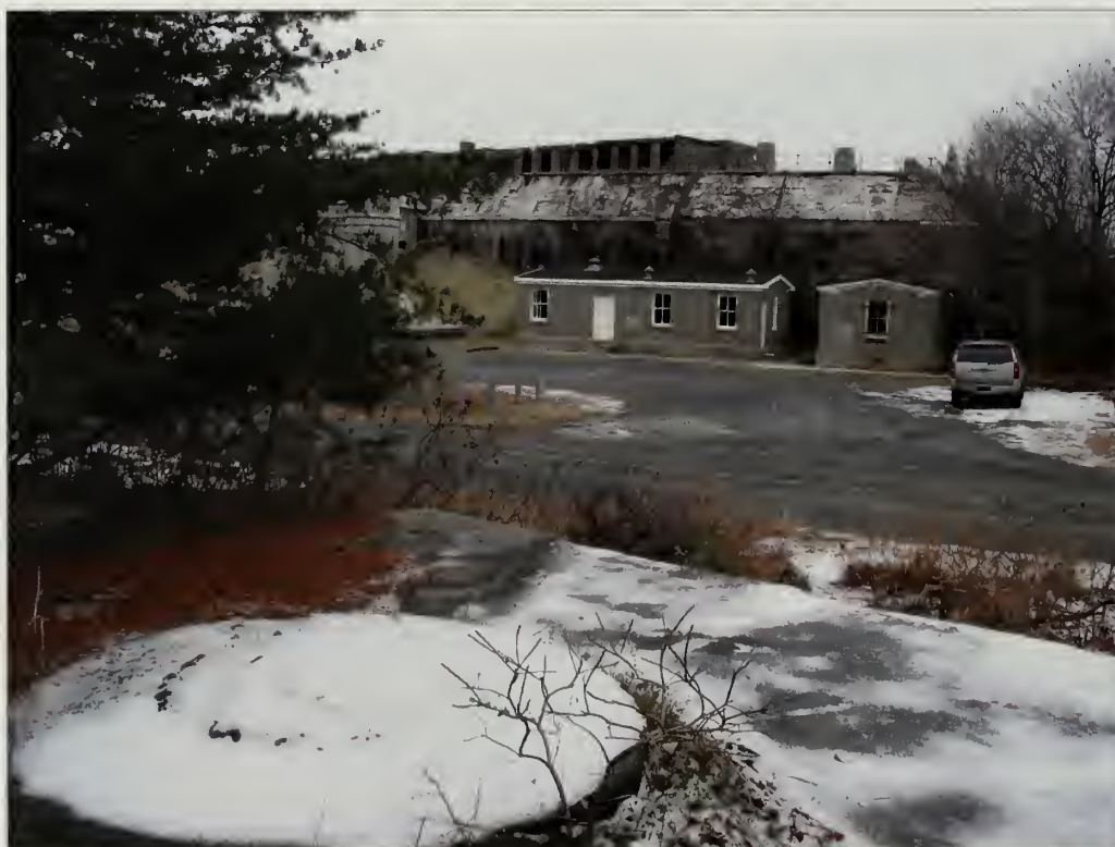
Figure 3.32. View looking northeast at foundation, Hudson Drive, and Battery Potter. Across from the parking area and west of Hudson Drive, a concrete foundation occupies a small opening in a dense stand of woody vegetation. The foundation supported a metal tower used to identify targets and improve fire control (Olmsted Center, January 2009).
