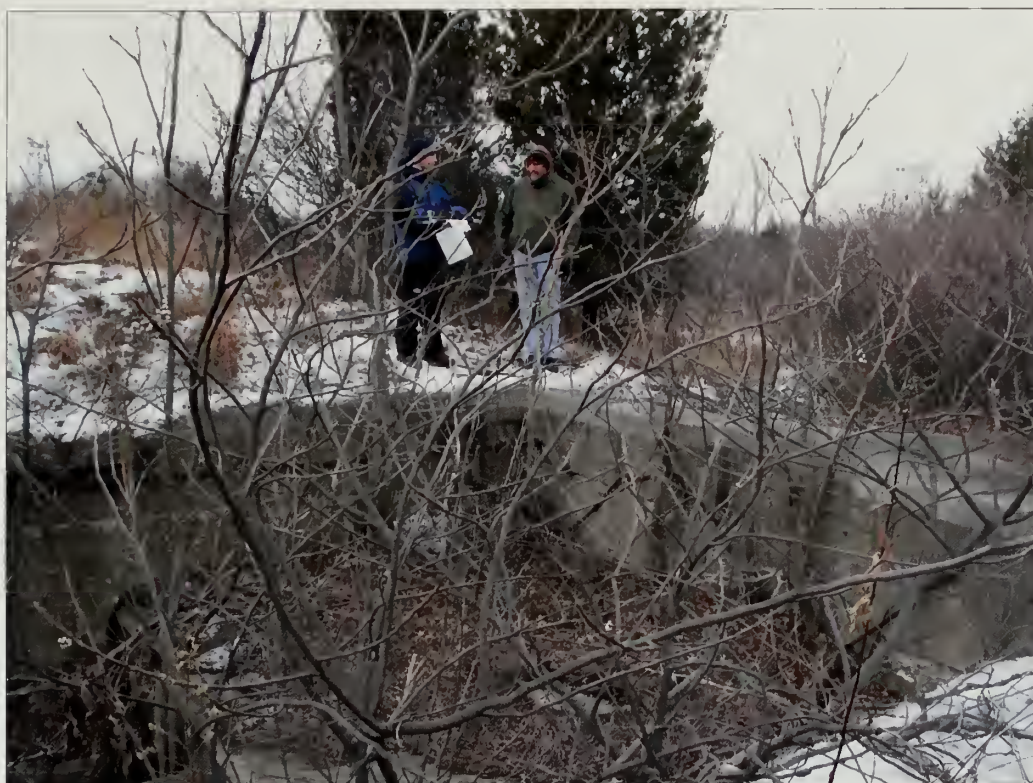
Figure 5.9. View looking northwest across gun platform #4, Battery Urmston. Low and flat areas like this gun platform have accumulated soil, leaf litter, and moisture. These conditions have resulted in the growth of woody vegetation that should be removed from the structure (Olmsted Center, January 2009).
