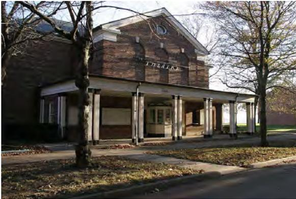
**Building 330** is a 700-seat theater with a stage and projection screen, built in 1937. The charming ticket booth, curving entrance ramps and theater area are all in excellent shape. The building has a cast-in-place concrete slab on grade system with cast-in-place concrete footings under load-bearing brick columns and walls. The slate roof is recently renovated.
