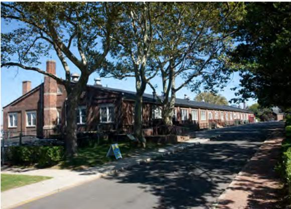
**Building 110** was constructed in 1879 and enjoys unmatched views of lower Manhattan from its lengthy northern façade. The building has brick on masonry bearing wall construction and much of the interior has wood columns at 12’ spacing. New HVAC and fire suppression systems were recently installed through most of the building and a new roof is being installed. Building 110 is directly adjacent to Soissons Landing. A portion of the upper floor is currently in use for artists’ workspaces.
