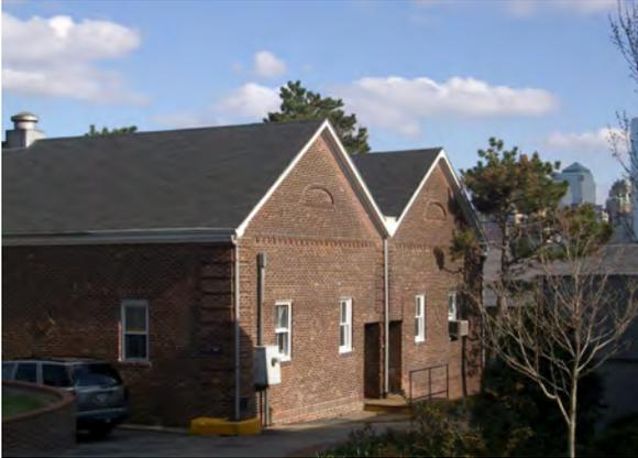
**Building 109** is an open floor plan building constructed in 1945. It is situated in a prime location adjacent to Soissons Landing. The double gable building is brick on masonry bearing walls. The roof is in poor condition and the structure is a shell only with some structural concerns.
