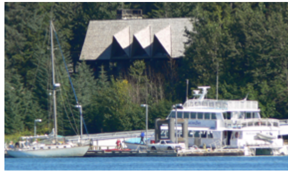
(above) A current view of the Glacier Bay Lodge and the public use dock. While the lodge site was selected for its scenic views, active vegetation management is needed to maintain the view because of the dynamic landscape (e.g., isostatic uplift at ~1 inch a year, less than 200 years of plant succession, and temperate rainforest conditions with ~70 inches of precipitation annually).
