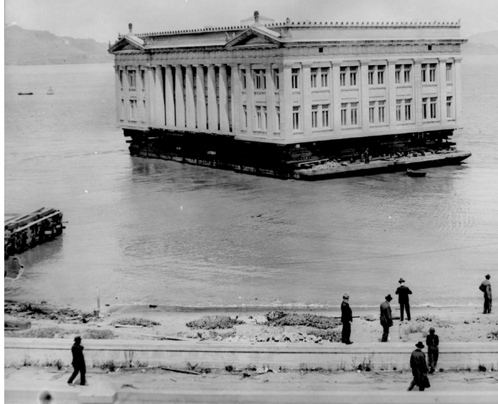
After the fair, everything had to go and the lands had to be restored to their pre-fair appearance. Here the Ohio State Pavilion floats away on a barge, intended for re-use at another municipality. Image courtesy of the California Historical Society.
