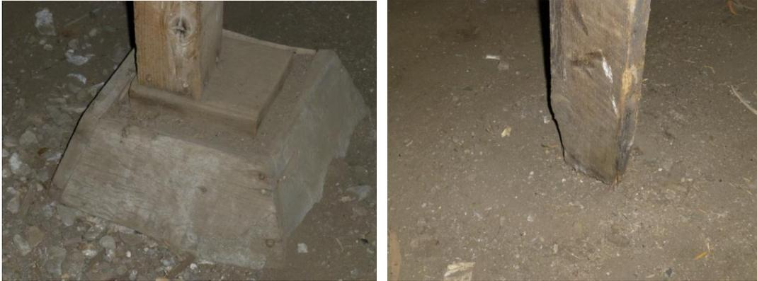
Eccentrically loaded pier footing at centerline of building and column in connection with dirt. (NPS Photos 2013)
