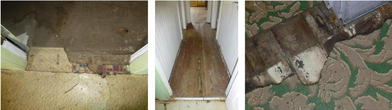
Two layers of laminate (Room 205), wood floor condition (room 211), painted wood floor under laminate (Room 213) (NPS Photos 2013)
