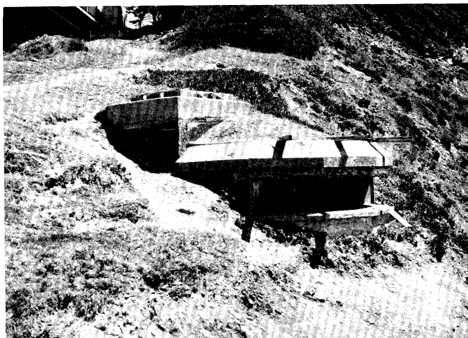
23. A Pre-World War II Concrete Fire Control Station on Fort Point, Fort Winfield Scott.
