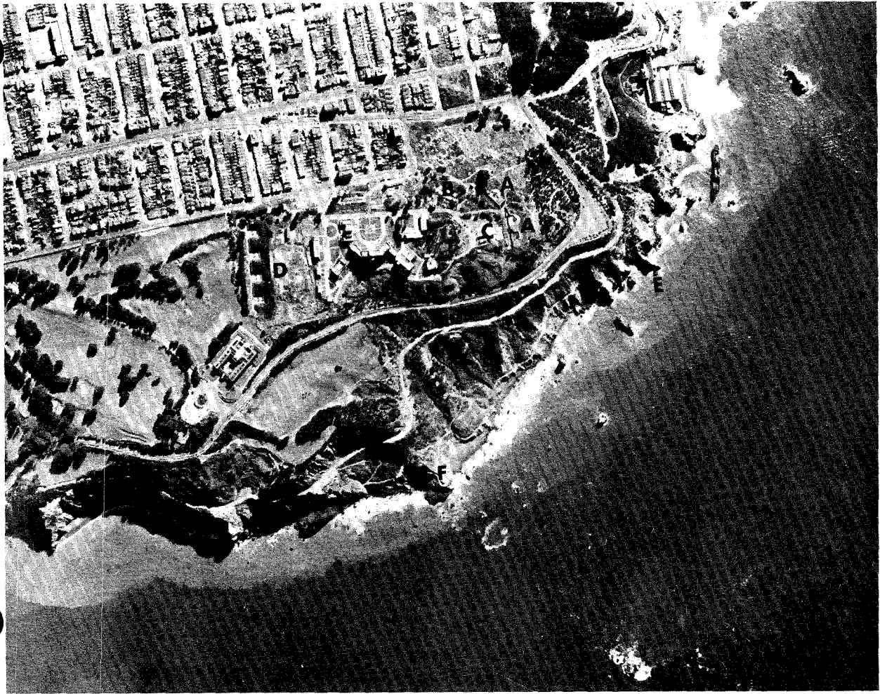
35. Aerial Photograph of Fort Miley, 1937.
