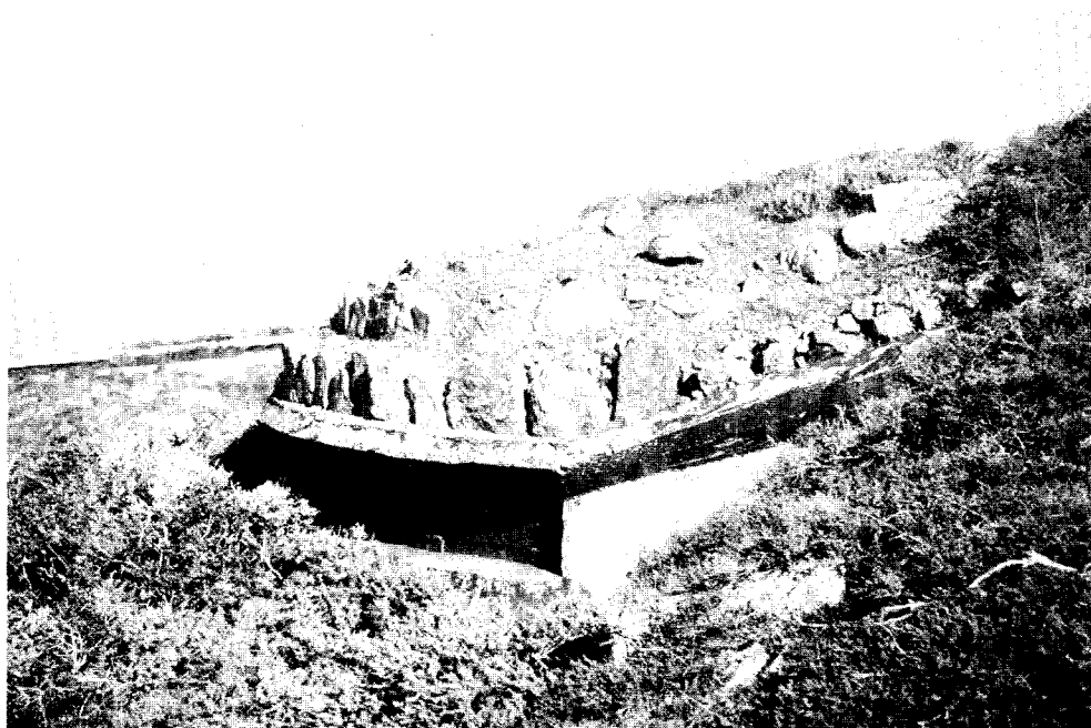
21. A Well-Camouflaged Fire Control Station, Also Located on Wolf Ridge, Fort Cronkhite.
