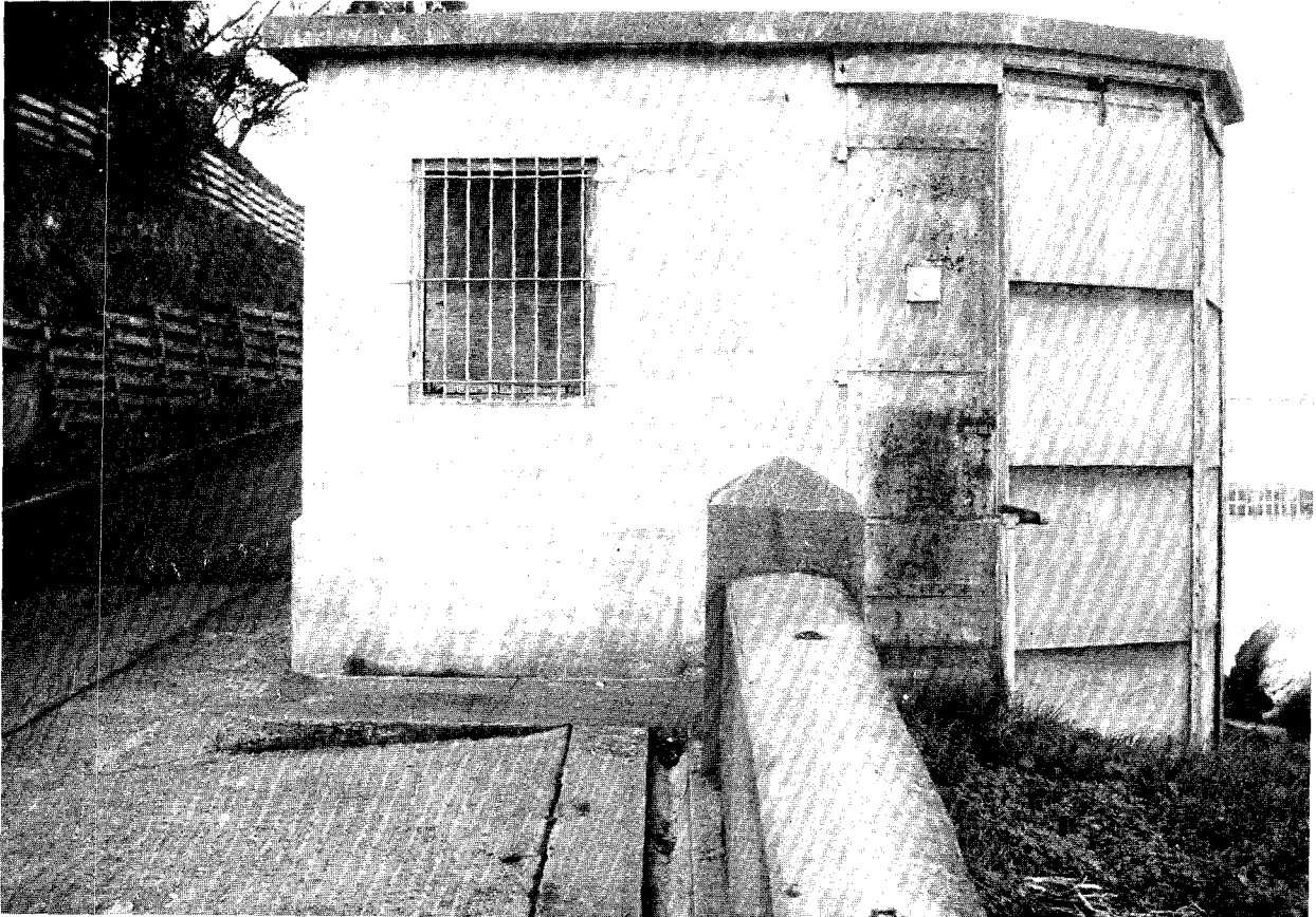
17. Steel Shelter for a 60-inch Seacoast Searchlight, Fort Mason.
