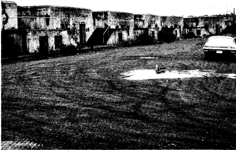
10. Battery Yates, Fort Baker, Six 3-inch Guns on Pedestal Mounts. Constructed in the Endicott period, Yates continued to be armed (two guns only) through World War II. Erwin N. Thompson, NPS, 1975.
