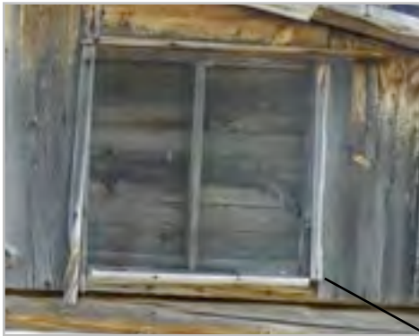
5 Construct sash with muntins matching those on east side. Repair / refasten trim.
