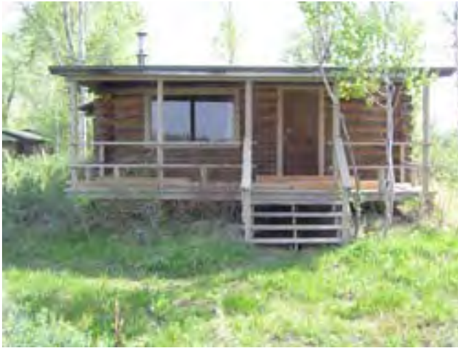
Figure 58 – Looking south at the front porch and entrance to the cabin. The cabin is in good condition and sits up on a good concrete foundation.
