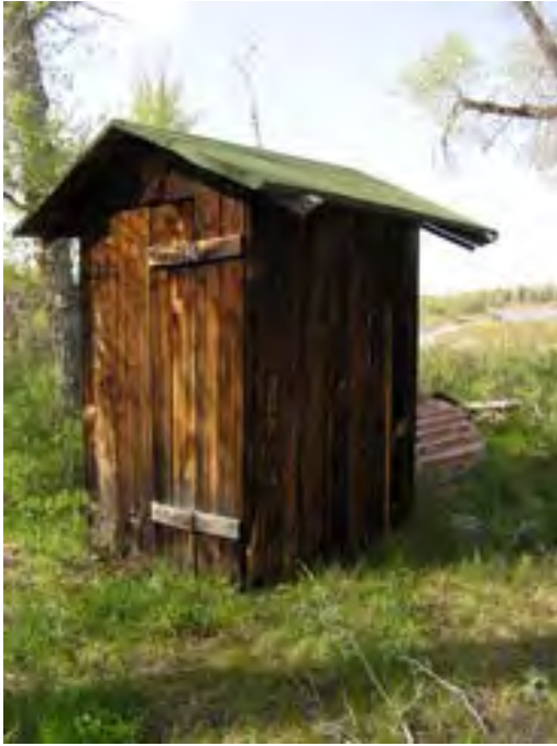
Figure 92 – Looking northwest at the smokehouse. The wood on the walls is very dry and there is some rot on the base of the building where soil has built up around the base of the structure. The door is in poor condition.
