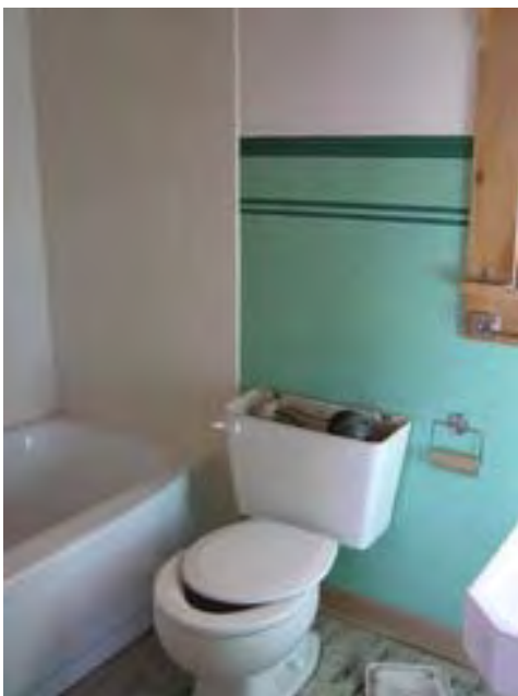
Figure 66 – Looking west at the bathroom. Note the sheetrocked walls with tile wainscot.
