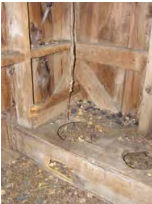
Figure 181 – Looking southwest at the interior of the outhouse. Note the filled in holes and the stained and rotted wood.
