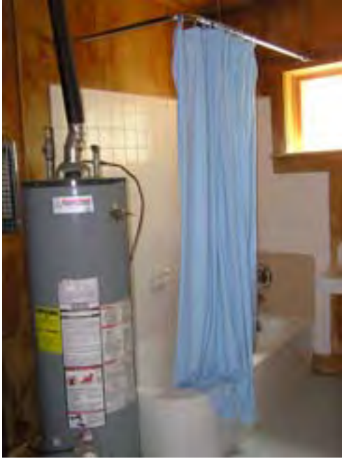
Figure 127 – Looking southeast at the water heater and bathtub in the bathroom.
