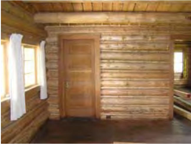
Figure 41– Looking north at a typical wall and wood paneled door in the great room.
