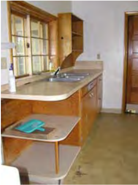
Figure 47– Looking south along some of the 1960's cabinets in the kitchen.
