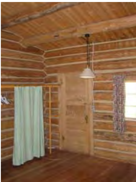
Figure 114 – Looking northwest at the wood paneled entrance door, window and closet. Most of the materials are in good condition.
