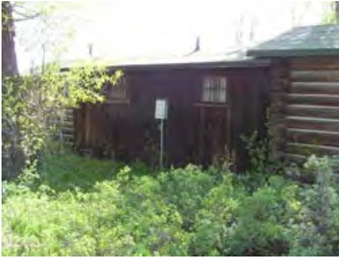
Figure 73– Looking at the center wood frame structure that connected the two log cabins. The wood is very dry and the base is rotted due to soil build-up around the building.
