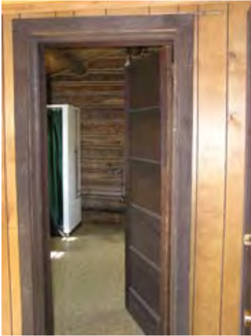
Figure 89 – Looking north at the connecting hallway and door to the bathroom in the log cabin portion of the building.
