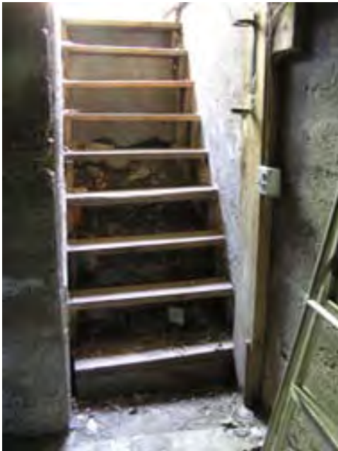
Figure 39 – Looking east at the stair to the exterior from the basement.
