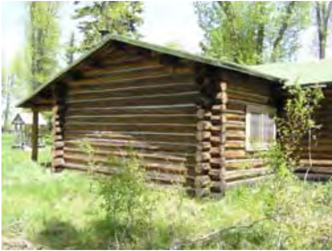
Figure 124 – Looking northeast at the cabin. Note the soil build-up around the base.
