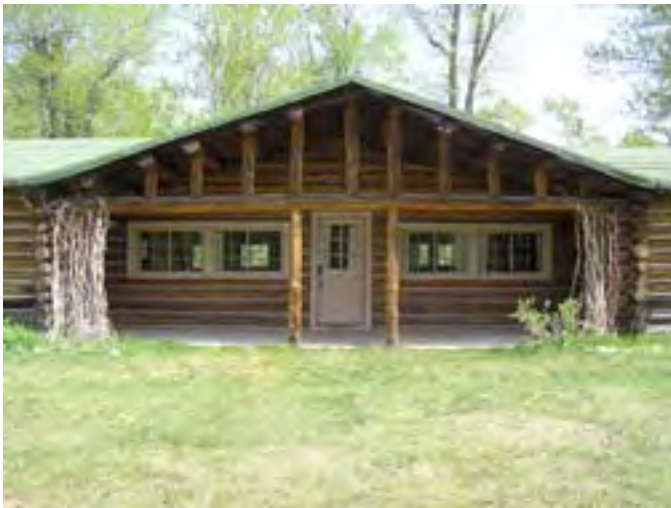
Figure 24. Looking east at the main entrance to the Lodge and the gable roof with the log structure.
