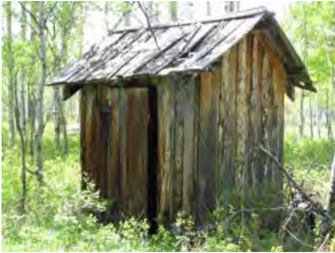
Figure 179 – Looking southwest at the outhouse. The building is in poor condition with weathered wood, a failing board and batten roof and rot along the base because of soil build-up.
