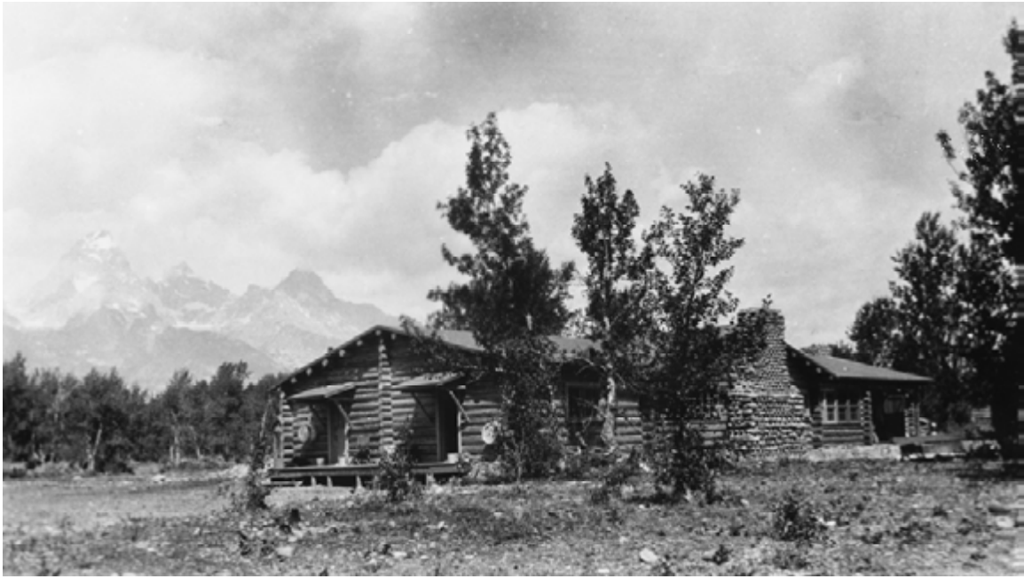
Figure 3. Looking northwest towards the south and east walls of the Lodge, soon after completion. Source: Collection of the Jackson Hole Historical Society and Museum, Jackson, Wyoming [1958.2031.01].
