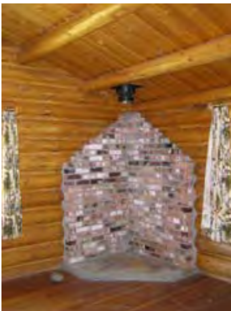
Figure 155 – Looking northwest at the corner of the bedroom with fire wall for the wood stove. The materials are in good condition.
