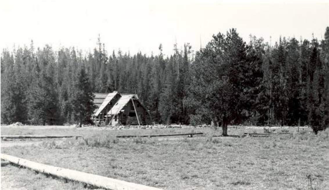
Superintendent's residence (HS-1) under construction, summer 1934. Also note log fencing lining the parking and drive areas. Source: GRTE Cultural Resource files.
