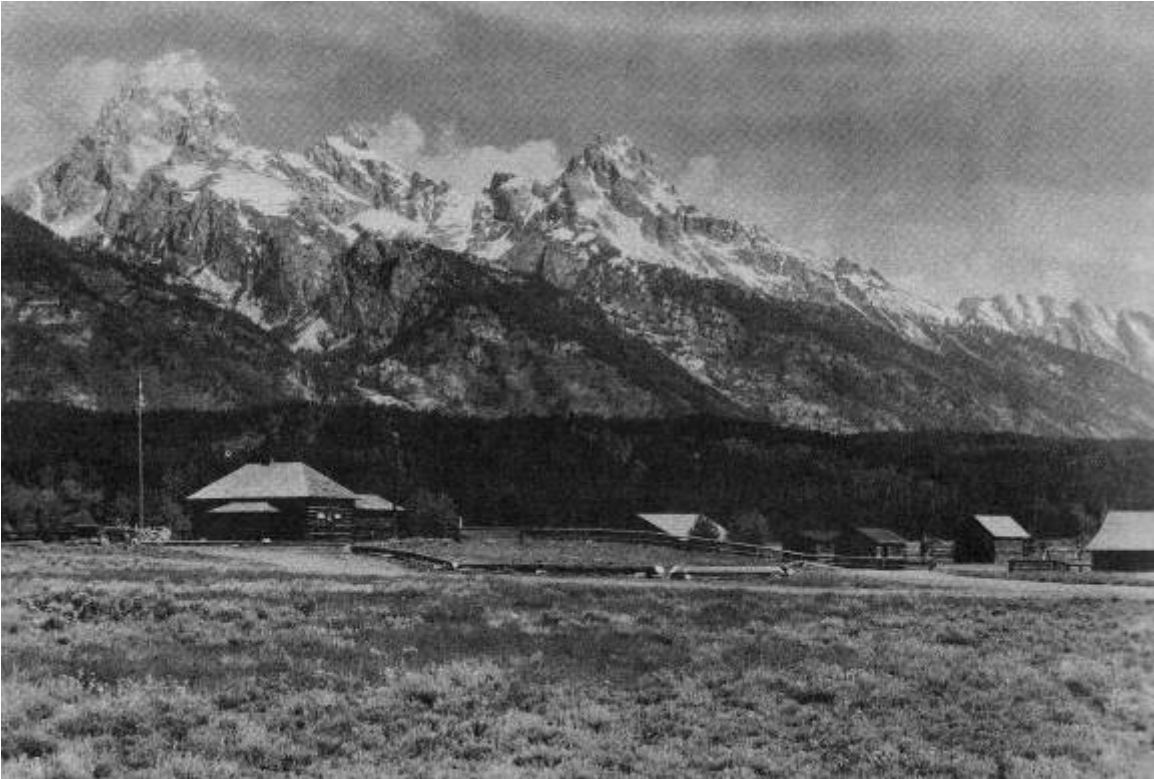
Cluster of early park buildings showing Administration Building (HS-10) and utility area buildings to the north, 1929-1934. Source: GRTE Cultural Resource files.
