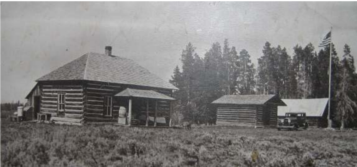
Forest Service Ranger Station, residence, and unidentified building sometime between 1908 and 1929. The Ranger Station and residence were later joined to create the Administration Building HS-10. Also note the loop drive with central flagpole. Source: GRTE Interpretive panel, Maud Noble cabin.
