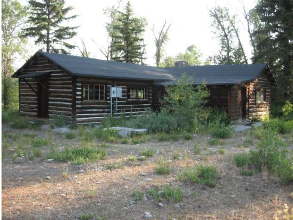
View looking northwest at the Maud Noble cabin 1916, moved 1918 (National Park Service, July 2010).
