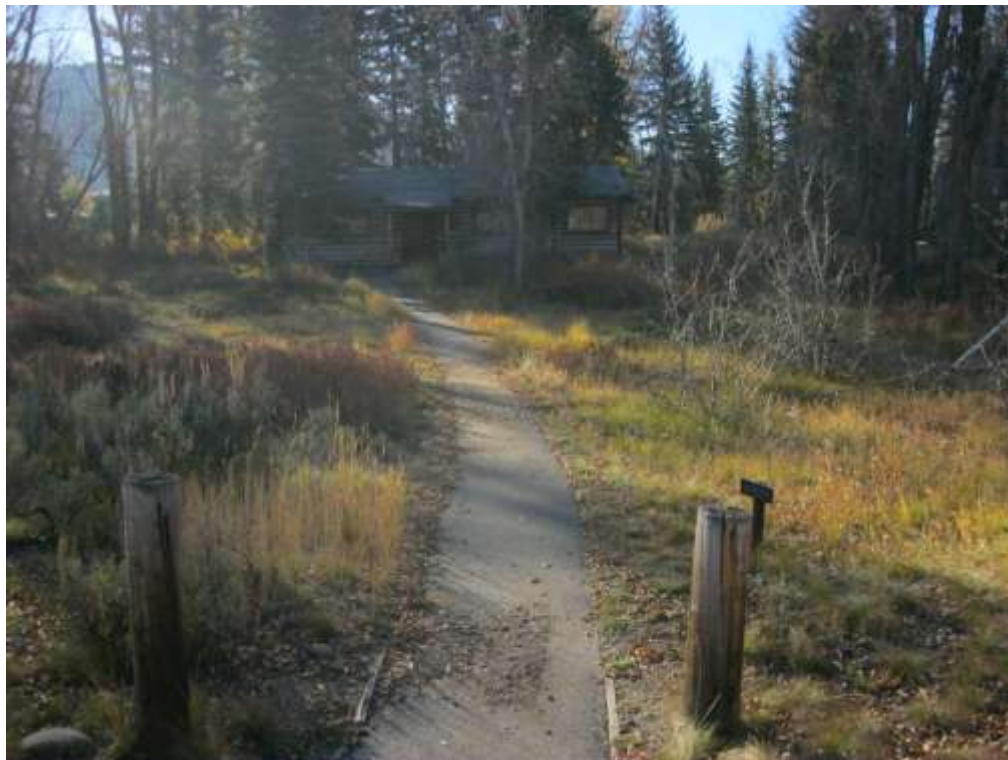
View looking west down the path leading to the Maud Noble cabin (National Park Service, October 2010).
