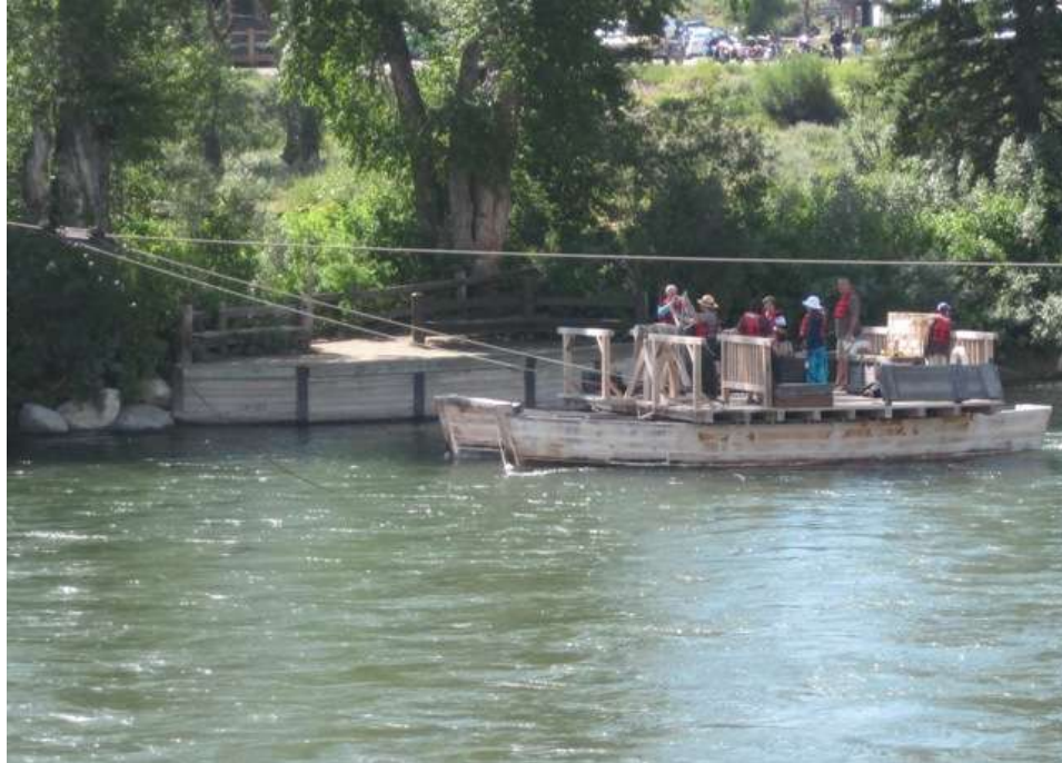
View looking east of Menor's Ferry reconstructed 1990, pontoons reconstructed 2001 (National Park Service, July 2010).
