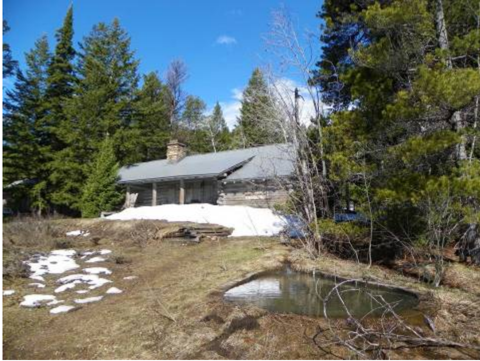
View looking southwest toward the Grand cabin with the concrete pond in the foreground. Source: National Park Service, 2011.
