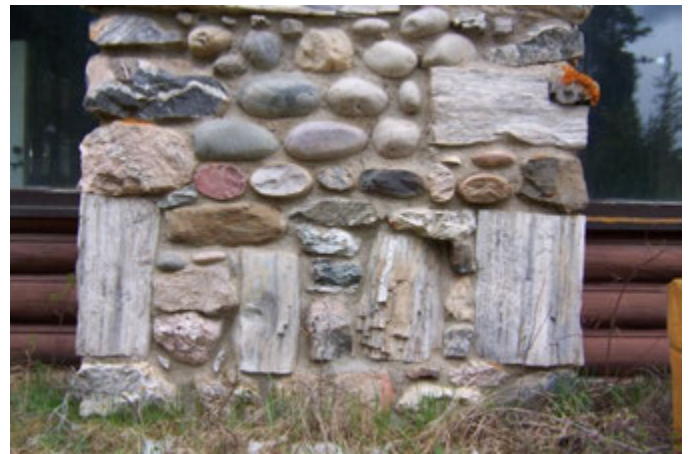
Fig. 20 – Detail of lower Chimney
