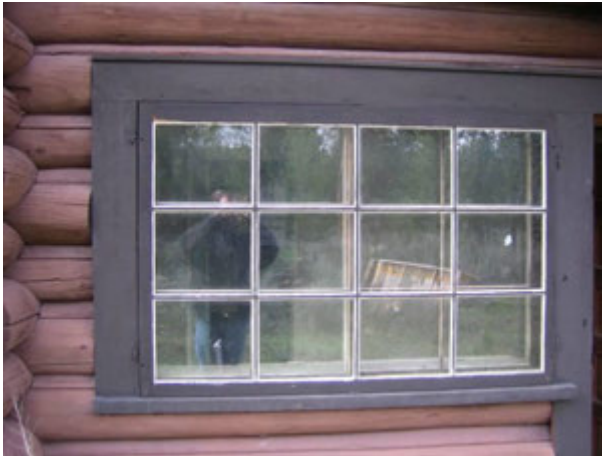
Figure 47 Window with fully intact storm window
