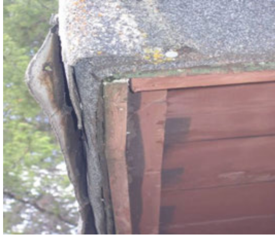
Rolled roofing covering fascia
