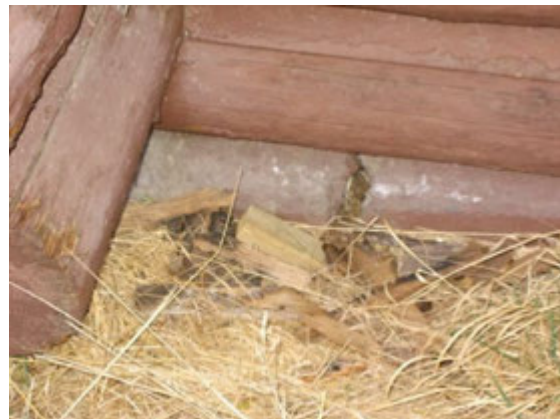
Figure 31 Bedroom 2 foundation freeze and thaw action and cracks
