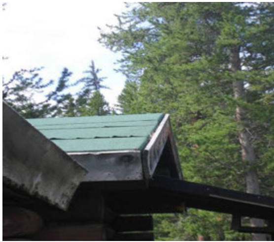
Figure 44 Rolled roofing w/ fascia covering flue
