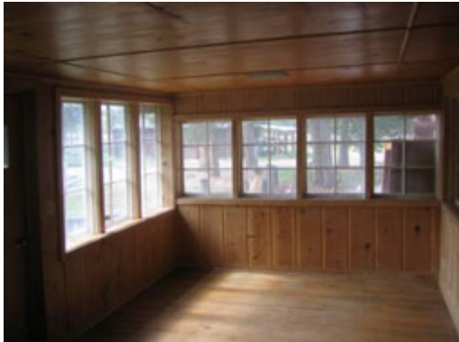
Figure 59 East porch enclosure
