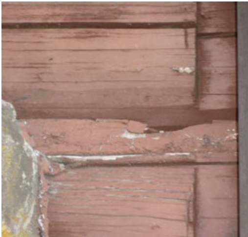
Figure 48 Daubing Deterioration
