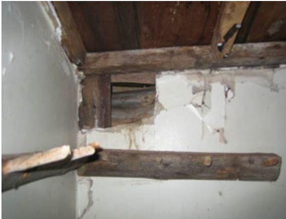
Figure 36 Log walls furred and sheetrock covering
