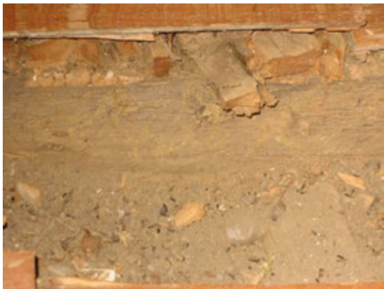
Figure 32 Rotting log sleepers and sub floor in Bedroom #3
