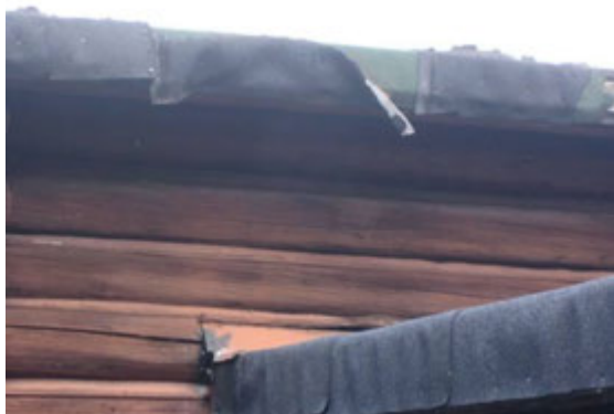
Figure 45 Rolled roofing covering fascia
