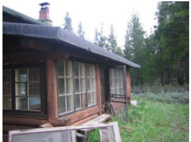
East porch enclosure with windows and door
