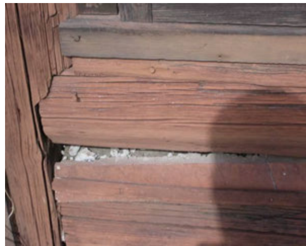
Daubing Deterioration 2
