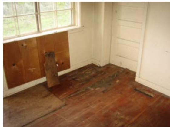
Figure 32 Rotting log sleepers and sub floor in Bedroom #3
