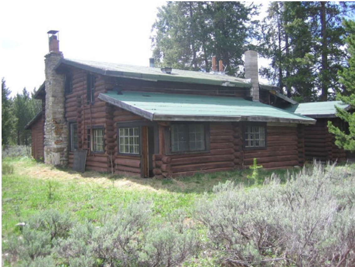
Figure 10 Building #117 northwest corner
