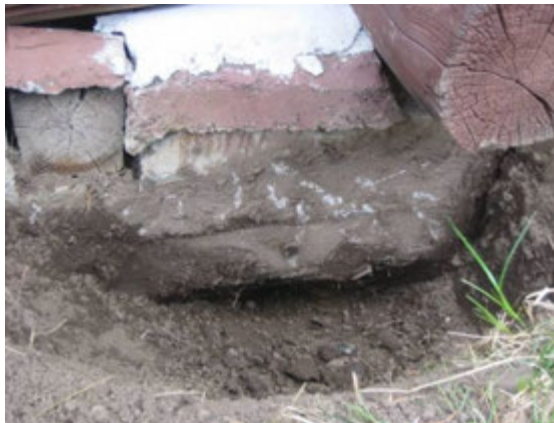
Figure 31 Bedroom 2 foundation freeze and thaw action and cracks
