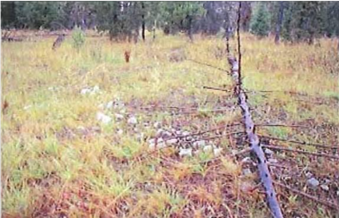
Caption: Looking northeast to the stone foundation for one of the bachelors' cabins, 2004. Source CLR.
