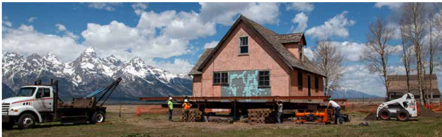
Moving the pink house off its foundation to repair the understructure.
