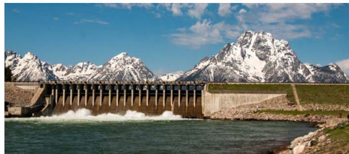
The dam on Jackson Lake increased the natural lake by 38 vertical feet and provides water storage for downstream users.
