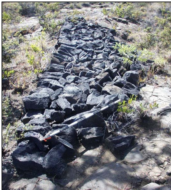
Figure 31. HAVO-2005-D-15, Retaining Wall
