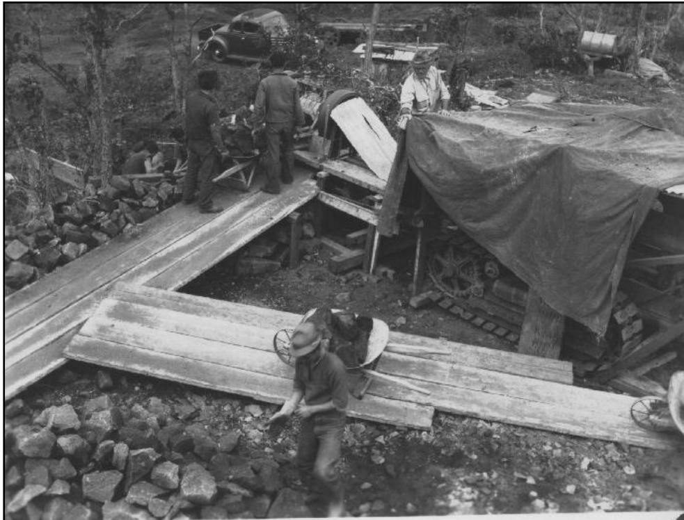
Figure 19. Portable rock crushing plant utilized by the CCC. Photo Courtesy of the National Park Service, Superintendent Reports, HAVO Archives, 1940
