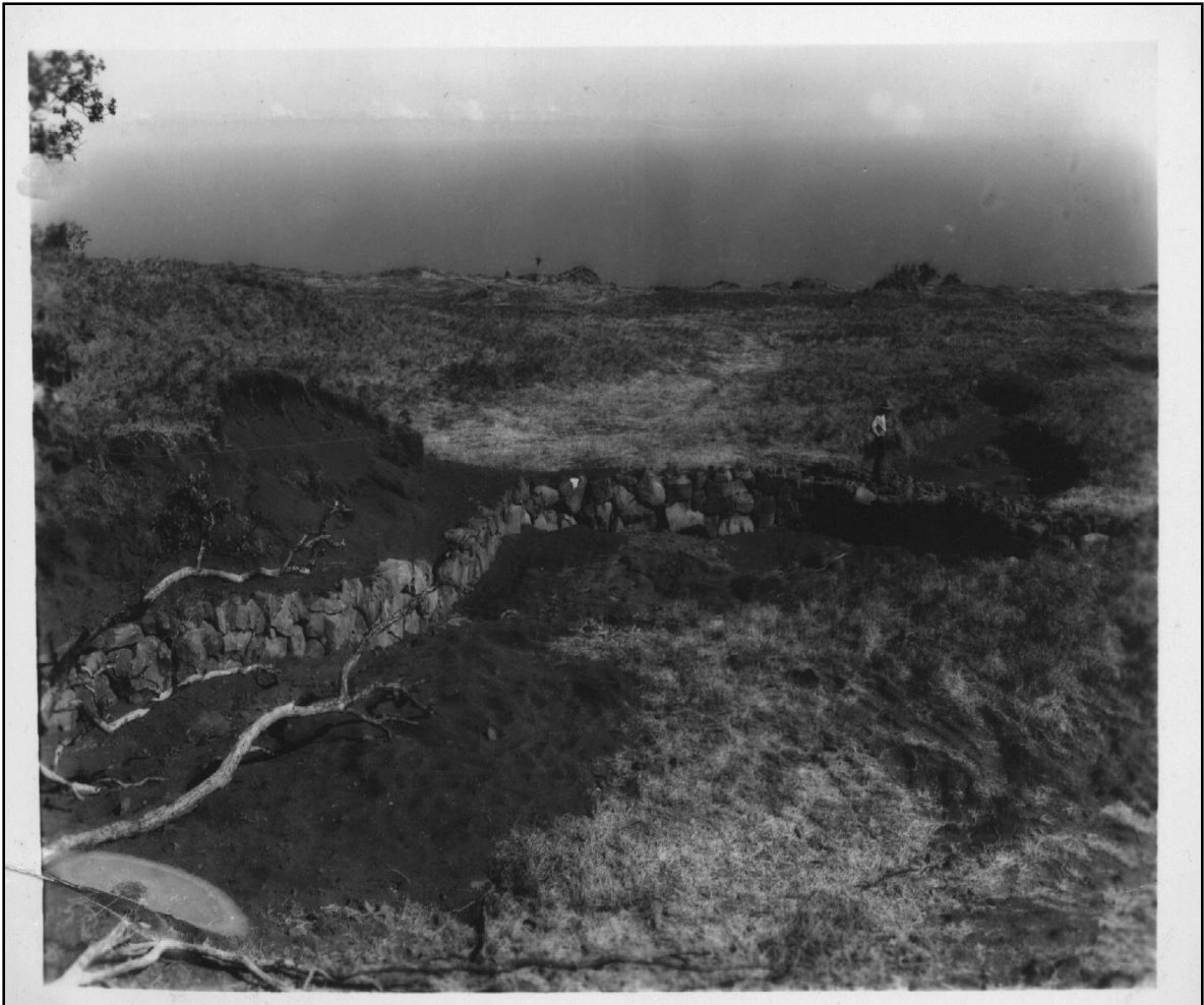
Figure 25. CCC Job 327, wall construction
