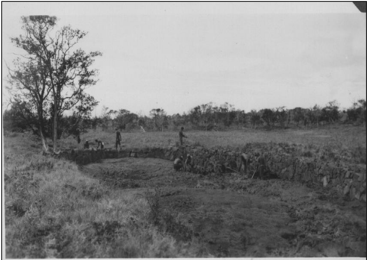
Figure 18. Caption Reads: “Erosion Control Project- Hilina Pali CCC Job 327, showing bank retaining wall and rock check dam”
