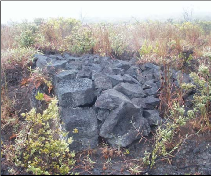
Figure 54. HAVO-2005-D-97 Dam Wall
