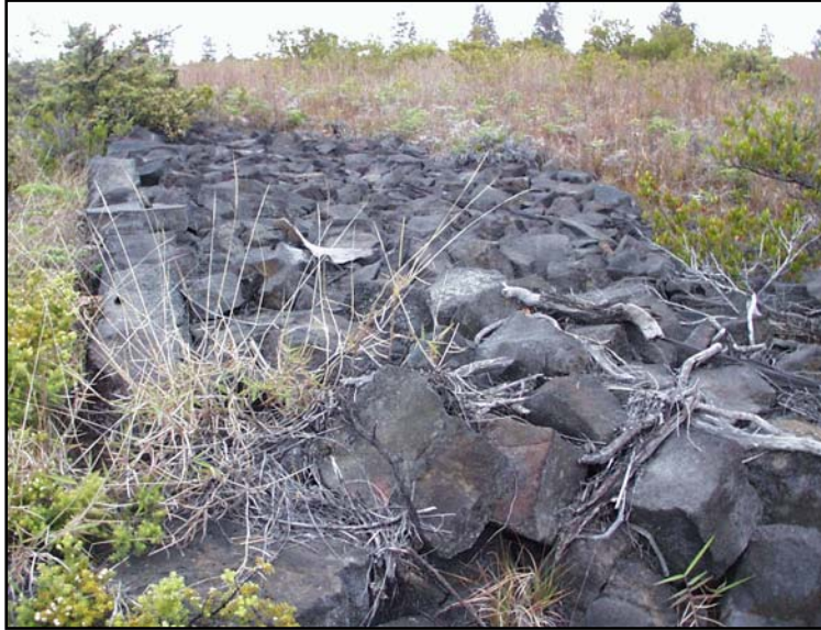
Figure 40. HAVO-2005-D-41 West Wall
