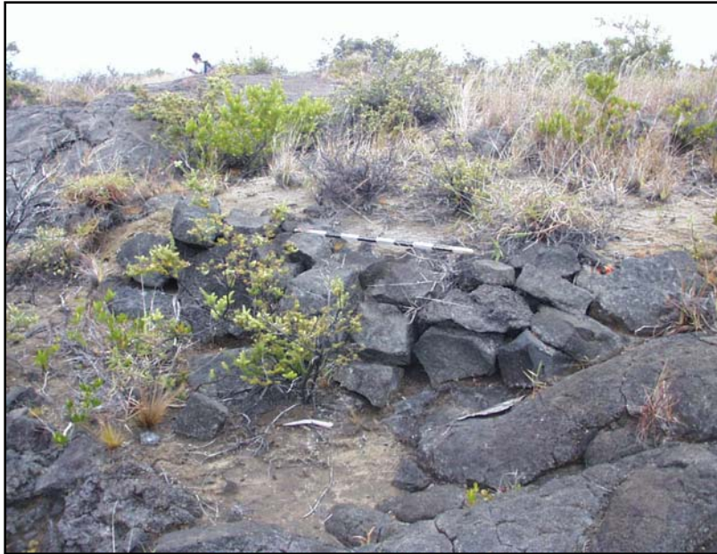
Figure 53. Feature HAVO-2005-D-86 Rock Wall
