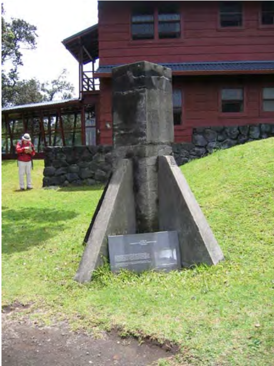
Buildings and Structures #3. Contemporary photo of the concrete pillar at the Whitney Seismograph Vault. The vault is beneath the mound in the background. (PWRO 2005)
