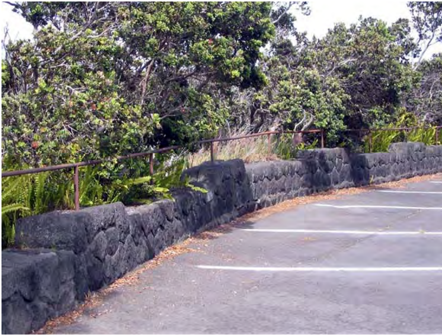
Buildings and Structures #5. The stone guard wall at Puu Puai parking lot was once along the Crater Rim Drive alignment. The metal guard rail was installed after the period of significance. (PWRO 2005)
