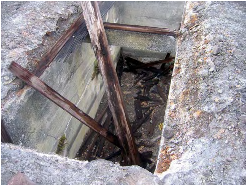
Archeological Sites #3. One of two concrete vaults cut into the lava near the Halemaumau parking lot. These vaults were likely the two comfort stations built sometime in the 1920s or 1930s. (PWRO 2005)
