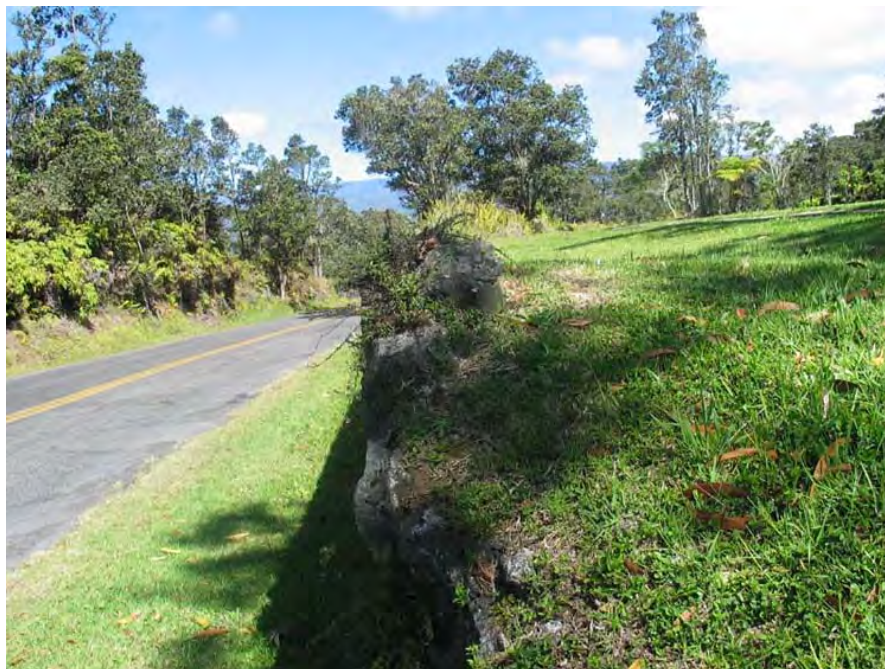
Topography #3. The terrace that held the Volcano House before 1940 is retained by a combination of stone retaining wall and natural rock cut. (PWRO 2005)
