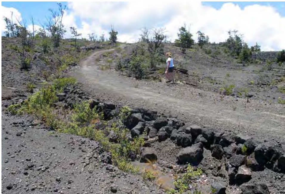
Circulation #2. Road traces and remnant retaining walls, most likely from Leavitt's Road from Uwekahuna to Halemaumau built in 1931, are today part of the Crater Rim Trail in the northwest corner of the caldera. (PWRO 2005)
