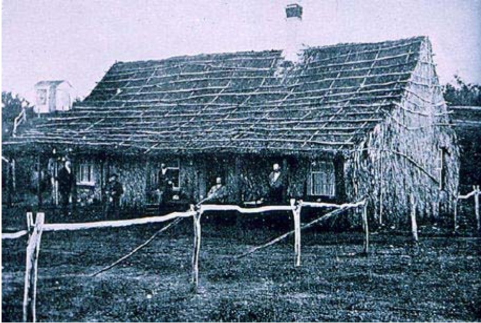
History #1. The grass thatch and ohia pole Volcano House built in 1866. It was here that Mark Twain stayed during his visit to Kilauea the same year. (Olson 1941)
