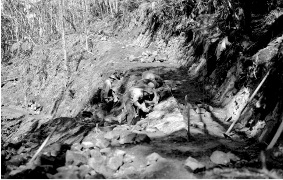
History #11. CCC crew laying stone embankment facing on a switchback of the Kilauea Iki trail in 1934. (HAVO Landscape Architect's Reports 1934)
