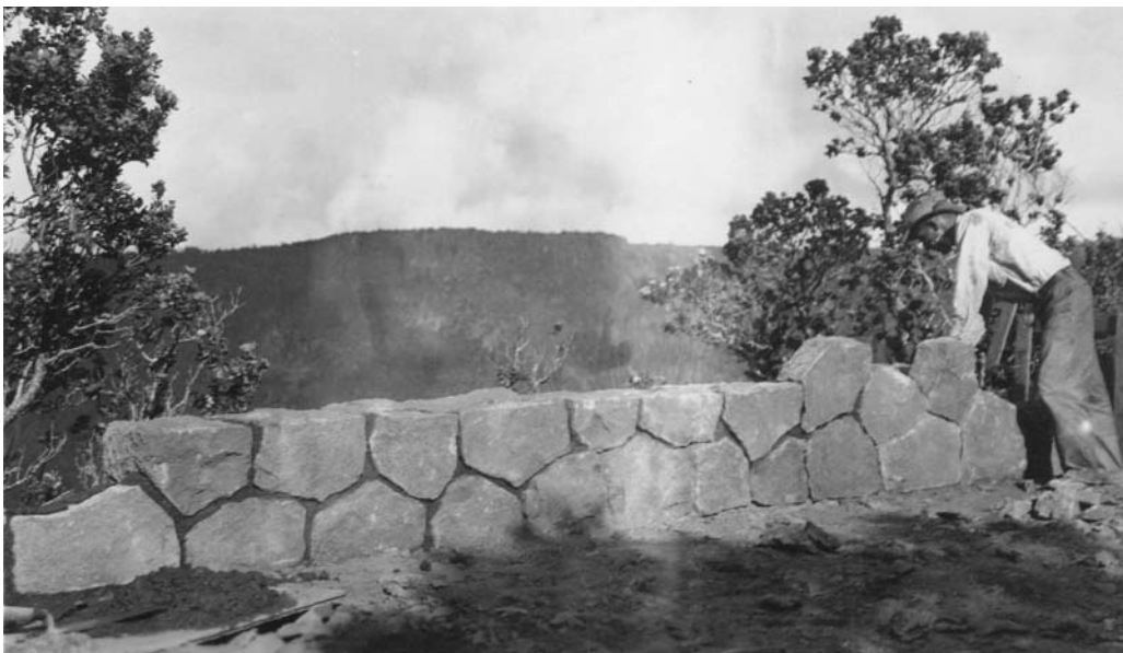
History #8. Parapet guard wall under construction in 1934. All of the guard walls constructed along Crater Rim Drive conformed to the specifications for the Type 2 guard wall developed by the NPS landscape department. (HAVO Landscape Architect's Reports 1934)
