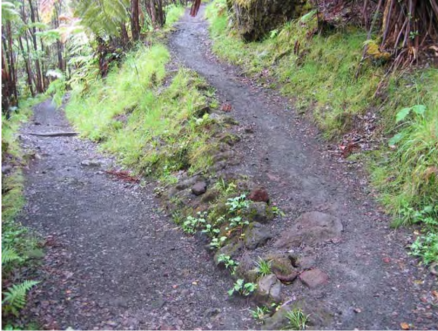
Topography #4. Contemporary photo showing grading on the Kilauea Iki Trail, built by the CCC in 1934. Stone riprap and dry-stacked retaining walls were used to support the steep slopes and switchback corners. (PWRO 2005)
