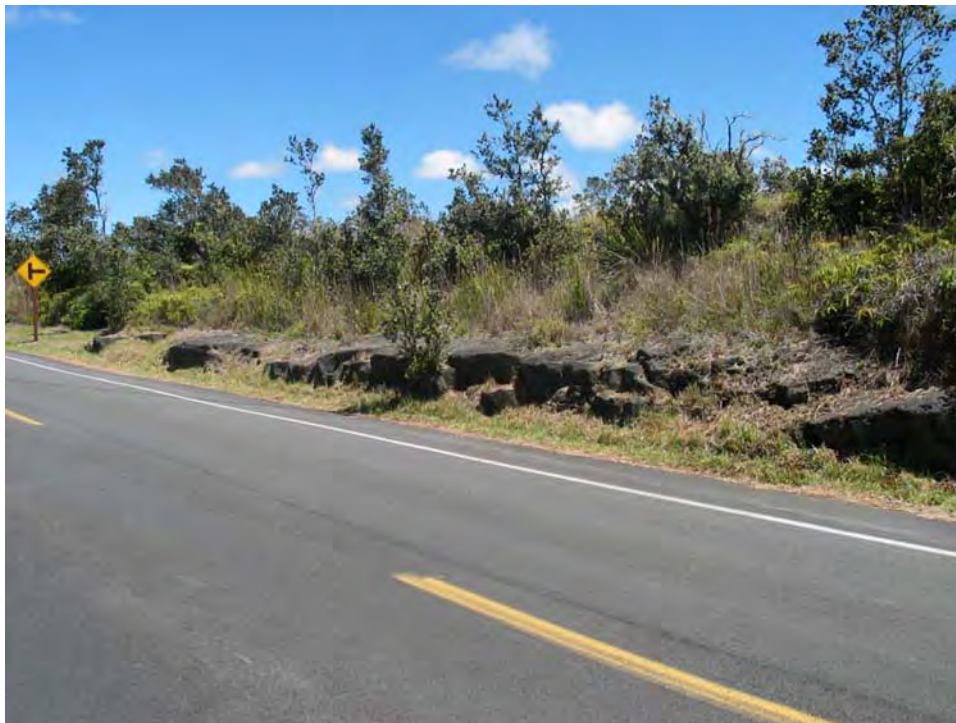
Topography #1. Rock cuts in the dark volcanic rock west of the headquarters site look like natural rock outcroppings. (PWRO 2005)
