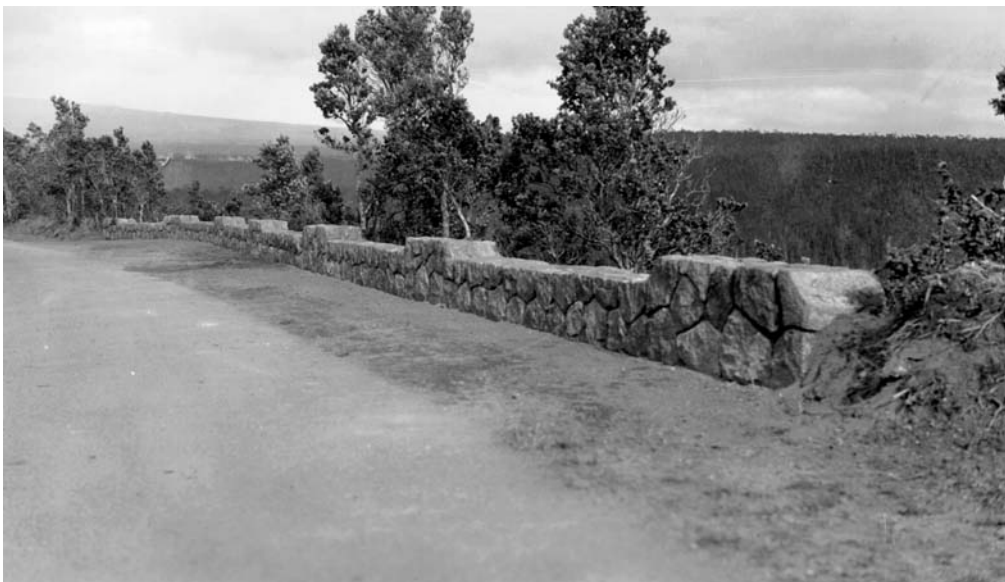
History #6. 1934 photo of the Kilauea Iki parapet guard wall. (HAVO Landscape Architect's Reports 1934)
