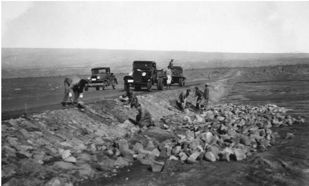
History #10. CCC crews installing mortared stone embankment facing on a section of Crater Rim Road in the Southwest Rift Zone in 1934. (HAVO Landscape Architect's Reports 1934)
