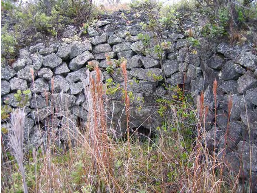
Archeological Sites #2. Several culverts, including this one with a dry-stacked retaining wall above it, remain on the abandoned Uwekahuna-Bird Park Road trace. (PWRO 2005)
