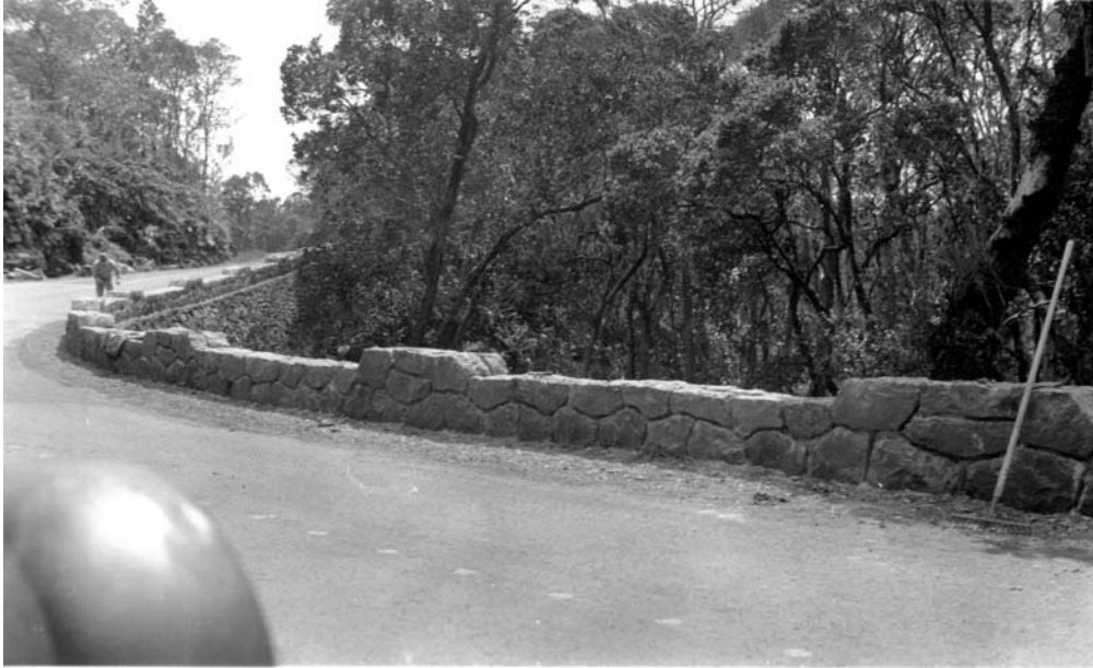
History #7. 1934 photo of the parapet guard wall at Thurston Lava Tube parking lot. The earlier stone retaining wall on which the guard wall was built is visible on the outside of the wall. (HAVO Landscape Architect's Reports 1934)
