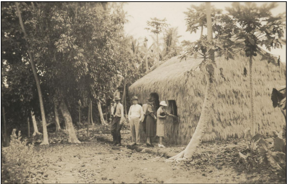
Photo 17. Imge Top, typical structure found in the coastal lowlands of western Puna in Kealakomo. Structure modified in historic period by fishermen to accommodate tin roofing material.
